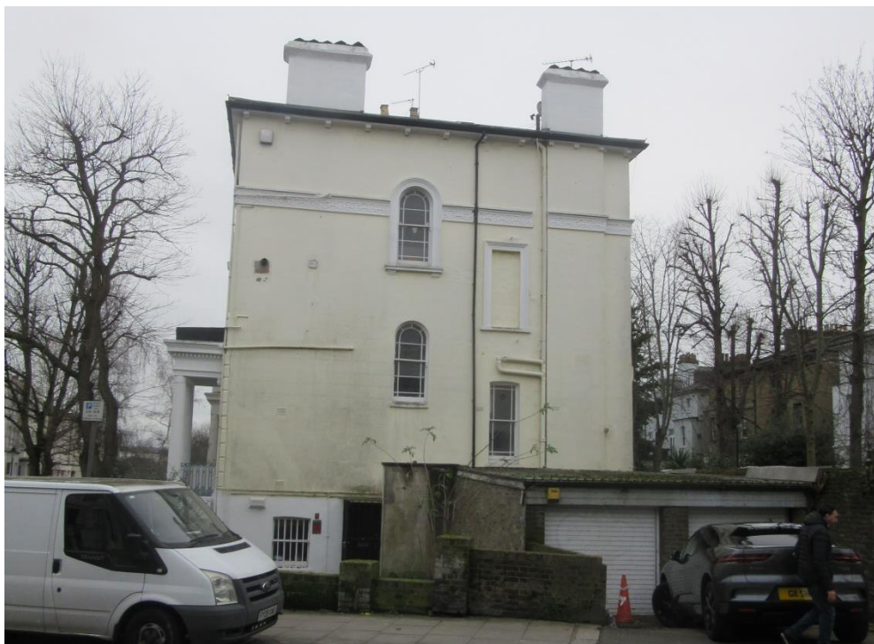
Figure 11: The subject site from Abbey Road, illustrating the unsightly 1960s pair of garages and the plain lower ground floor treatment of the side elevation of No. 39.
