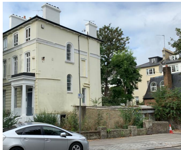
Figure 12: 39 Priory Terrace - Northern elevation
