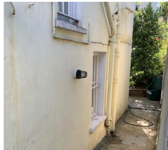
Figure 14: Secondary bedroom window
