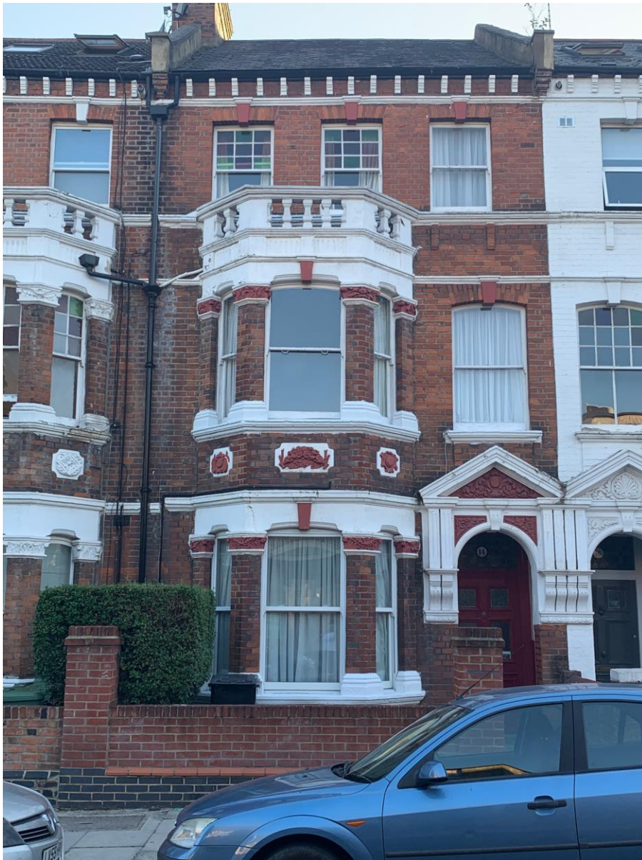
14 Mazenod (adjacent building): UPVC sash on ground floor level
