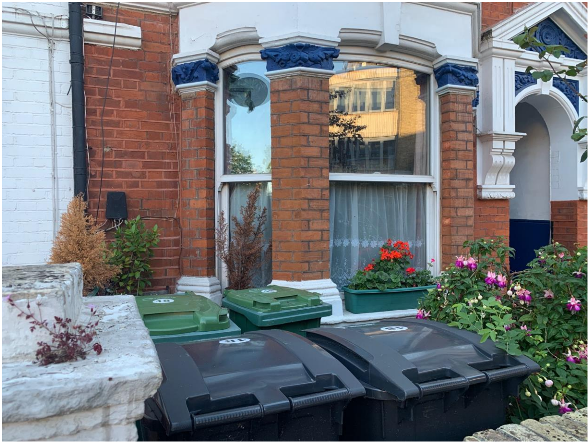
18 Mazenod (adjacent building): UPVC sash on ground floor
