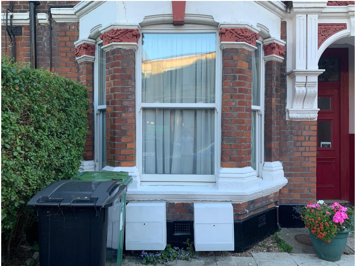
14 Mazenod: ground floor close-up
