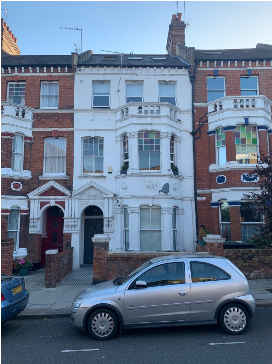
16 Mazenod (my building): UPVC sash on ground floor and UPVC casement on top floor
