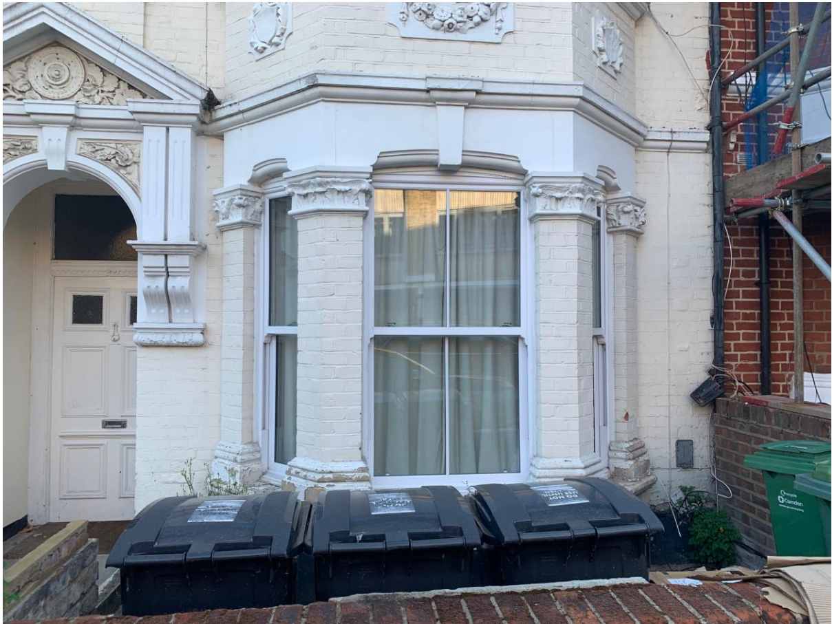
20 Mazenod: ground floor close-up
