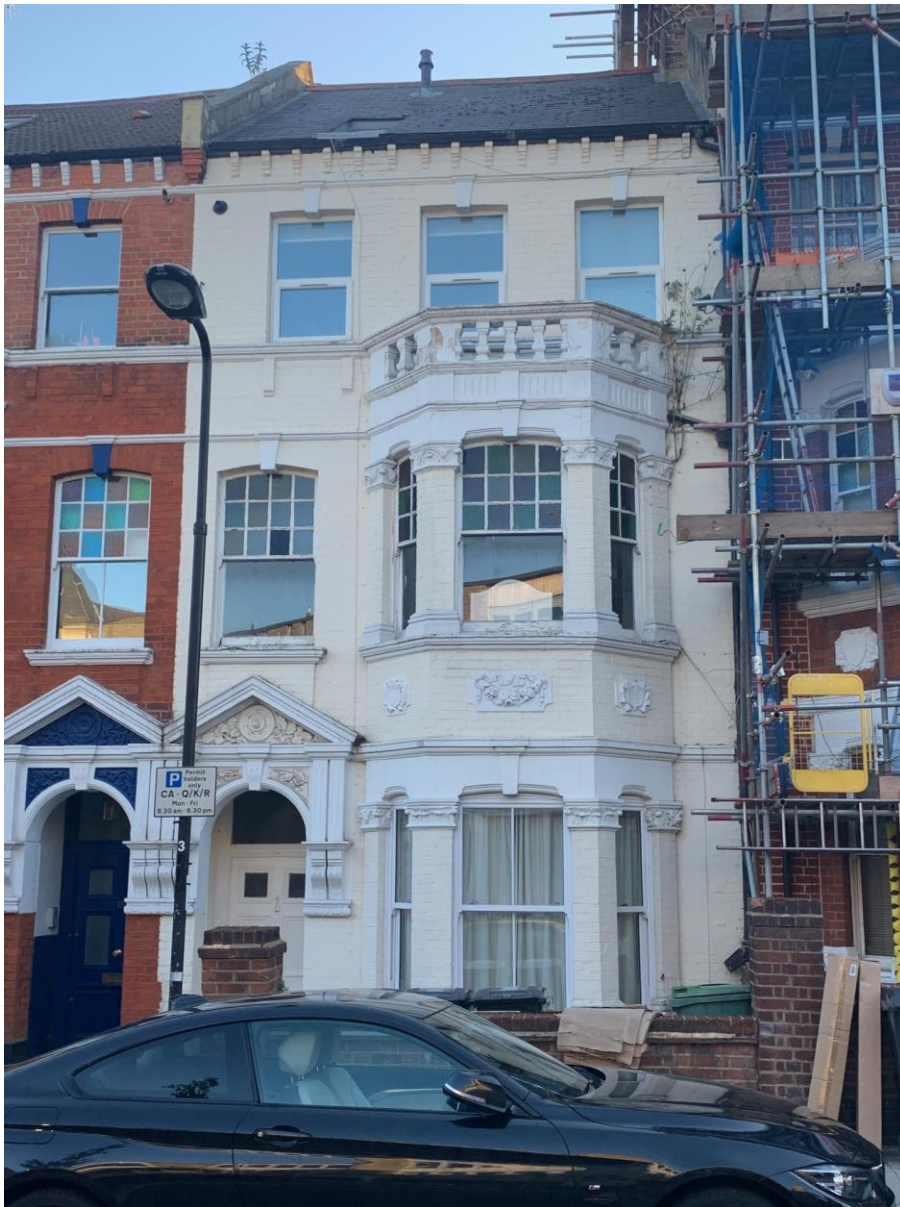
20 Mazenod: UPVC sash on ground floor and UPVC casement window on top floor
