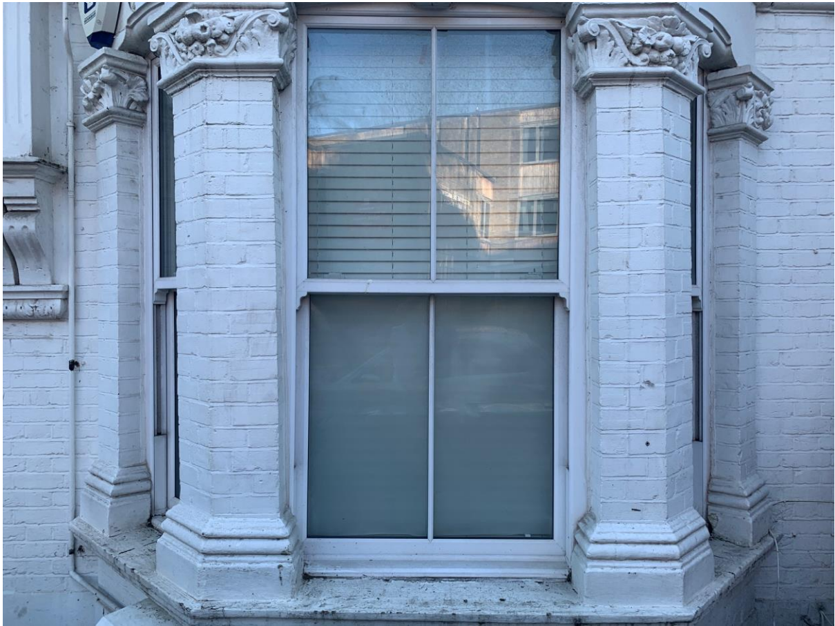
16 Mazenod: ground floor close-up
