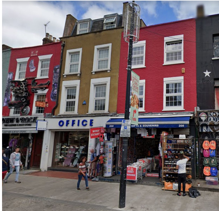
Image 2 - Mansard Extension at 210 Camden High Street
