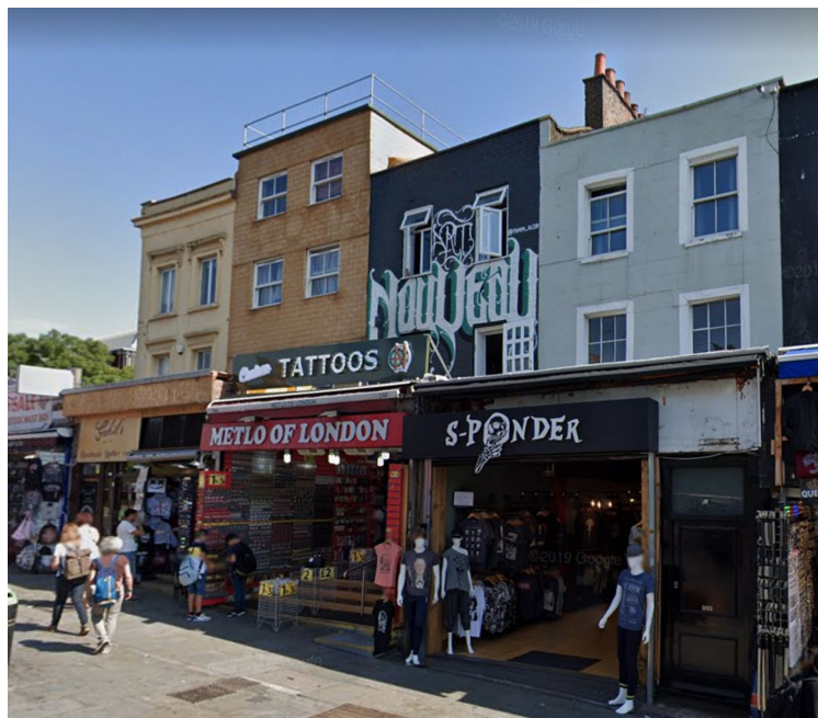
Image 3 - Three storey extension at 246 Camden High Street
