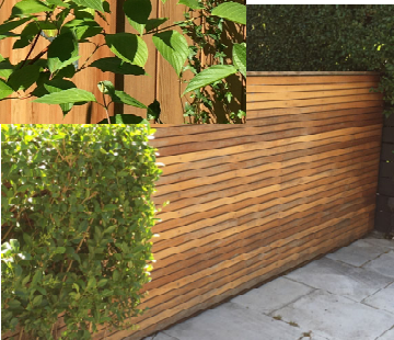
Slatted timber to bin and bike enclosures (larch, cedar or oak)
