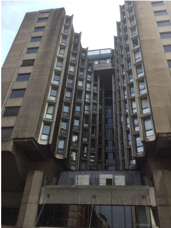
5. View of A/C units looking up towards St. Giles Hotel room windows.
