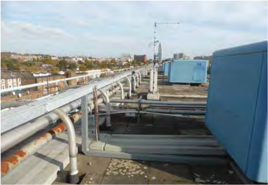
Image 2: Existing heating network on roof of Block A
