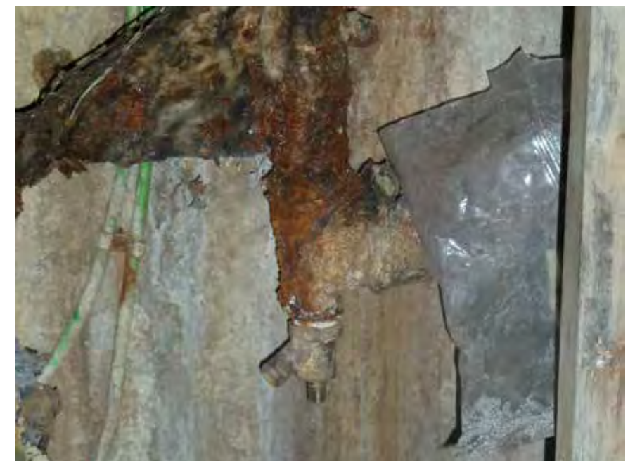
Corroded valve found on site
