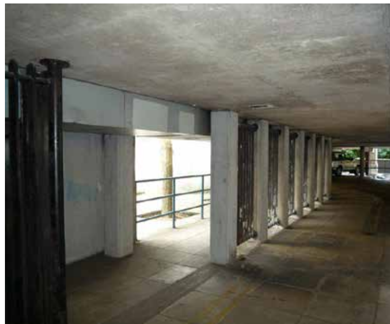
Image 1: Existing pipes fixed to soffit within substantial casing. Allows circa 1800mm clearance to underside
