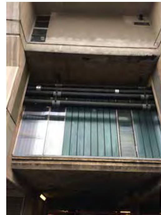
Profiled glazing & black mechanical pipes
