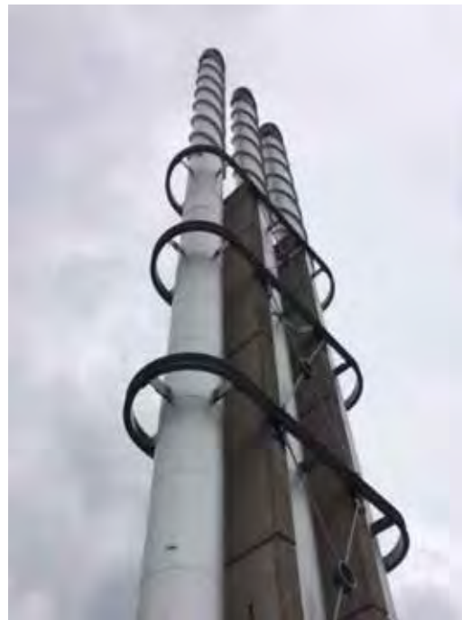
Metal casing to chimney flue
