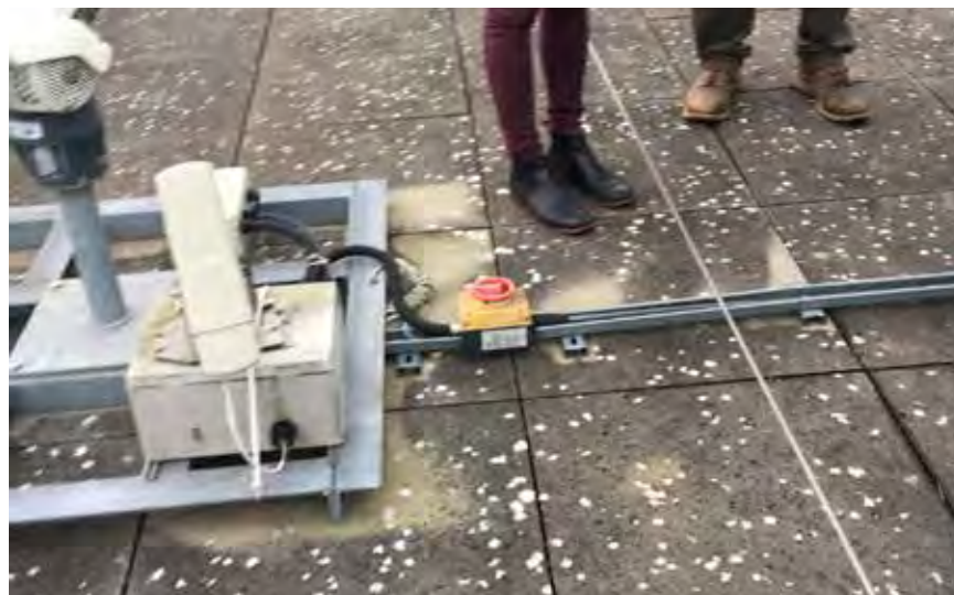
Typical bracing currently used elsewhere on Block B roof
