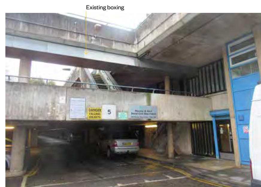
Existing condition of boxed section fixed to walkway soffit
