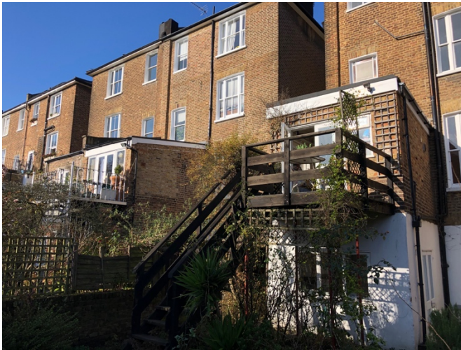
existing timber balcony and stair | we propose to replace this unsightly and dilapidated balcony and stair, with a lightweight steel balcony, painted in a dark colour
