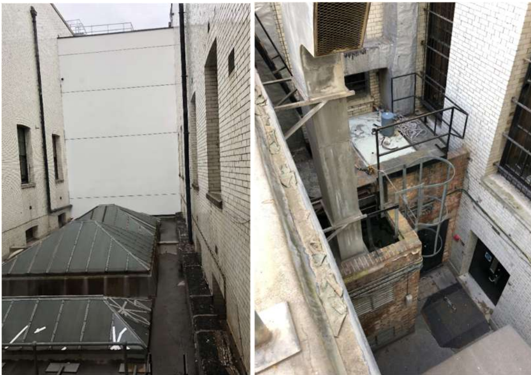
Figure 1 VIEW OF COURTYARD TOWARDS CRAWFORD STAIR & EXISTING DUCTS IN COURTYARD
