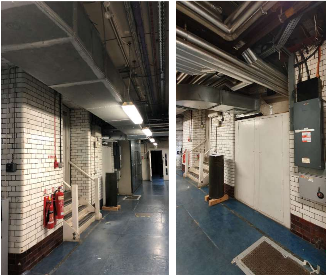
Figure 4 LEVEL 01 EAST CORRIDOR & EXISTING BLOCKEDUP WINDOW FOR SERVICE ROUTE
