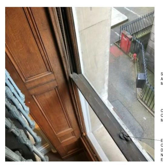
SASH BOXES TO BE CHECKED FOR ROT — AND REPAIRED, CLEANED TO ALLOW FREE MOVEMENT.
