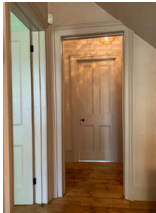
existing view 2 showing landing/lobby with original doors to study & office
