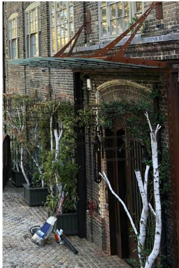
Front door at 10A Belmont Street
