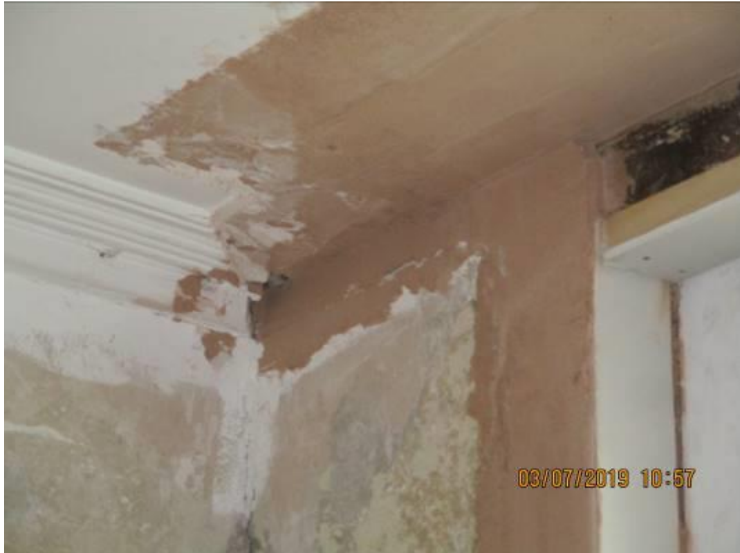
Photo No. 9 – Missing Moulded Cornice and Picture Rail
