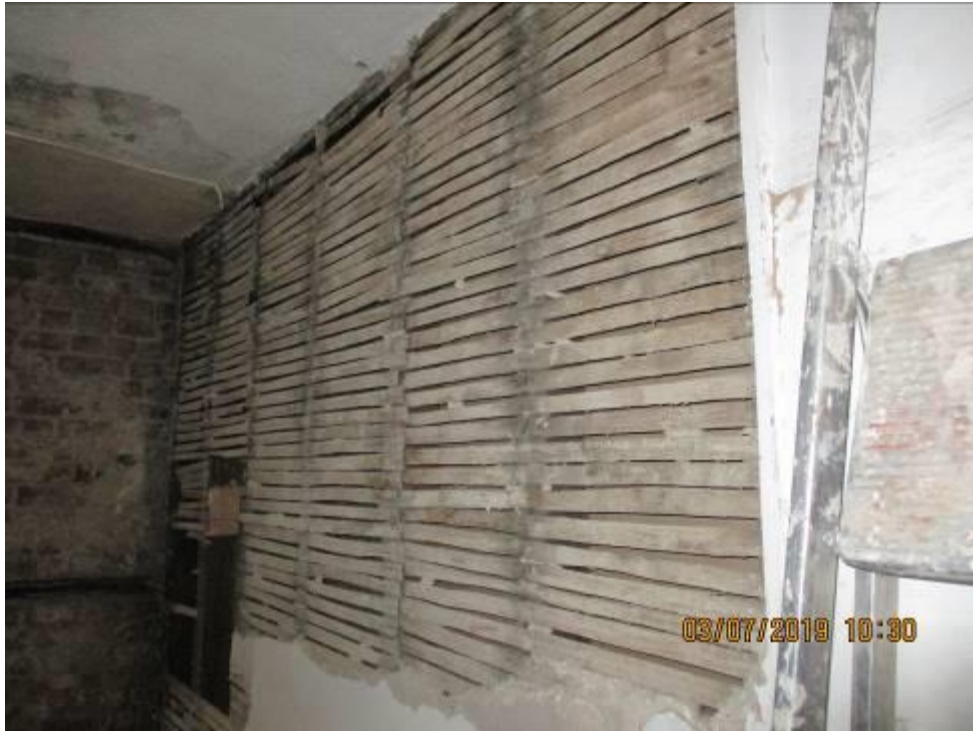
Photo No. 5 – Missing Internal Wall Plaster
