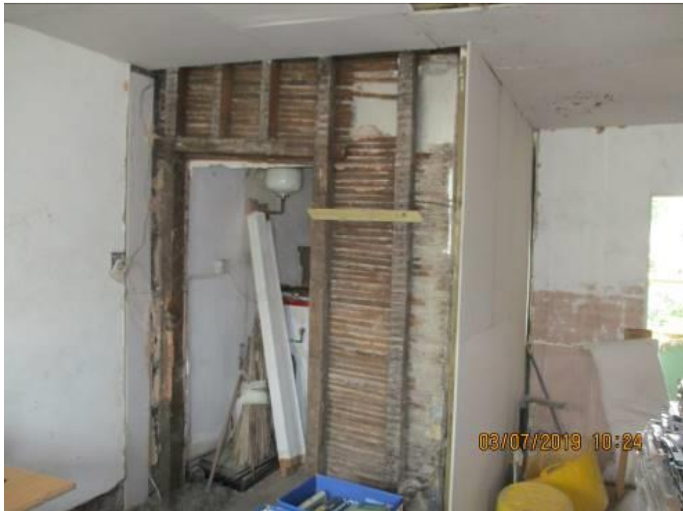
Photo No. 4 – Missing Internal Wall Plaster
