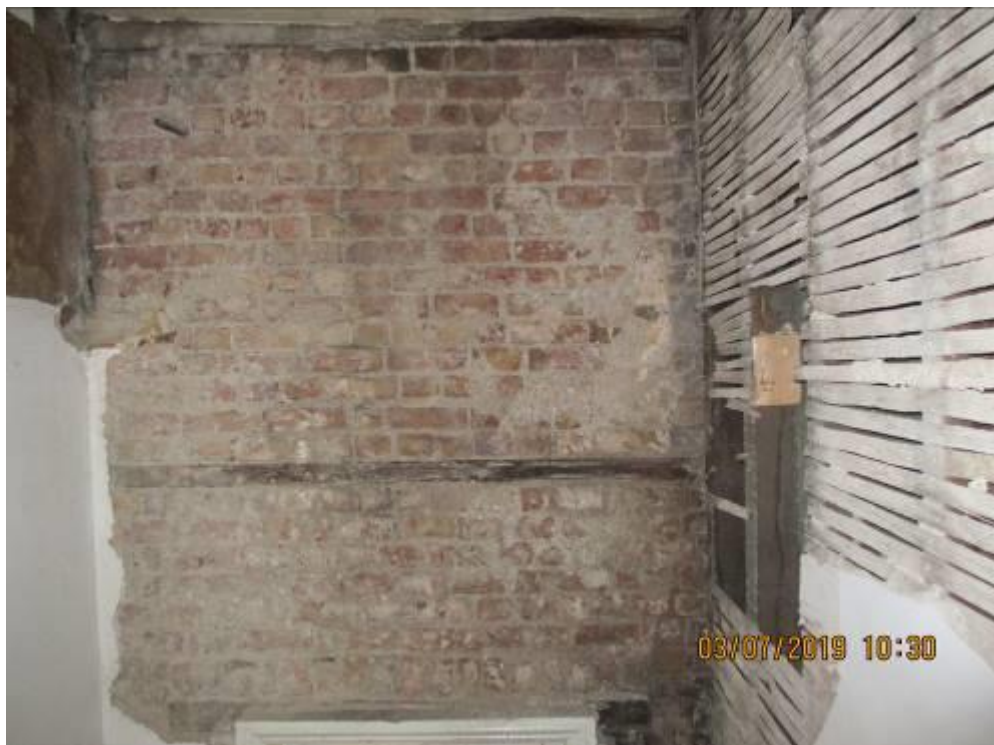
Photo No. 6 – Missing Internal and External Wall Plaster
