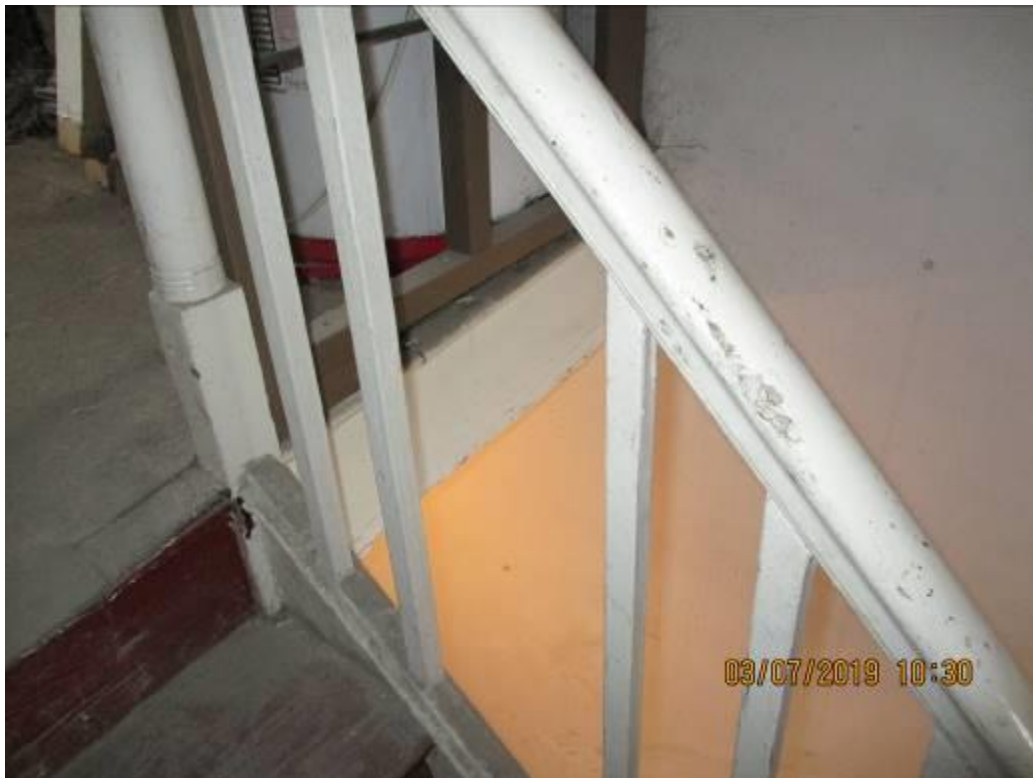
Photo No. 7 – Missing Timber Balusters
