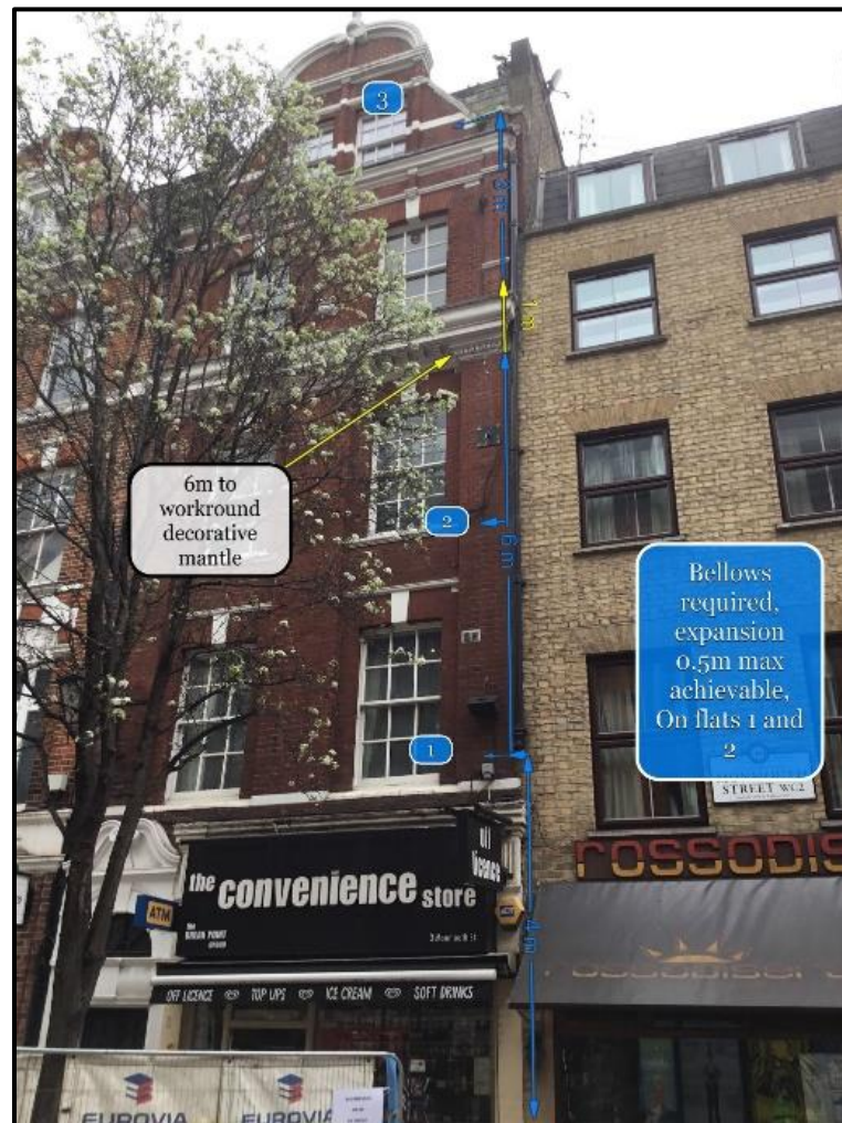
Plate 2 – Route of the proposed external riser to the west frontage
