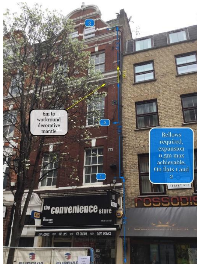
Plate 2: An indicative drawing of the proposed vertical gas riser and lateral gas pipes to the west facing (front) elevation of 3 Monmouth Street.
