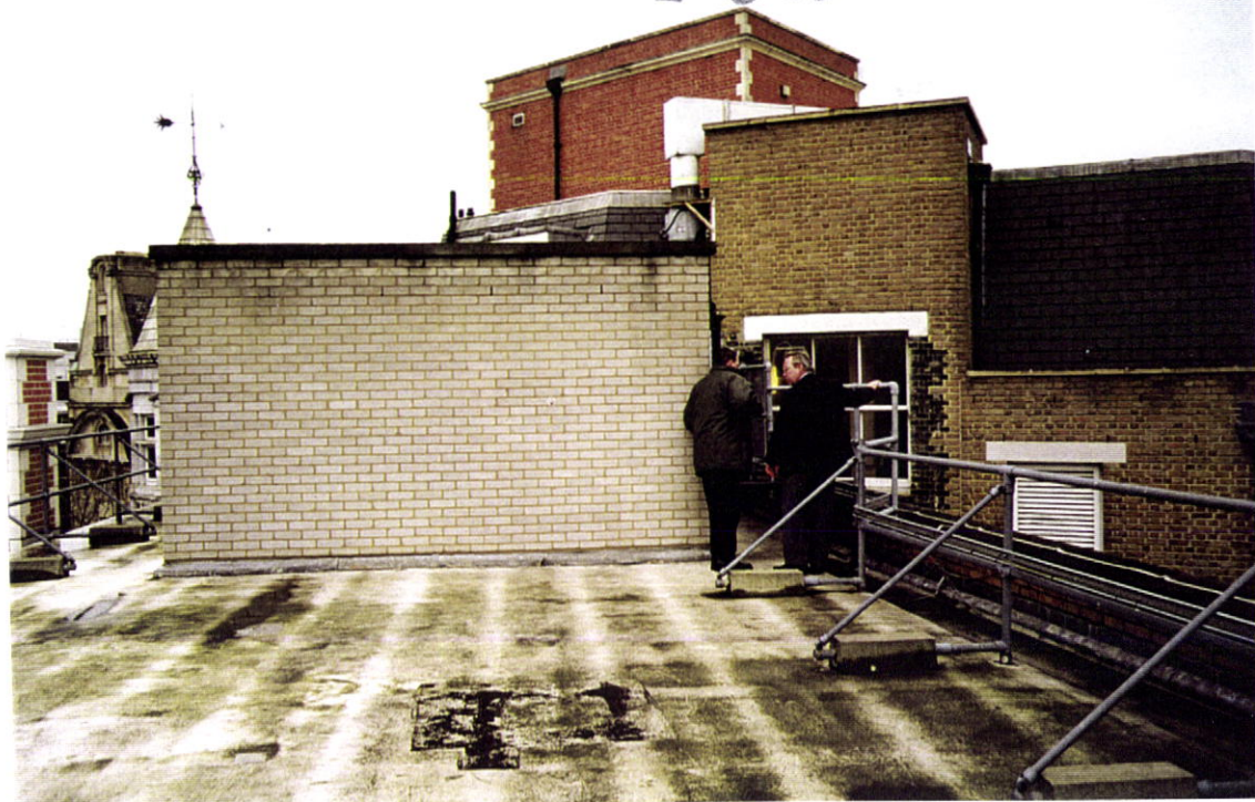
Roof level showing lift motor room housing and existing AC unit behind
