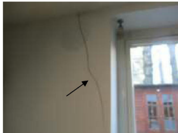
Cracking to rear wall in kitchen
