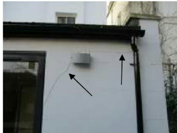
Cracking to rear wall
