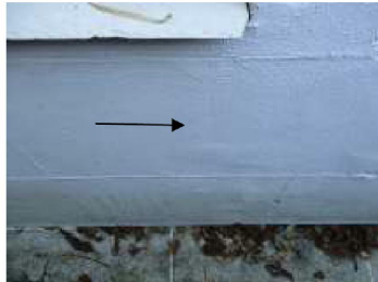
Cracking below flank window
