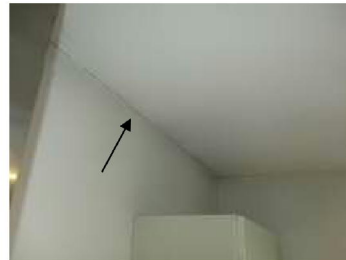
Cracking along flank wall in kitchen
