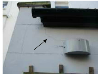
Cracking to rear wall
