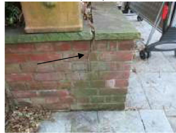
View of unrelated damage to garden wall
