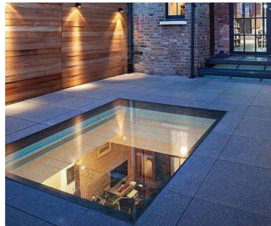
Example of a walk on rooflight to a basement
