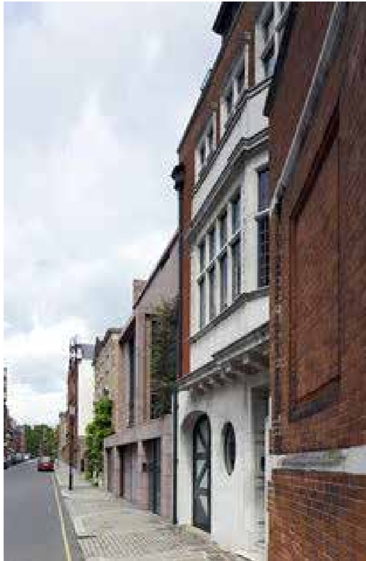
The Red House - Tony Fretton Red Limestone in a Conservation Area
