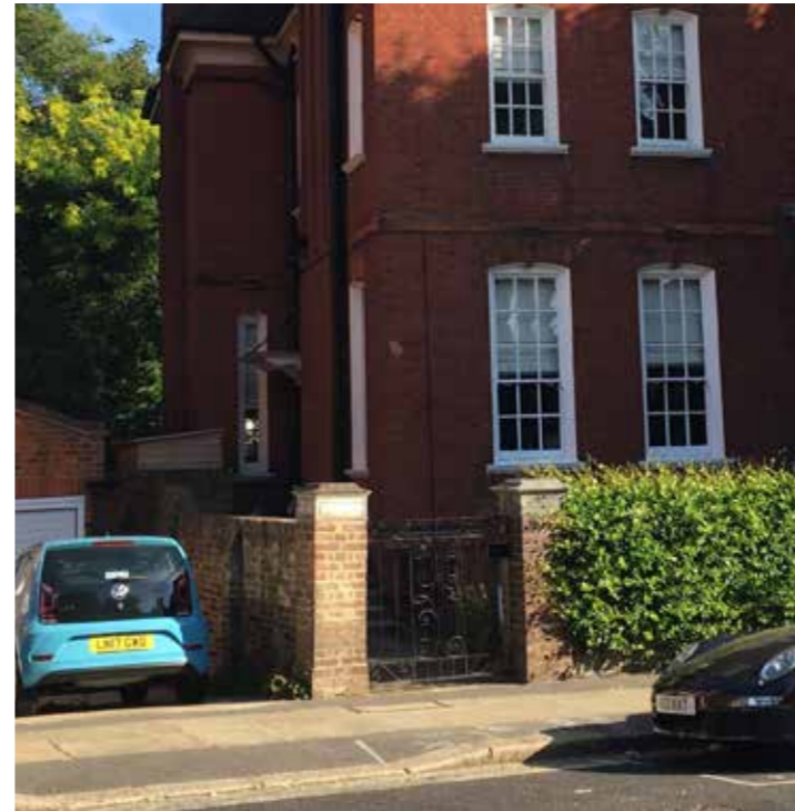
Typical entrance gate (no.7 / no.9)
