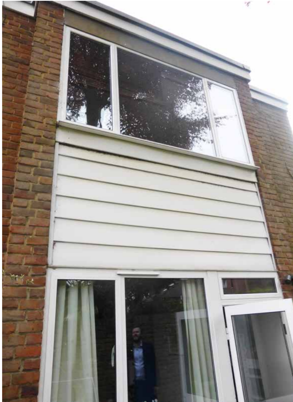
Rear elevation of existing building. Living room window at 1st floor.
