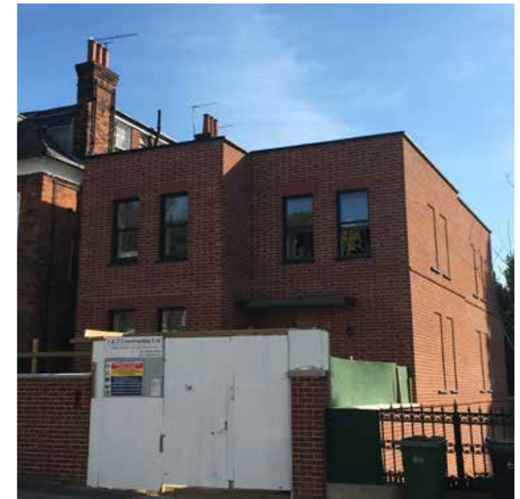
Recent redevelopment - 23a Hampstead Hill Gardens
