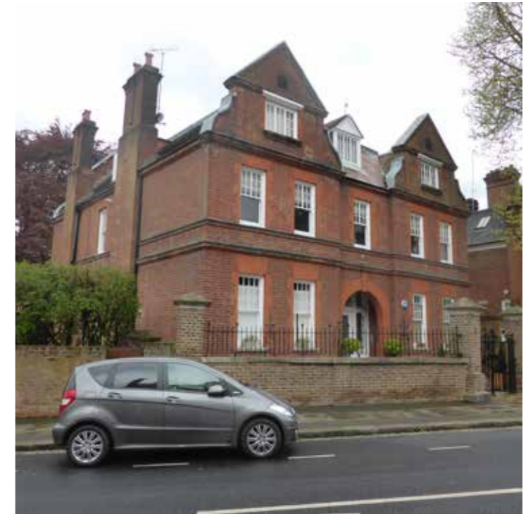
Typically boundary wall and railings (no.4)
