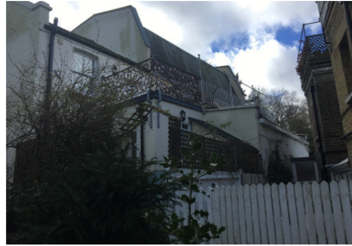
view 7 Rear elevation of Ambridge Cottage and Sandy House looking west.
