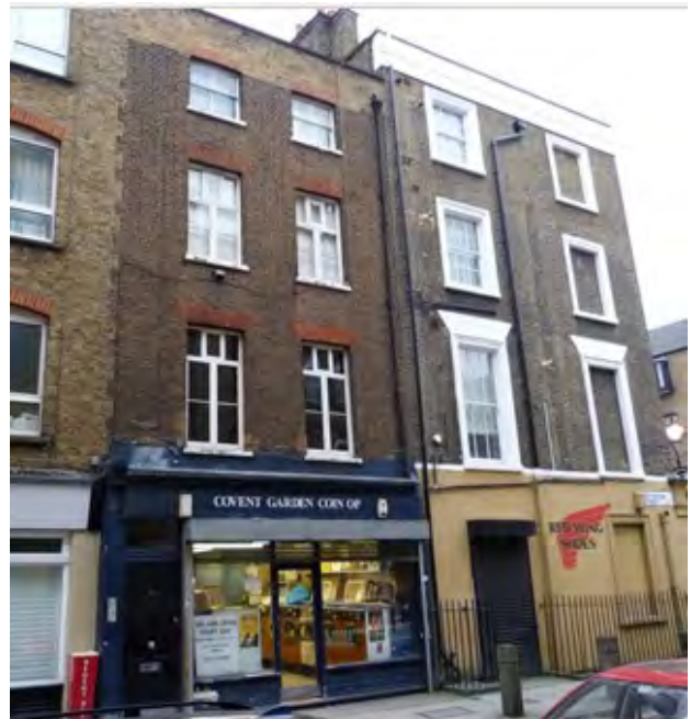
Figure 7: No.33 Betterton Street, Grade II listed
