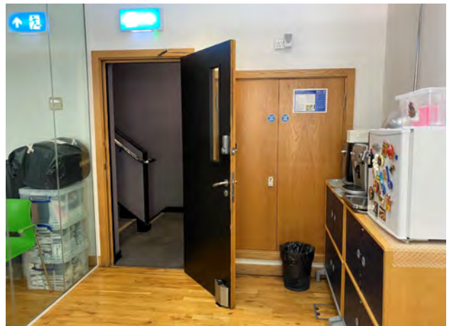
Figure 28: 1980s staircase lobby
