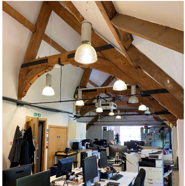
Figure 27: Exposed roof structure
