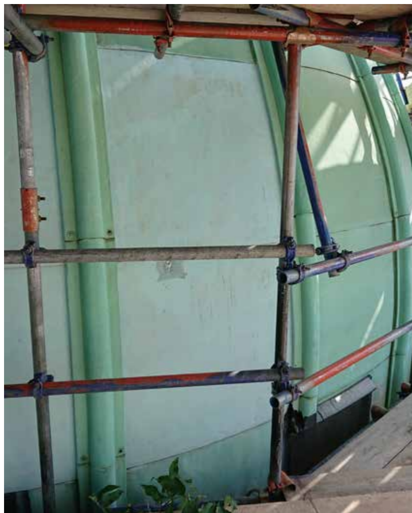
Figure 29: Exterior view of copper cladding on dome roof (2019) © H&R
