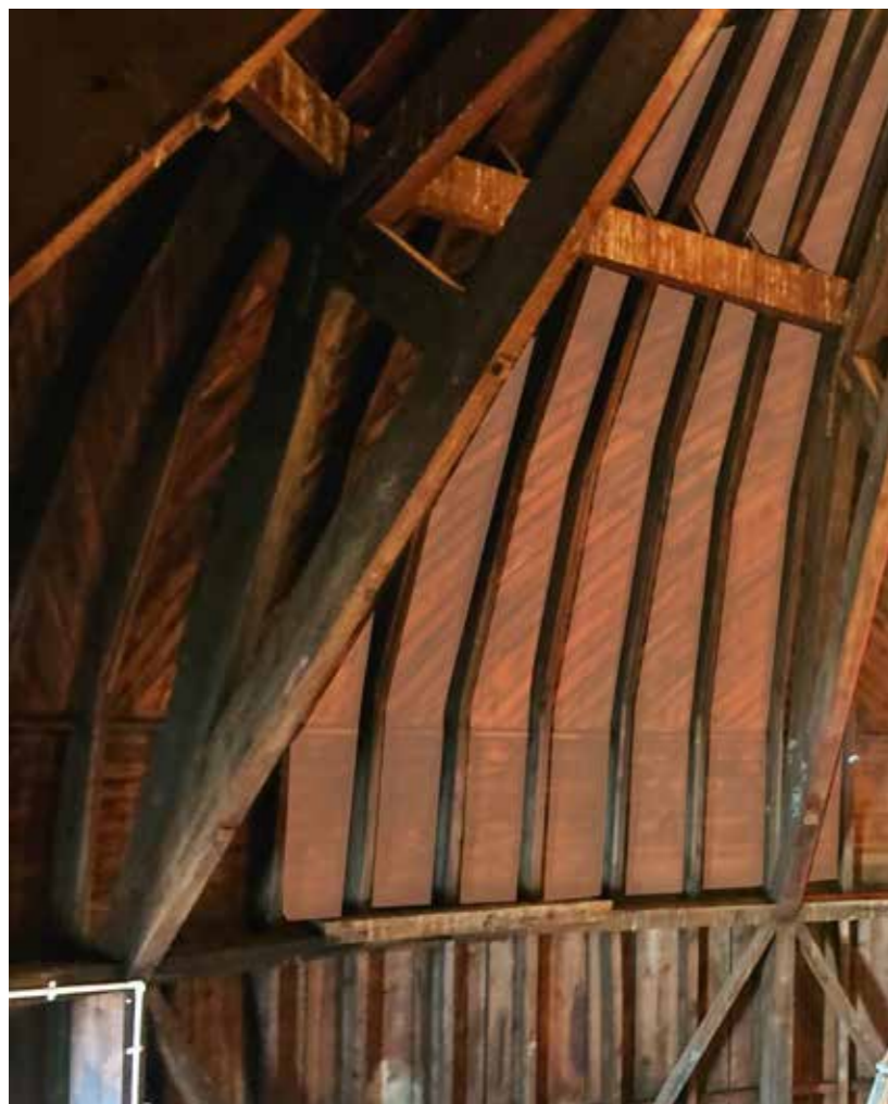
Figure 32: Interior view of dome and indication of the roof boarding (2019) © H&R
