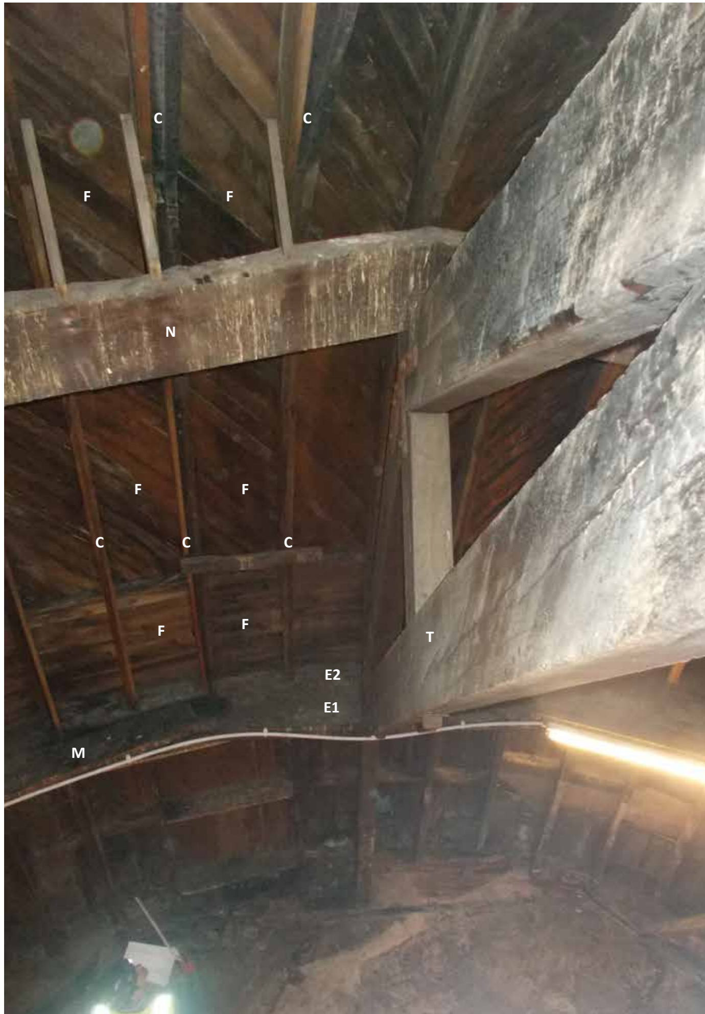
Figure 14: View facing down from apex, showing timber framework construction (2019) © H&R
