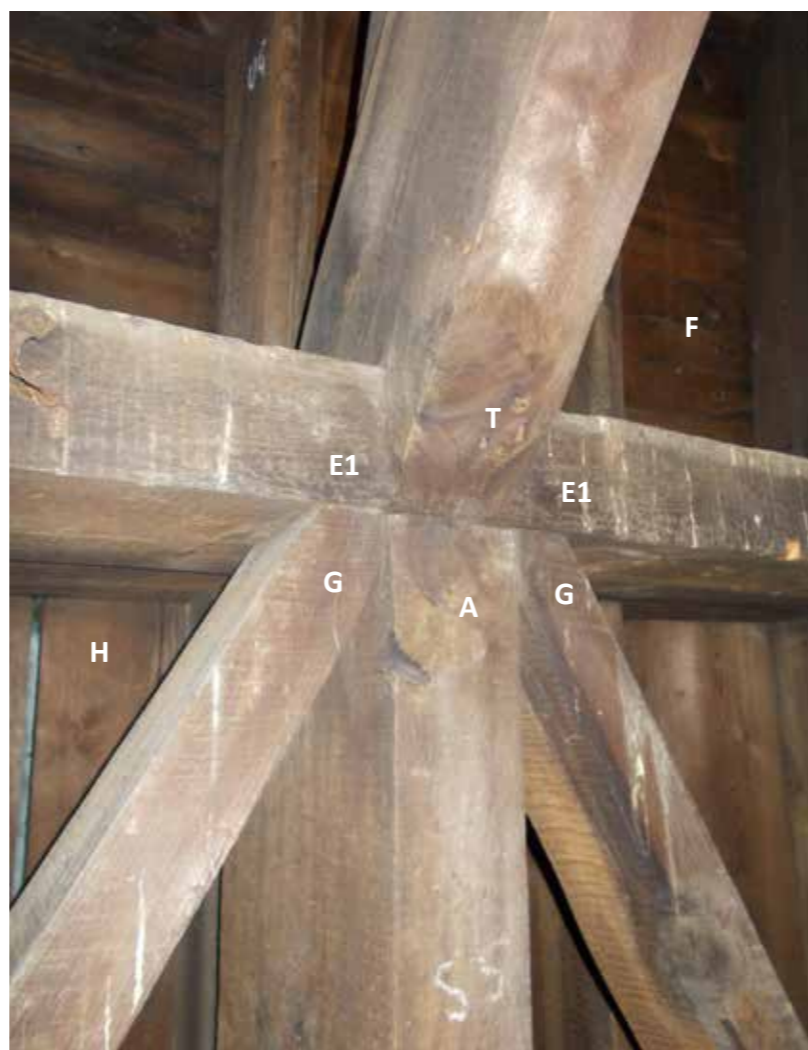
Figure 7: Birds-mouth joinery detail between outer rafter plate and end of truss. Junction point for main support post with braces and outer rafter plate (2019) © H&R
