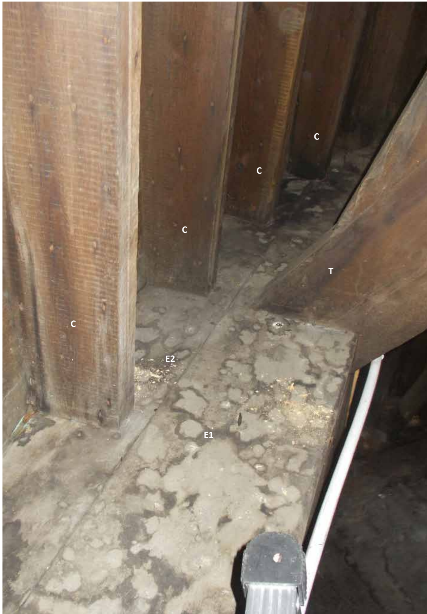
Figure 20: Top face view of upper rafter plate (2019) © H&R
