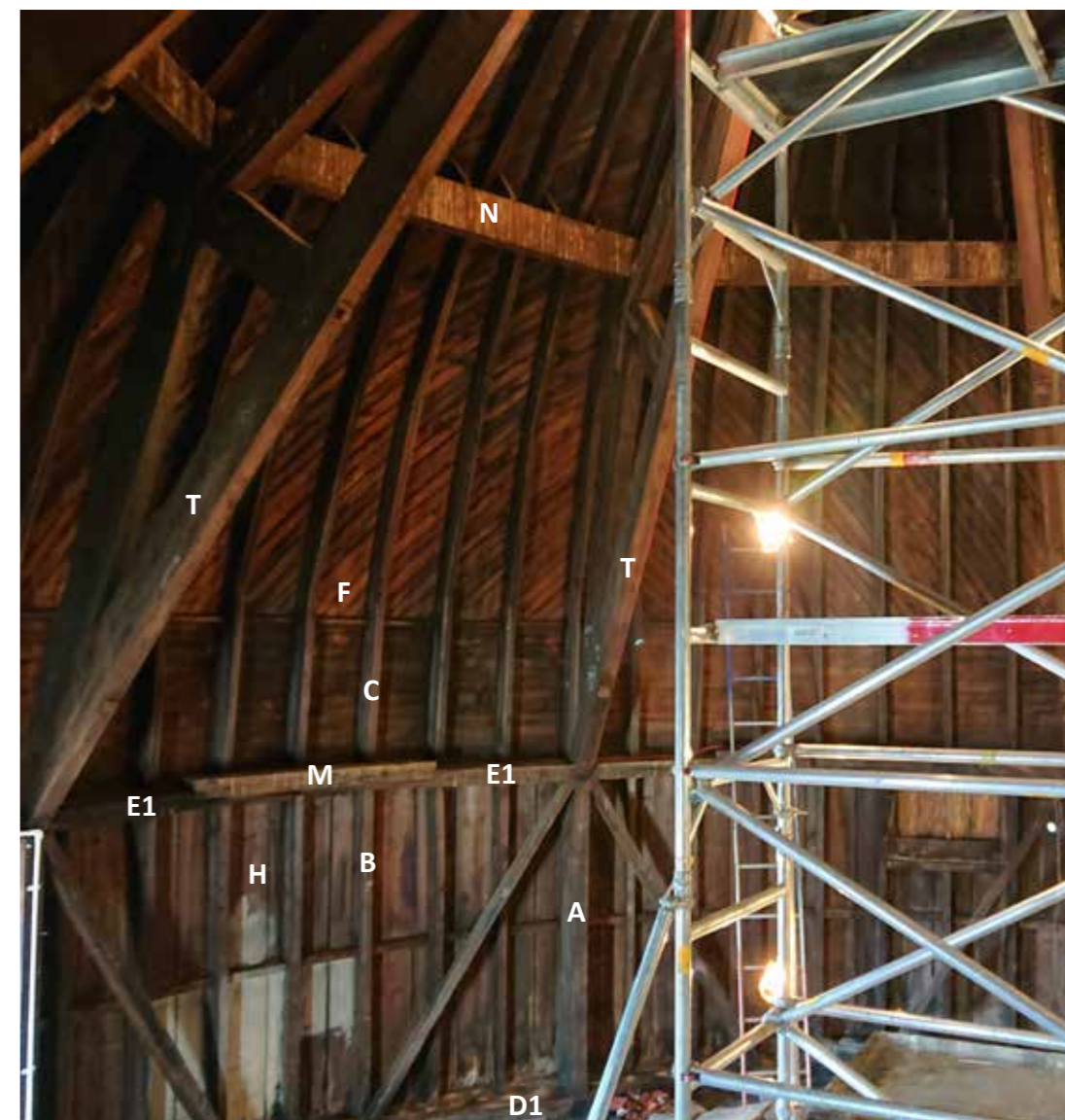
Figure 8: Inside of the dome, showing timber framework construction (2019) © H&R
