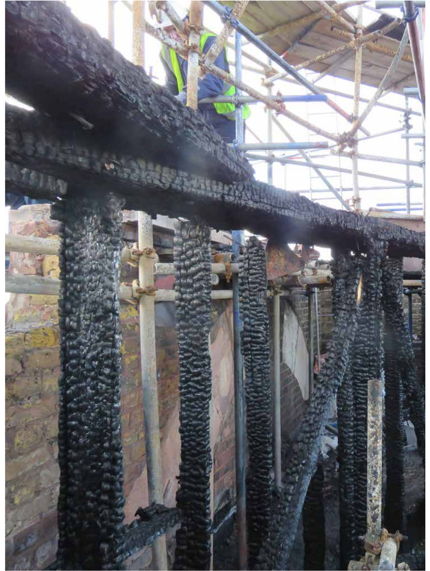
Figure 147: Horizontal rafter wall ties (M) with upper rafter plate (E) and wall studs (B) in situ (2020) © SLHA
