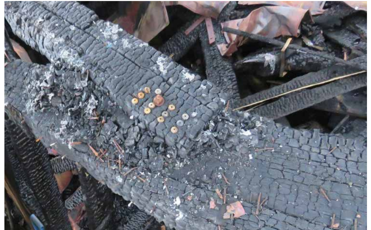
Figure 143: Horizontal rafter wall ties (M) with upper rafter plate (E) in situ. Note evidence of modern strengthening inserts used to connect them to the upper rafter plates. (2020) © SLHA
