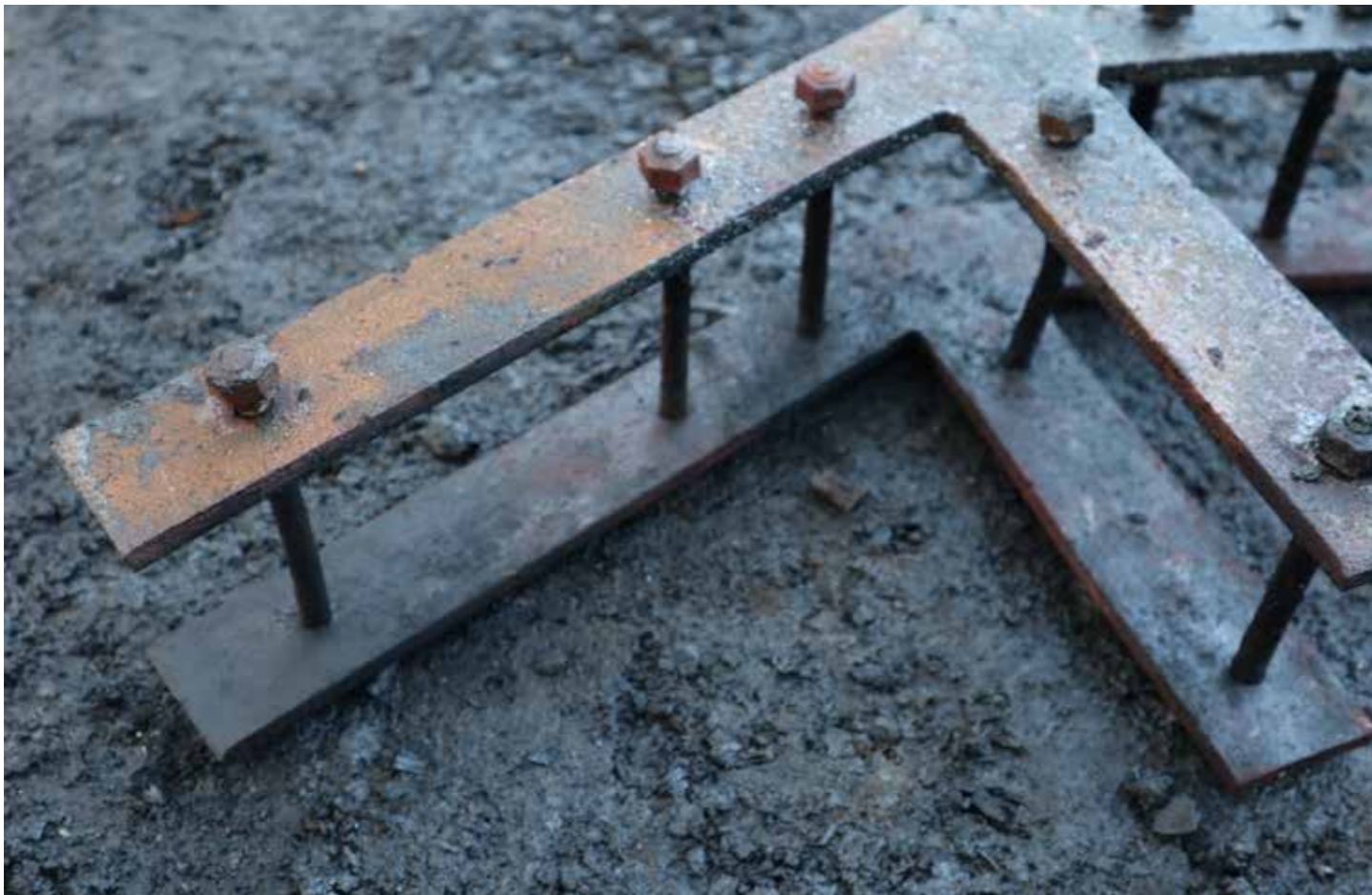
Figure 157: Sample #23 - Bolted arrowhead metal brace (T4) (2020) © SLHA
