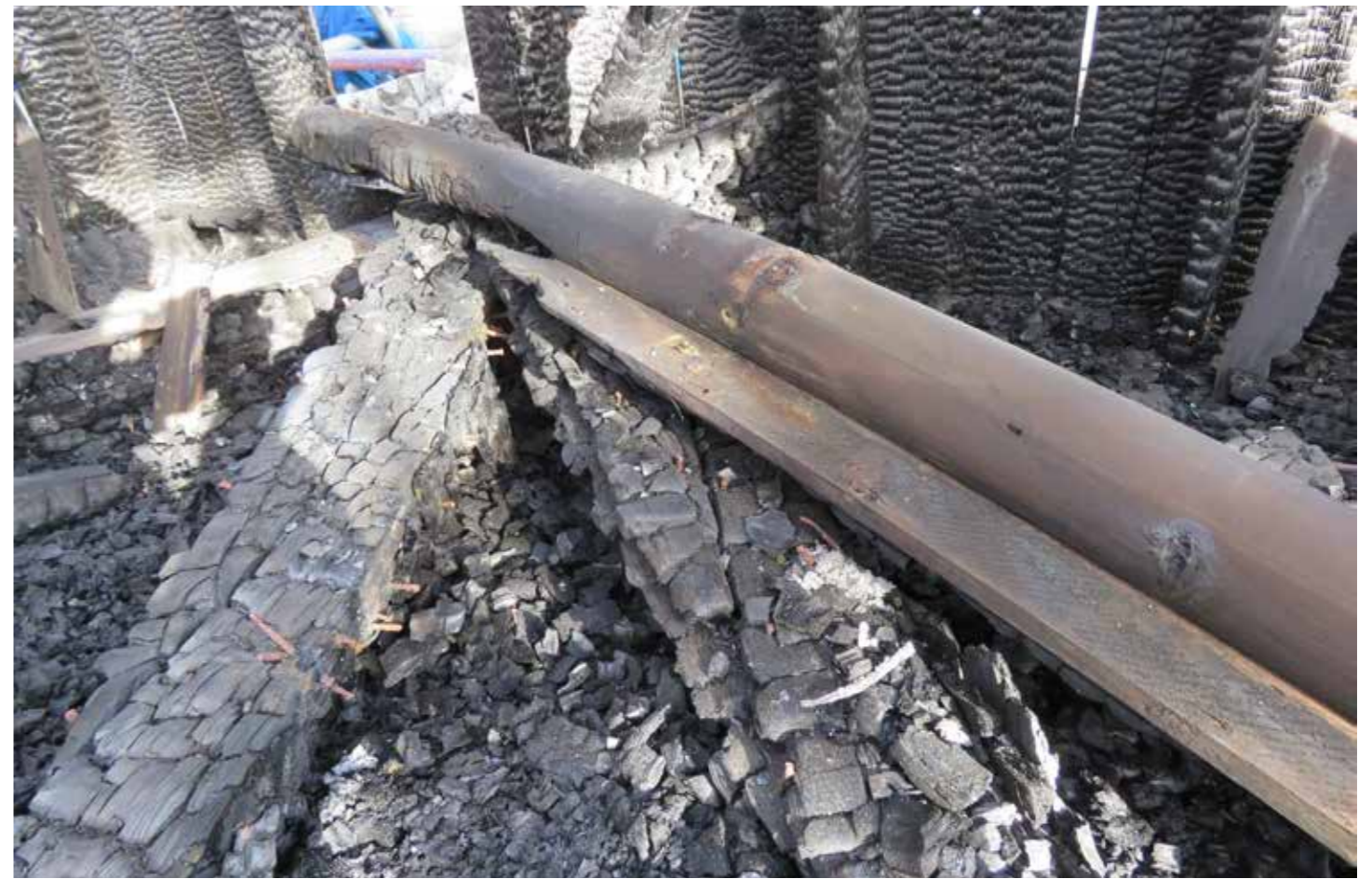
Figure 133: Timber roof rolls (L) in situ (2020) © SLHA
