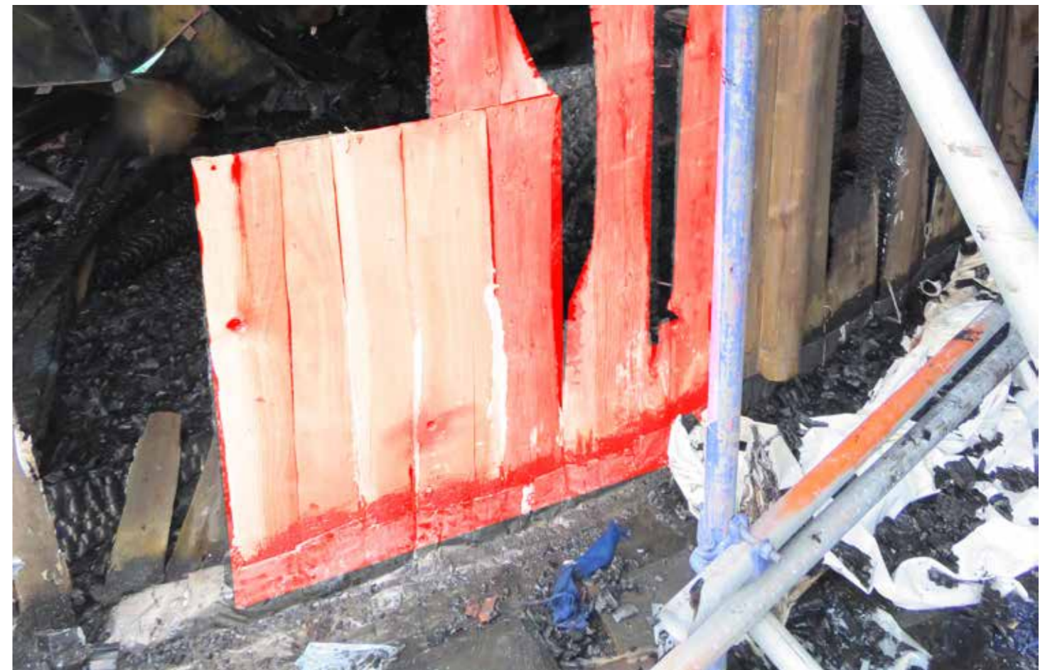
Figure 108: Wall boarding (H) in situ (exterior view) (2020) © SLHA
