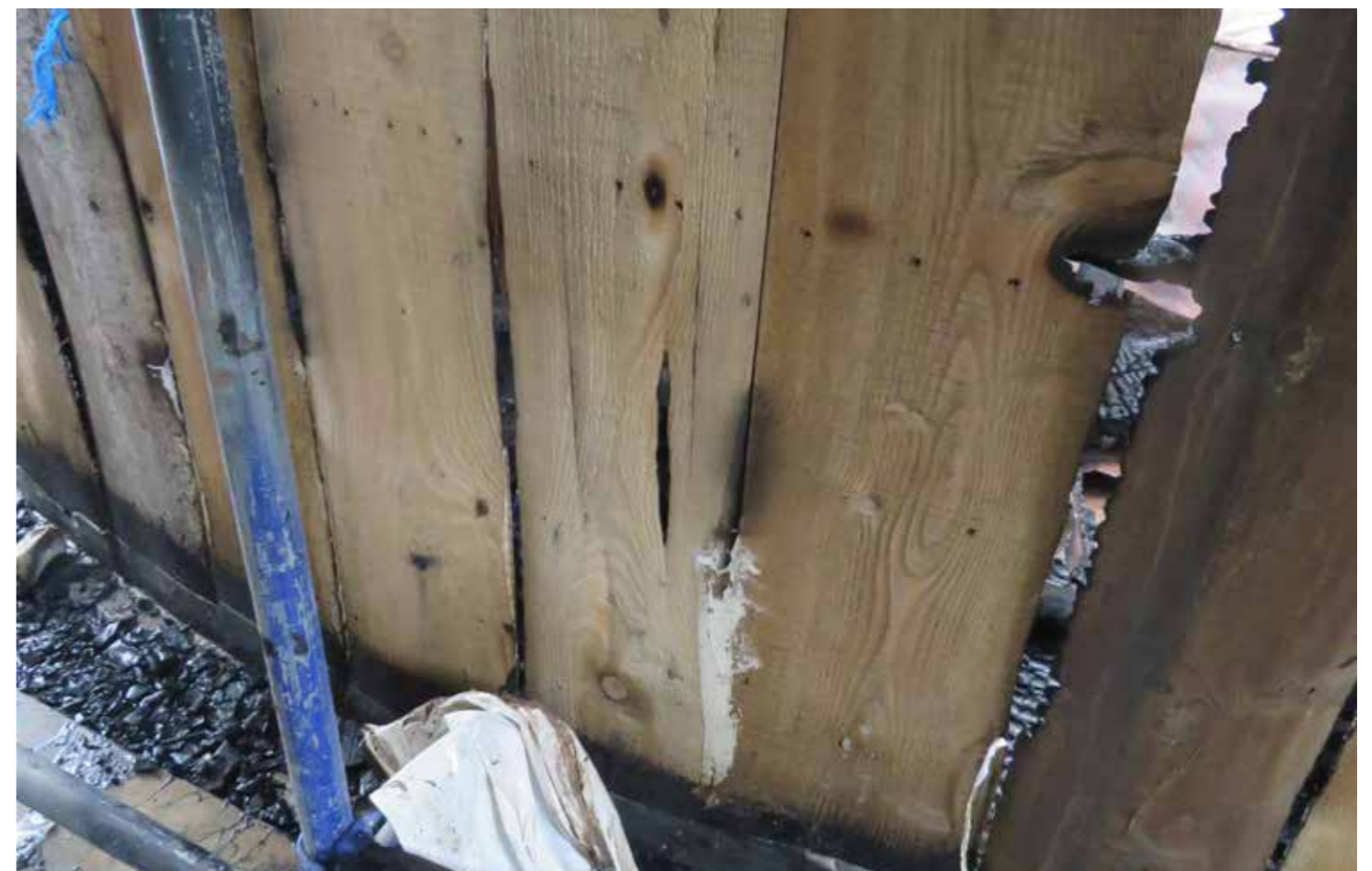
Figure 111: Wall boarding (H) in situ (exterior view) (2020) © SLHA
