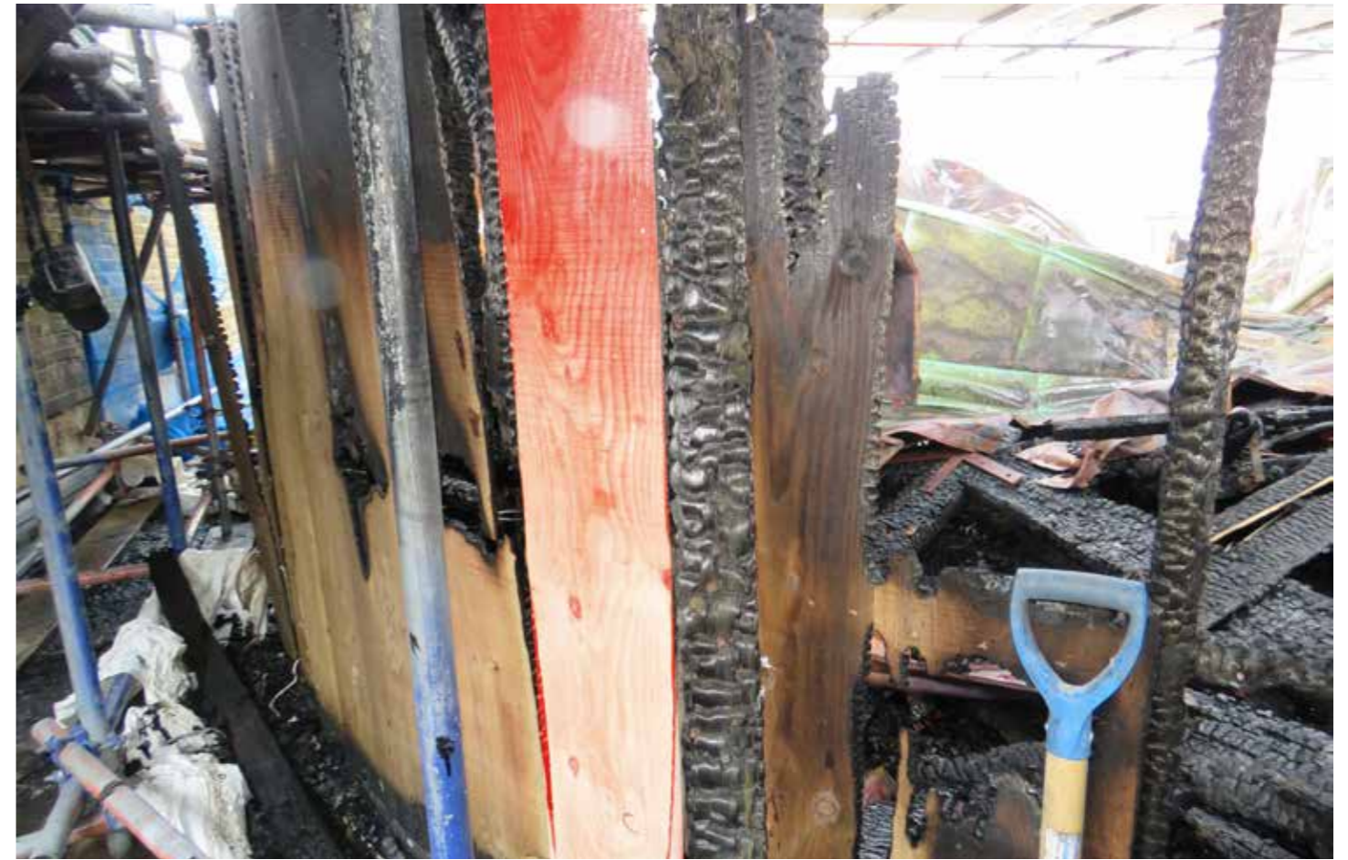
Figure 107: Wall boarding (H) in situ (exterior view) (2020) © SLHA
