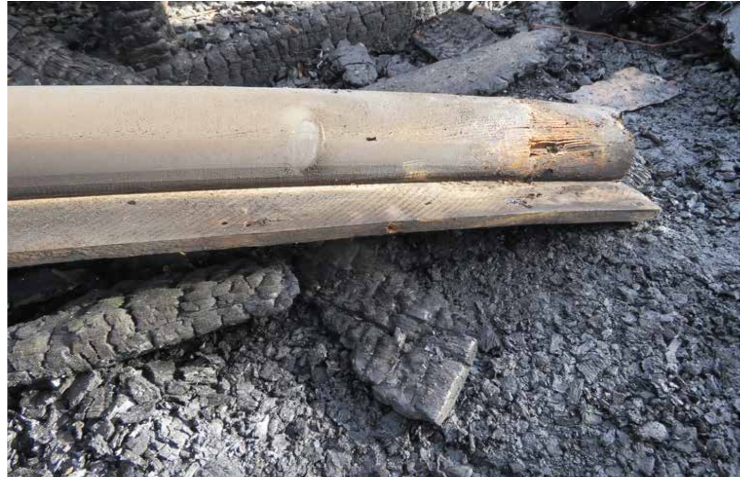
Figure 129: Timber roof rolls (L) in situ (2020) © SLHA
