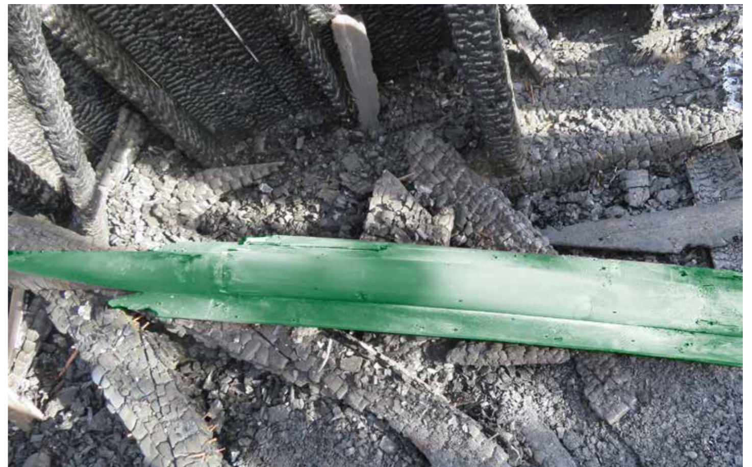
Figure 127: Timber roof rolls (L) in situ (2020) © SLHA
