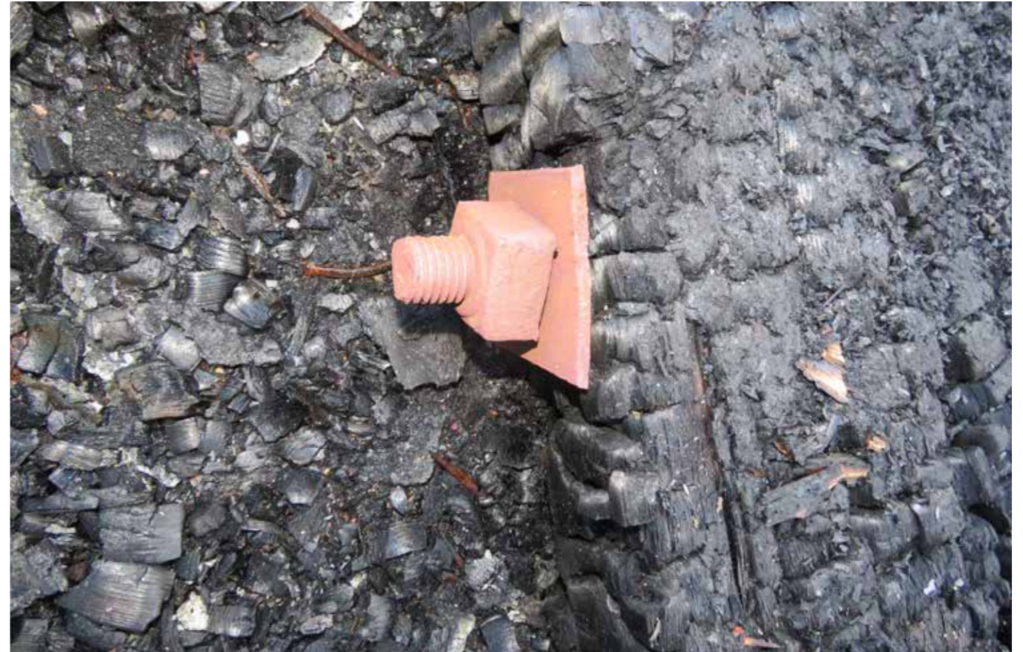
Figure 155: Bolted metal brace (T4) in situ (2020) © SLHA
