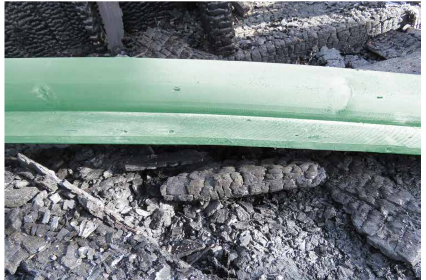
Figure 126: Timber roof rolls (L) in situ (2020) © SLHA
