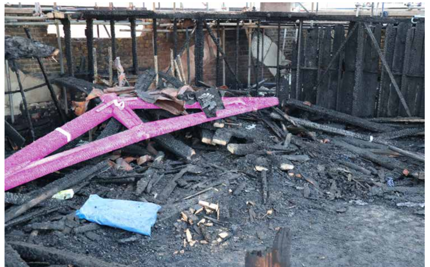
Figure 153: Trusses (T) found in debris (2020) © SLHA
