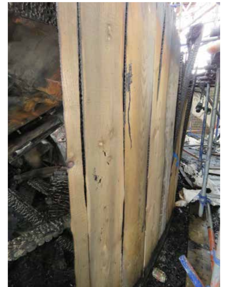
Figure 115: Wall boarding (H) in situ (exterior view) (2020) © SLHA
