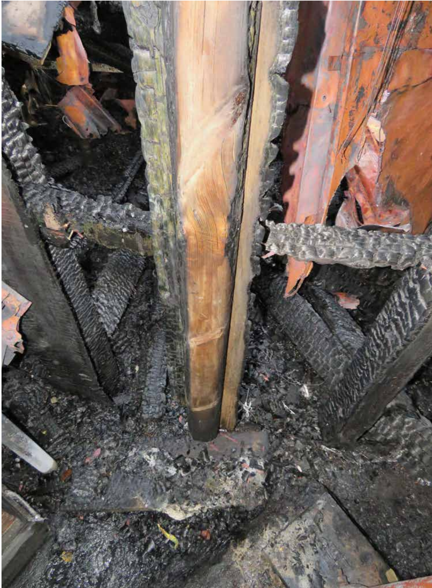
Figure 128: Timber roof rolls (L) at base level in situ (2020) © SLHA
