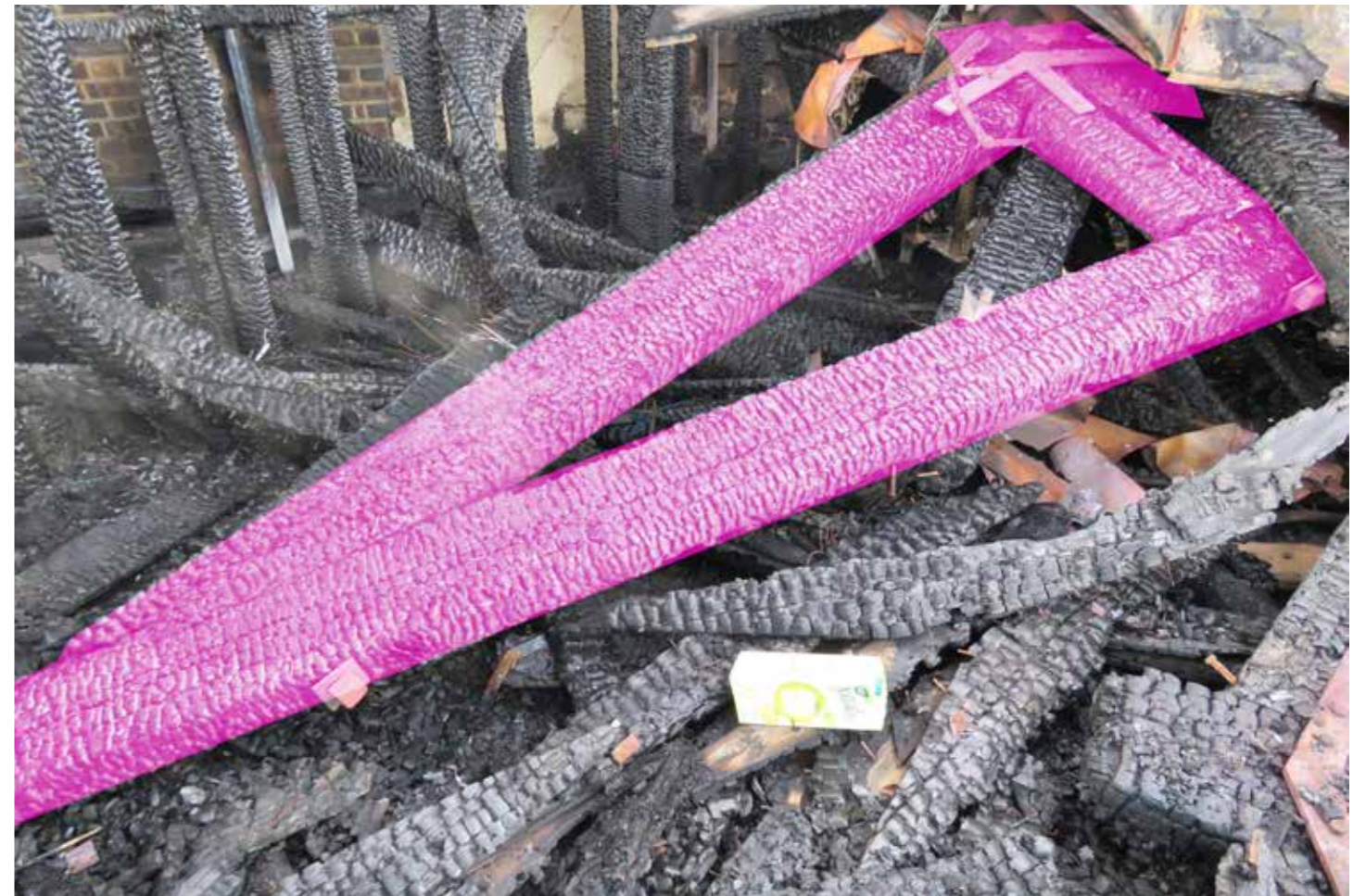
Figure 152: Trusses (T) found in debris (2020) © SLHA
