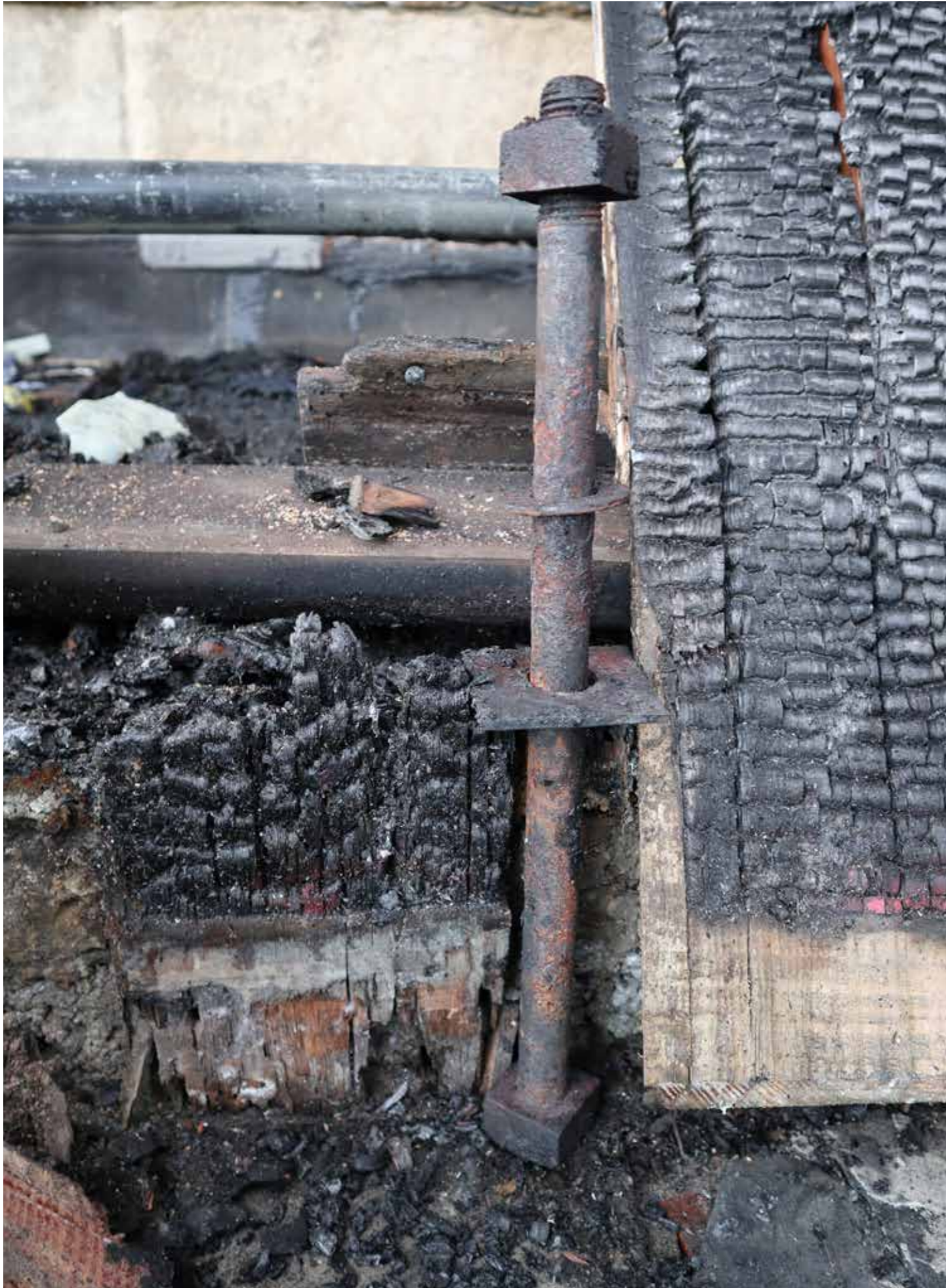
Figure 154: Sample #22 - Bolted metal brace (T4) (2020) © SLHA
