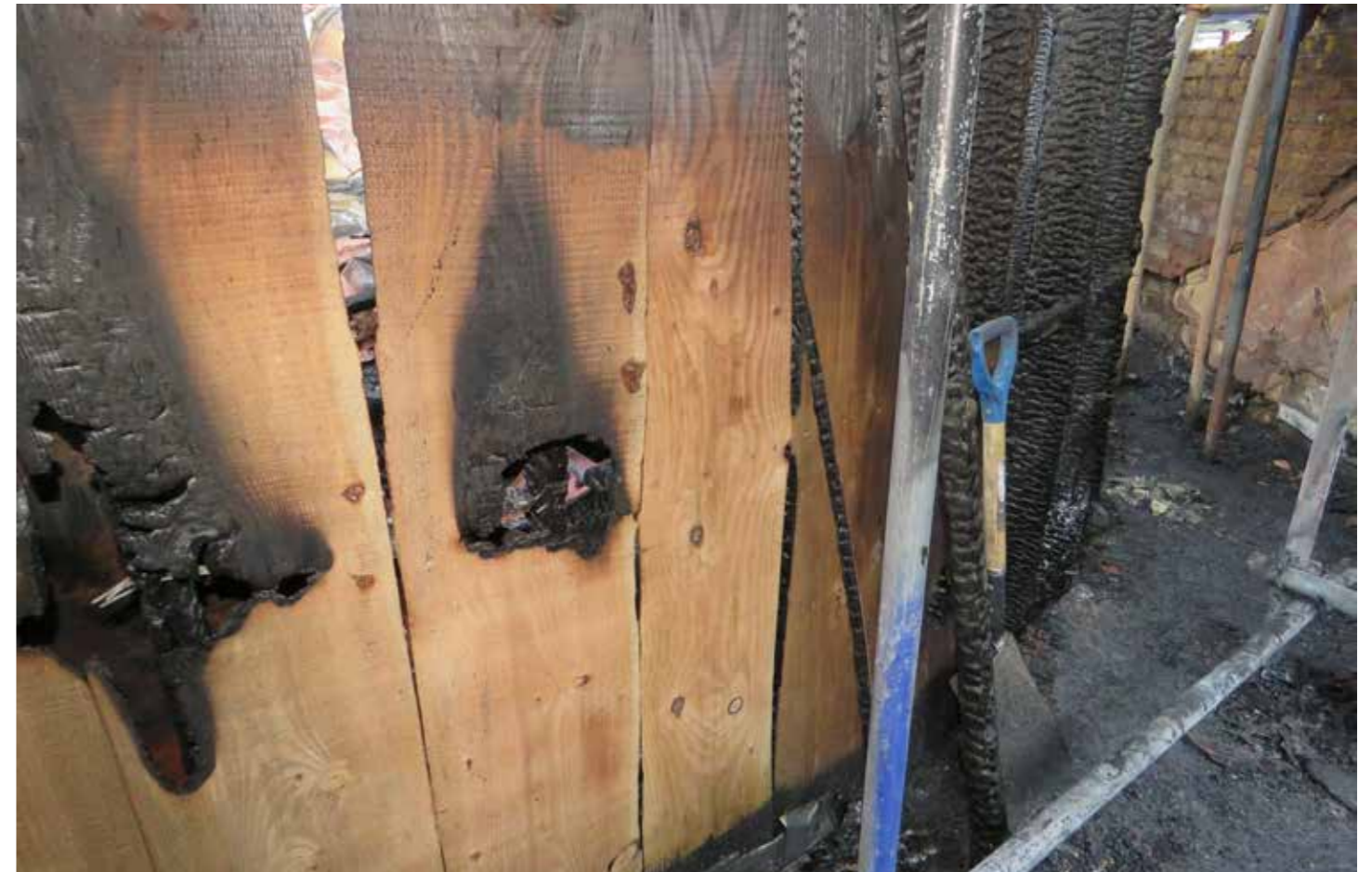
Figure 110: Wall boarding (H) in situ (exterior view) (2020) © SLHA
