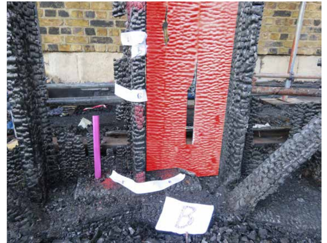
Figure 104: Wall boarding (H) in situ (interior view) (2020) © SLHA
