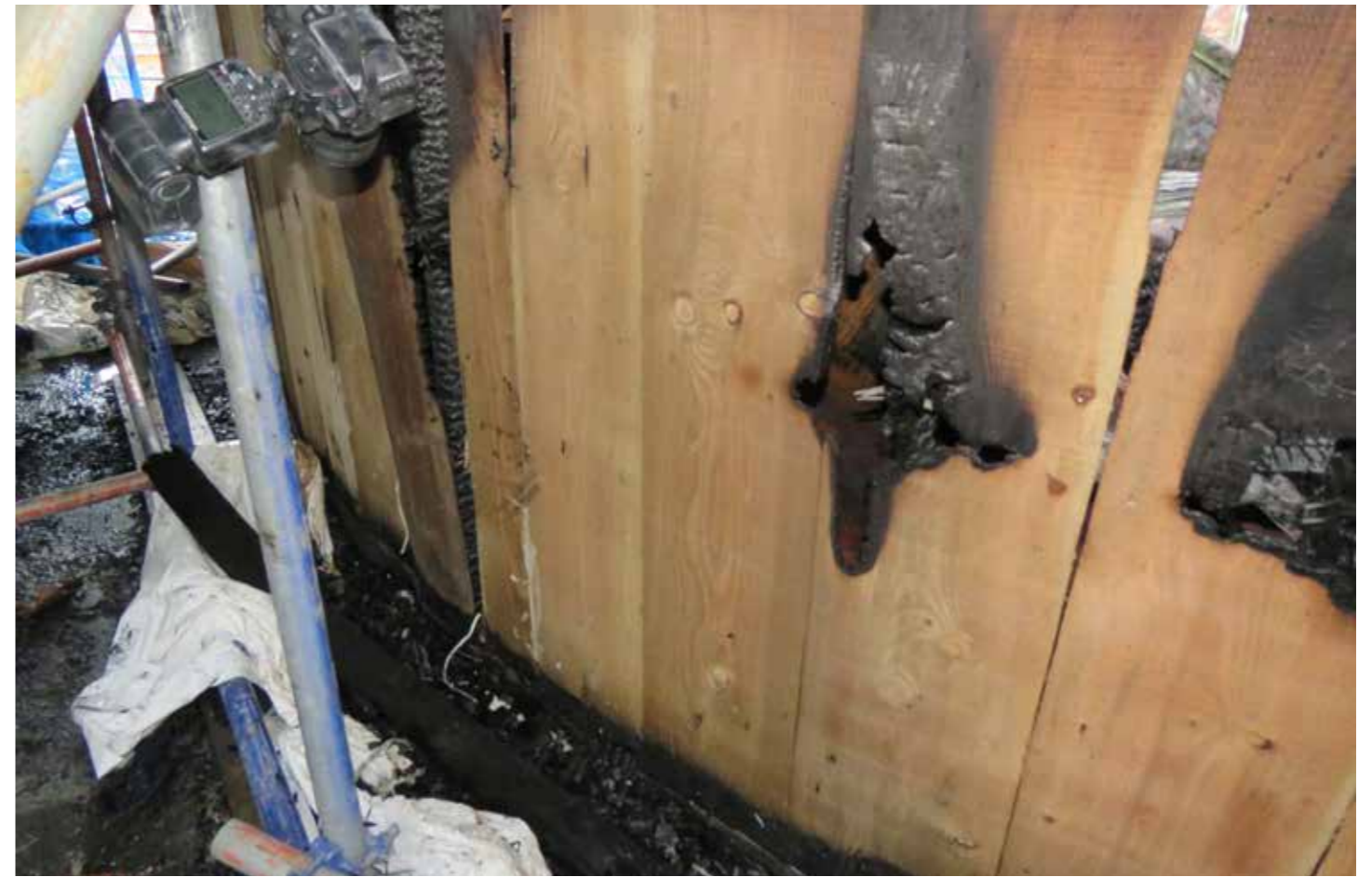
Figure 113: Wall boarding (H) in situ (exterior view) (2020) © SLHA
