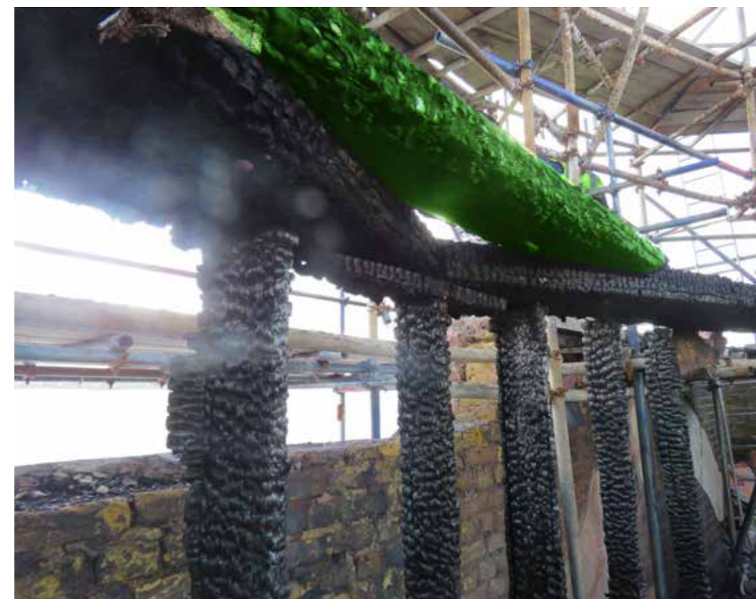
Figure 136: Horizontal rafter wall ties (M)s in situ (2020) © SLHA
