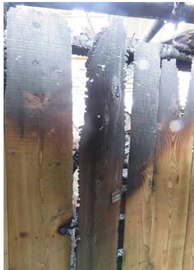
Figure 114: Wall boarding (H) in situ (exterior view) (2020) © SLHA
