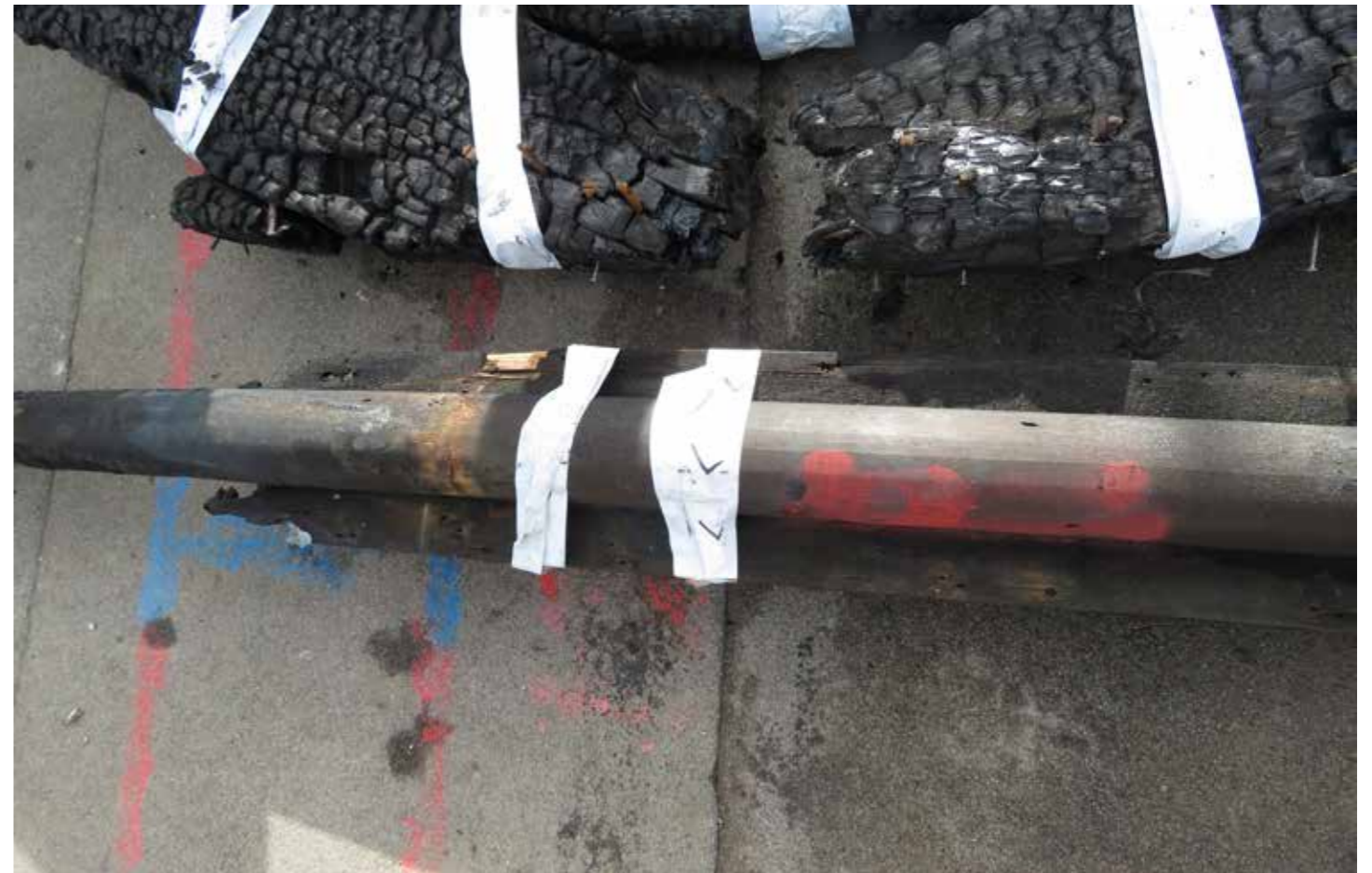
Figure 134: Sample #19 - Timber roof rolls (L) (2020) © SLHA
