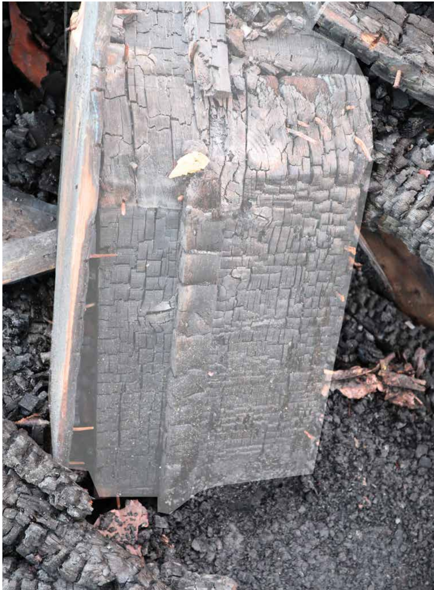
Figure 119: Sample #16 - Inner apex ring beam (I) in situ (2020) © SLHA
