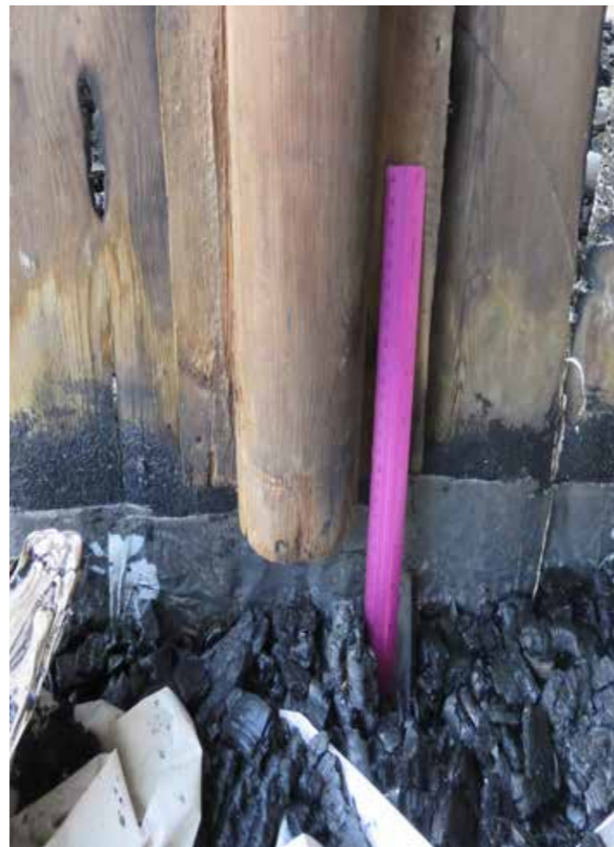
Figure 130: Timber roof rolls (L) at base level in situ (2020) © SLHA
