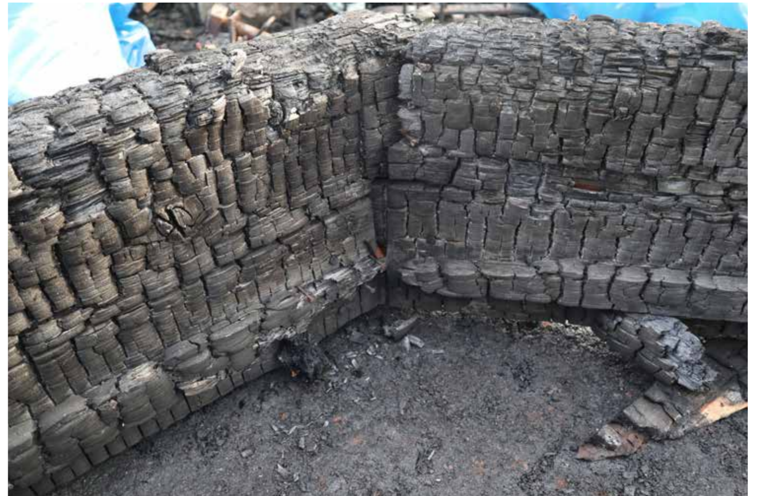
Figure 120: Inner apex ring beam (I) in situ (2020) © SLHA
