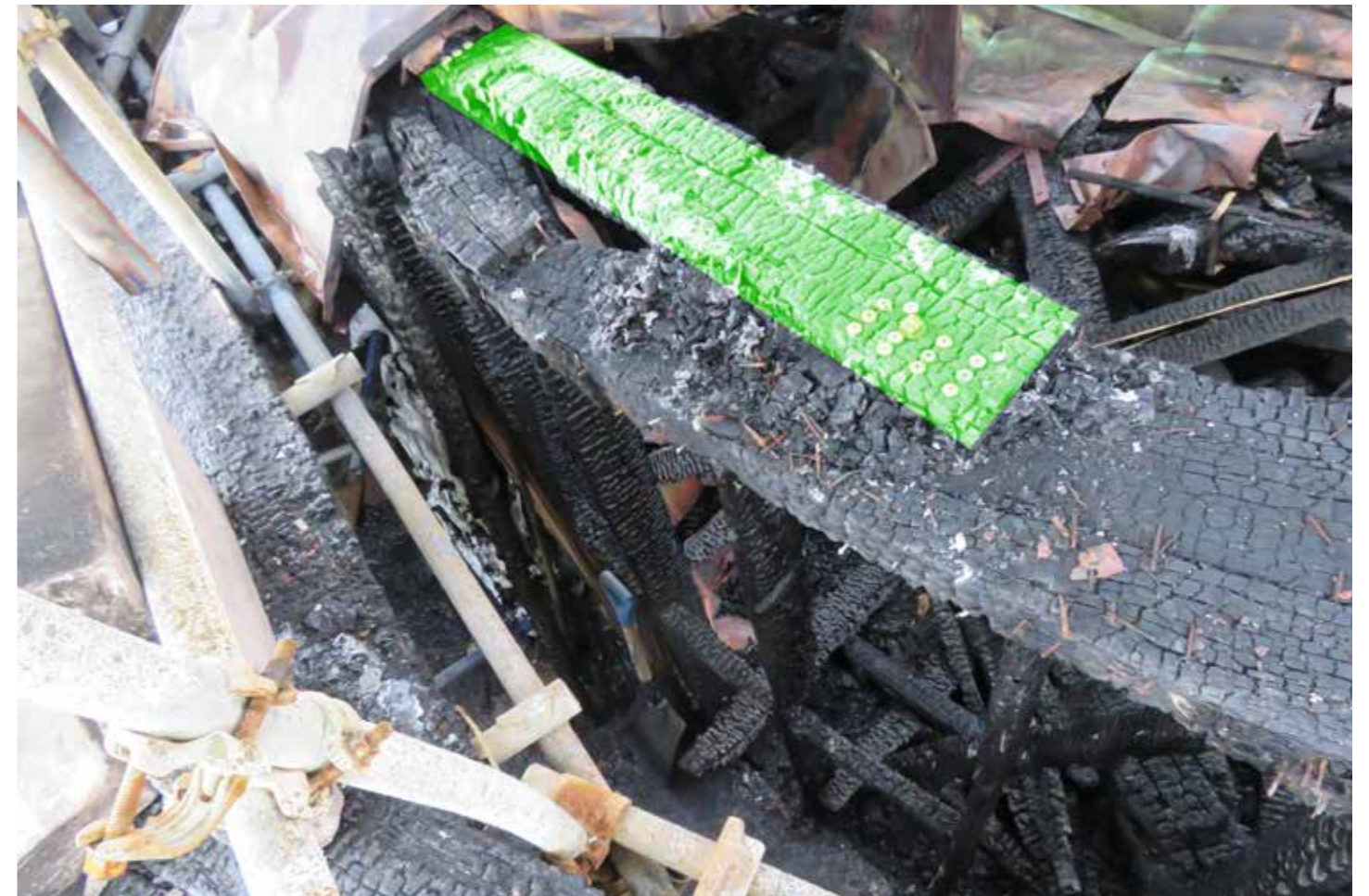
Figure 140: Horizontal rafter wall ties (M) with upper rafter plates (E) in situ (2020) © SLHA
