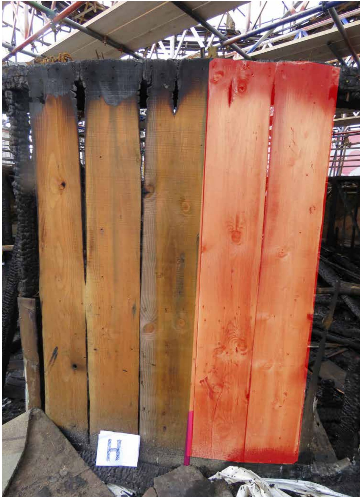
Figure 106: Wall boarding (H) in situ (exterior view) (2020) © SLHA
