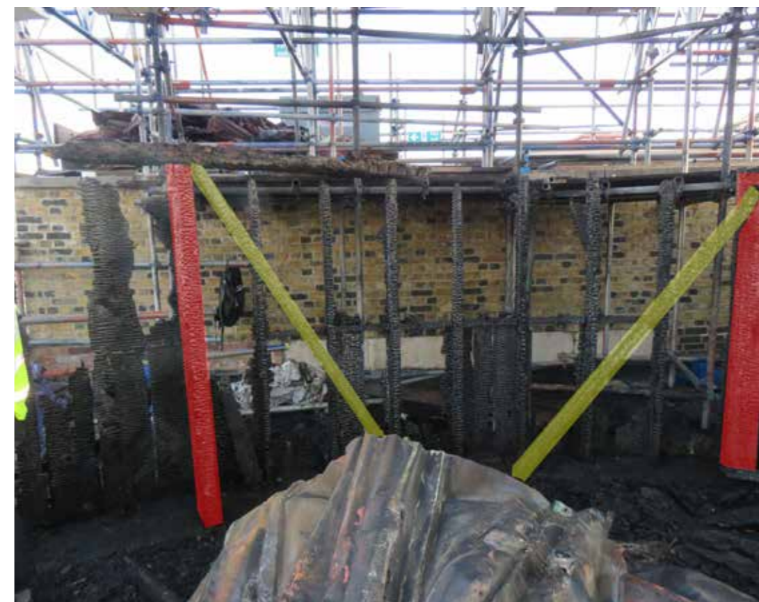
Figure 42: Main support posts (A) & Supporting braces (G) indicated in situ (2020) © SLHA
