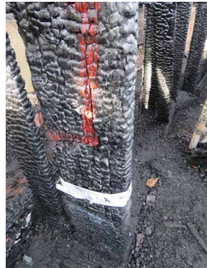
Figure 53: Main support posts (A) in situ (2020) © SLHA
