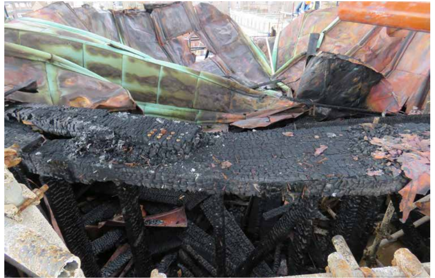
Figure 101: Upper rafter plates (E) in situ (2020) © SLHA
