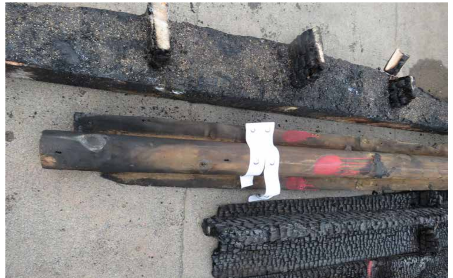
Figure 84: Sample #12 - Outer lower stud wall plate (D) with wall stud ends (B) (2020) © SLHA
