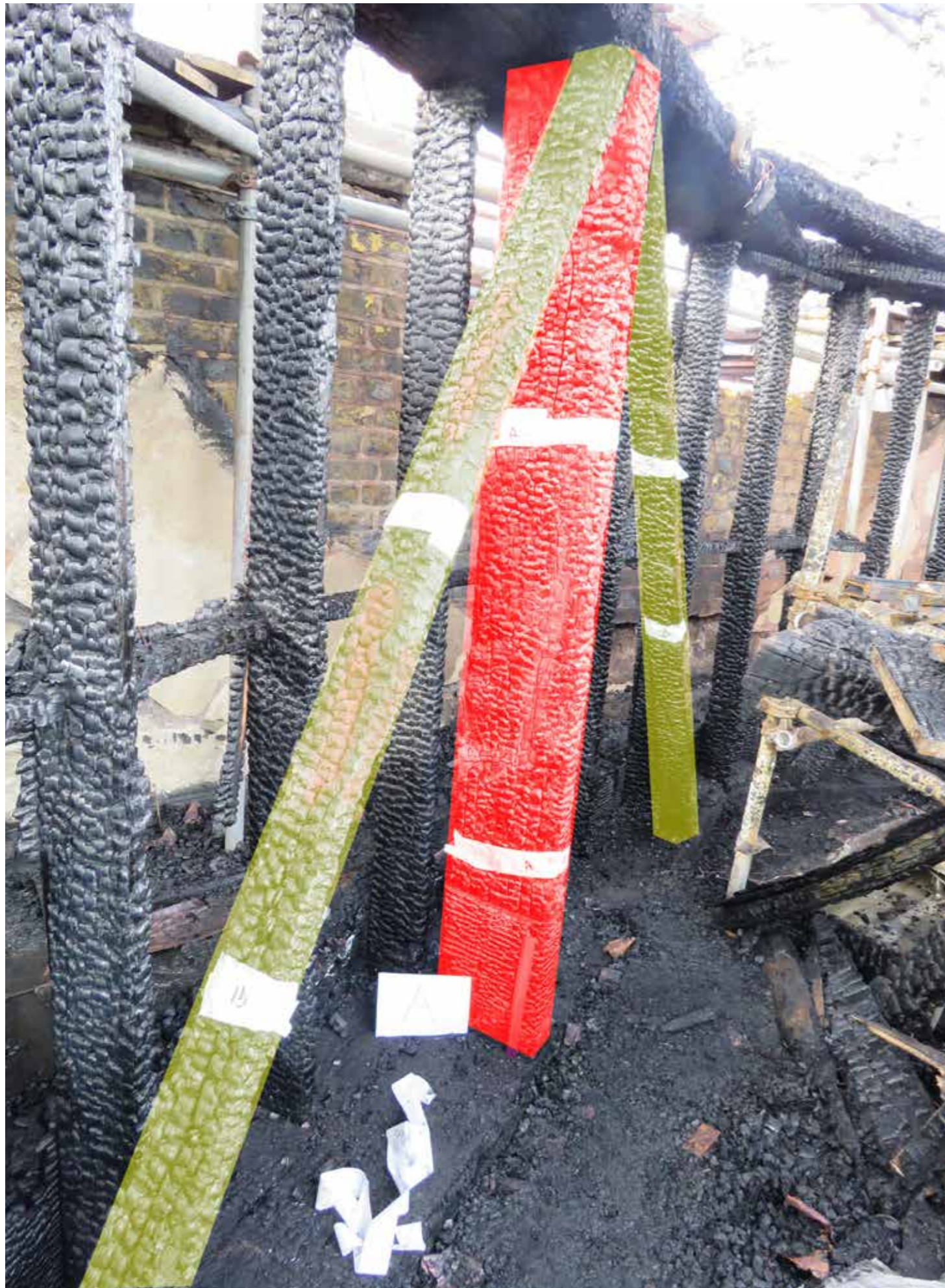
Figure 44: Main support posts (A) & Supporting braces (G) indicated in situ (2020) © SLHA
