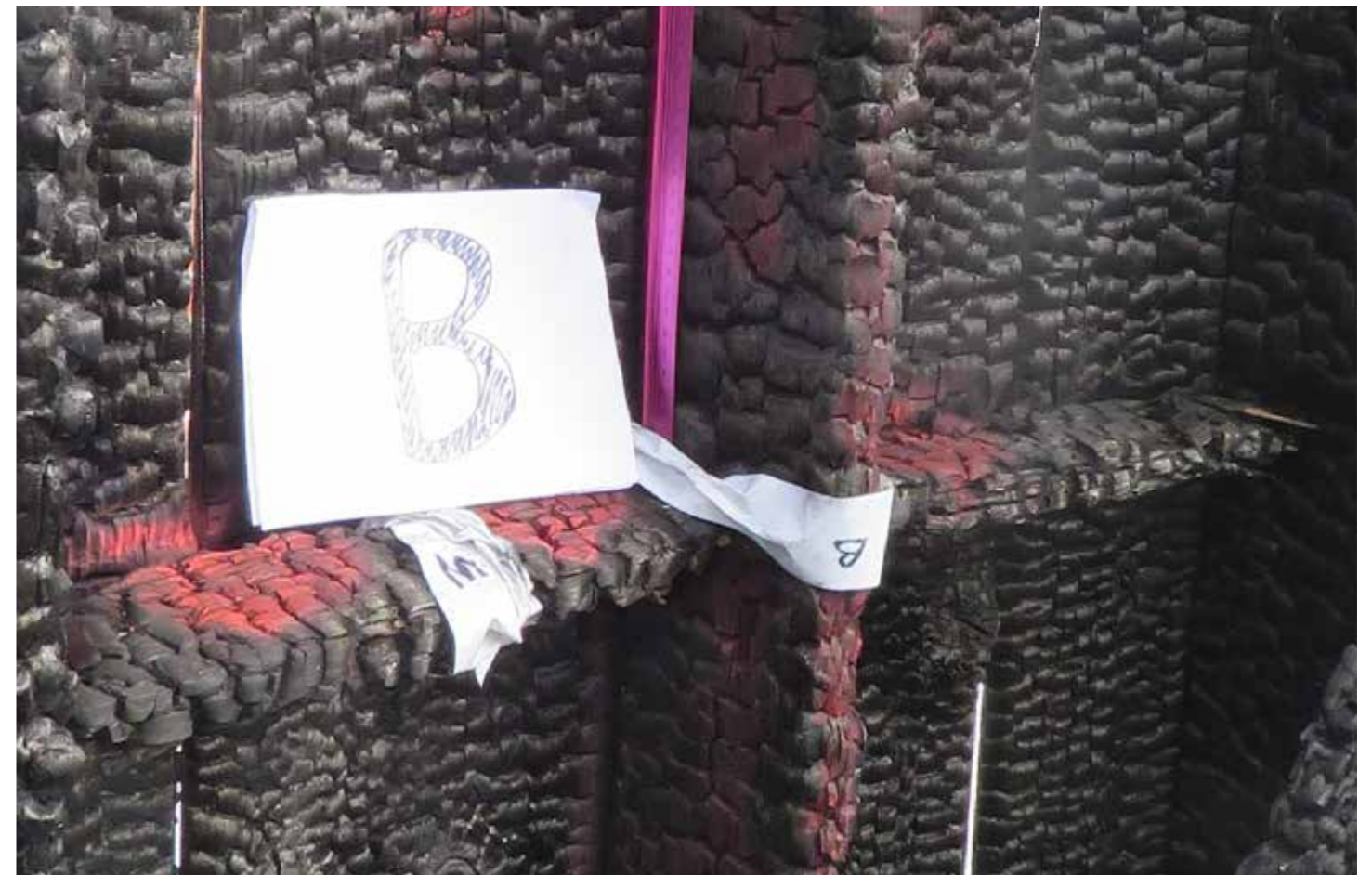
Figure 66: Wall studs and ties (B) in situ (2020) © SLHA
