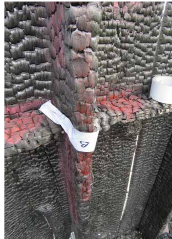
Figure 63: B- Wall studs and ties in situ (2020) © SLHA
