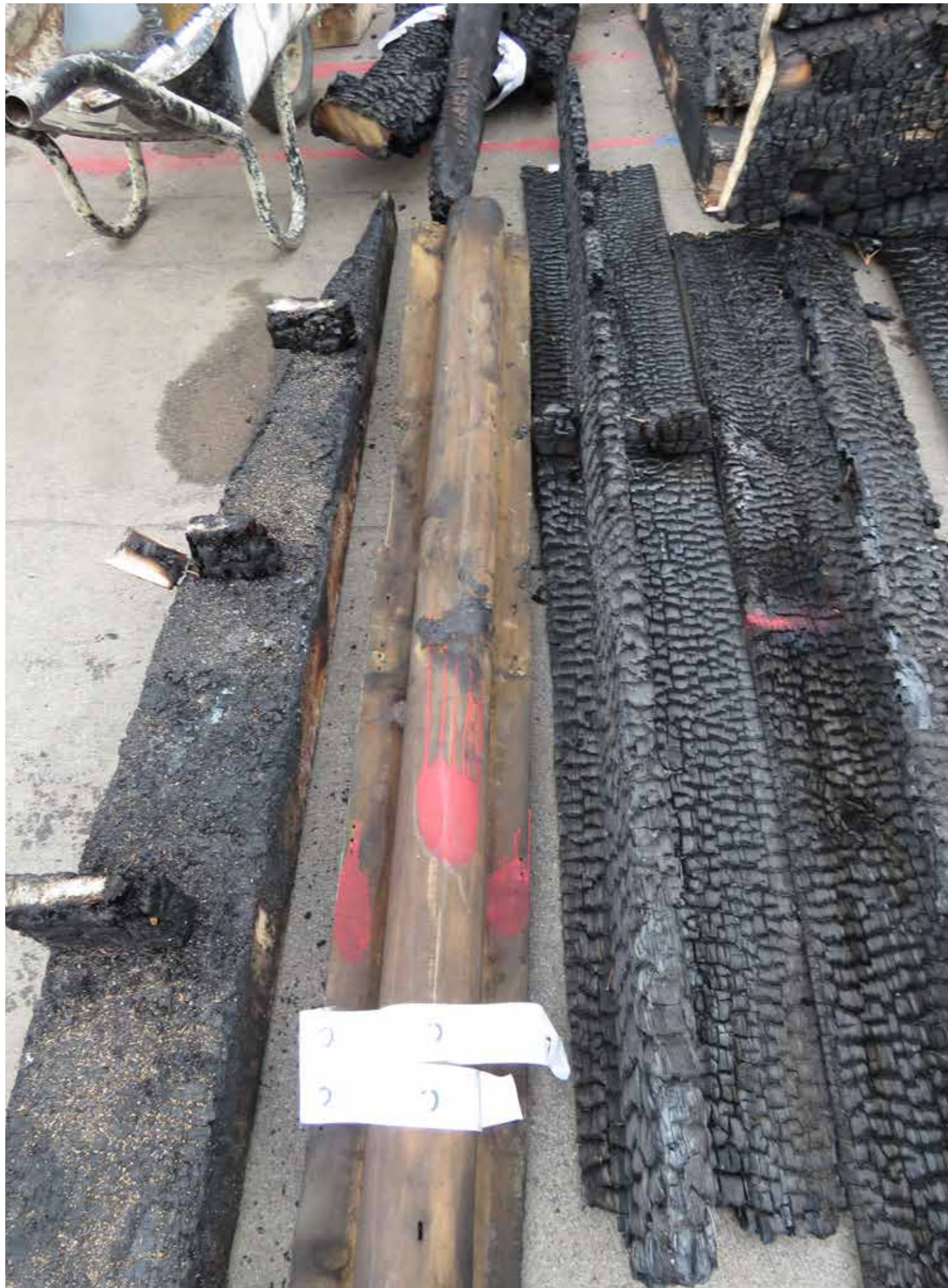
Figure 82: Sample #12 - Outer lower stud wall plate (D) with wall stud ends (B) (2020) © SLHA
