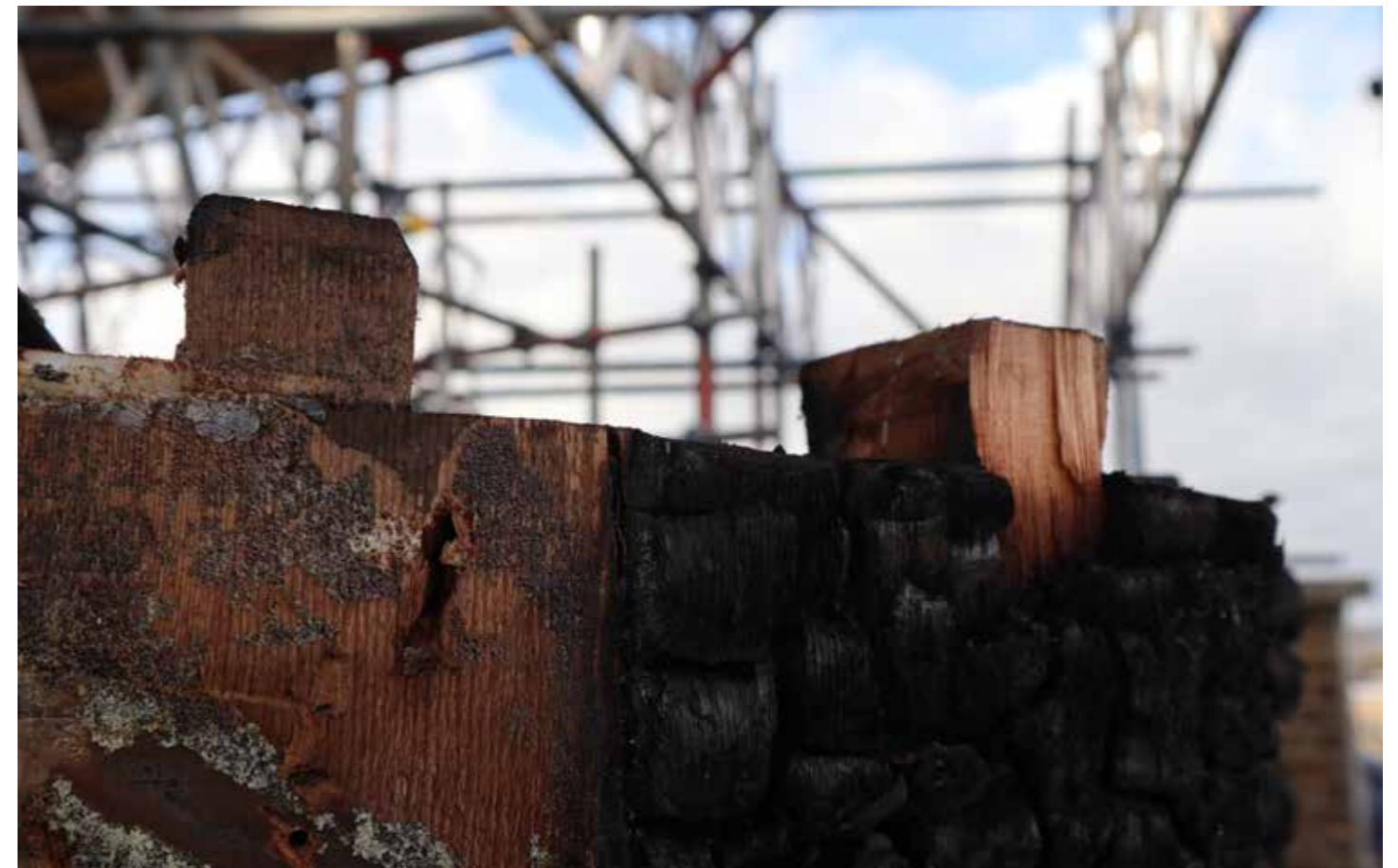
Figure 49: Sample #3 - Tenon joints at the top of main support posts (A) (2020) © SLHA
