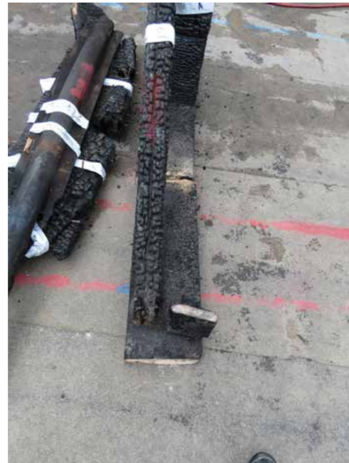
Figure 87: Sample #14 - End of inner lower stud wall plate (D1) with supporting braces (G) and overlapping wall stud (B) (2020) © SLHA
