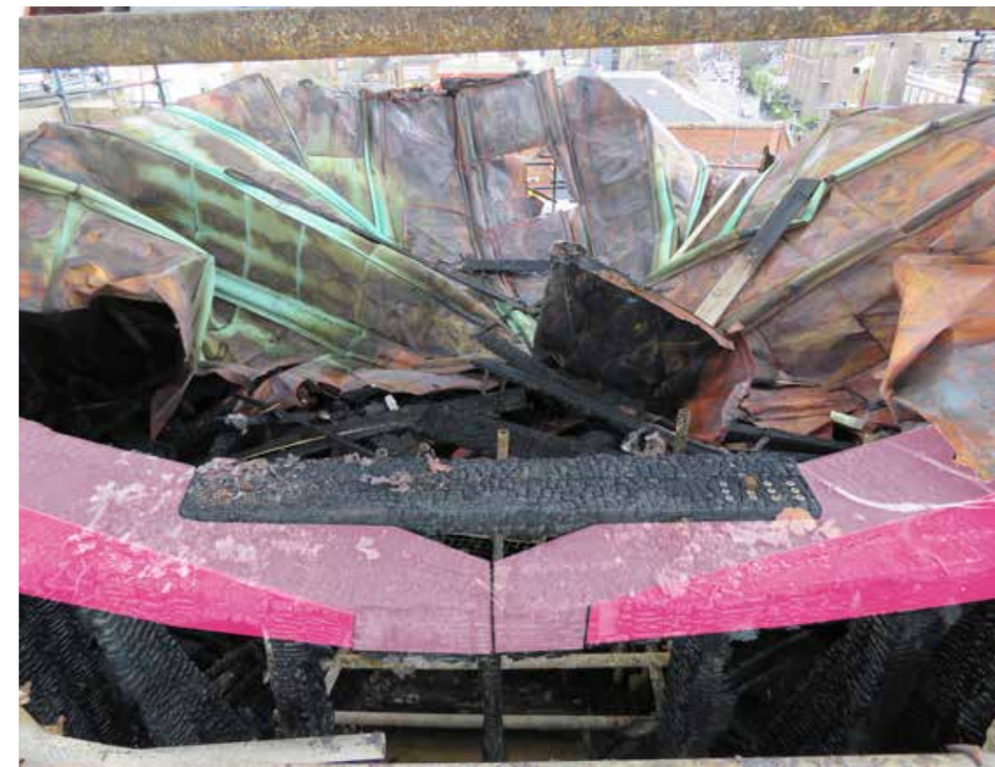
Figure 90: Upper rafter plates (E) in situ (2020) © SLHA
