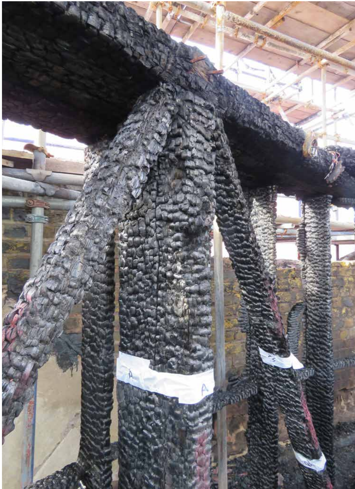
Figure 47: Main support posts (A) & Supporting braces (G) in situ (2020) © SLHA
