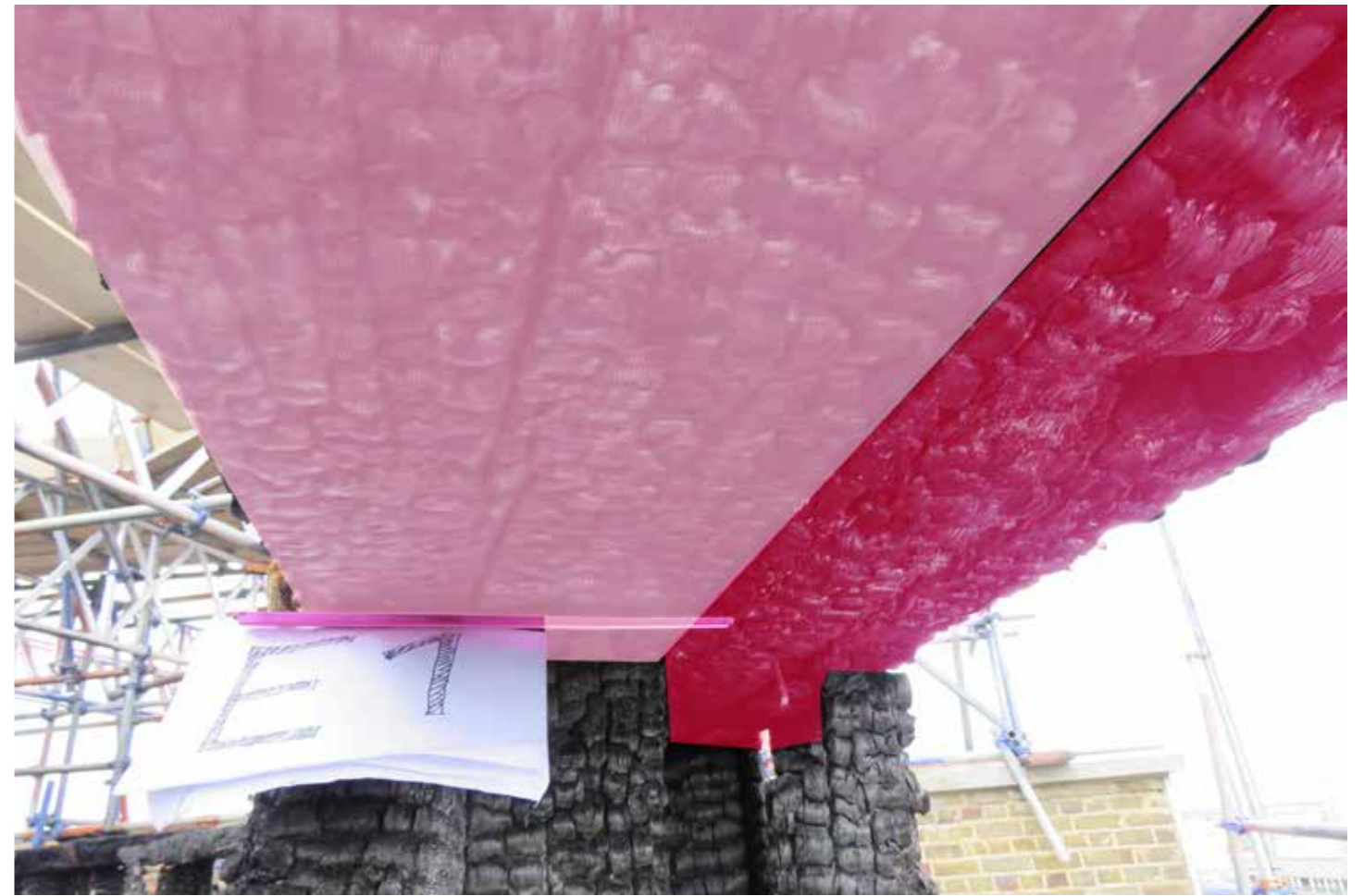
Figure 94: Upper rafter plates (E) in situ (2020) © SLHA
