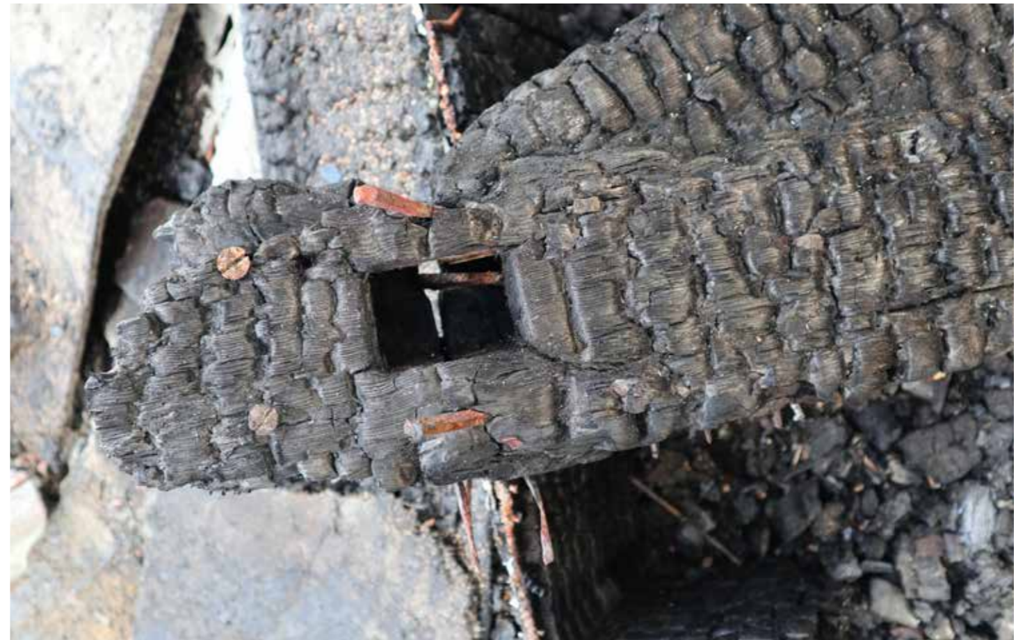
Figure 62: Mortise joint on addition plate for top of wall stud (B) to connect with upper rafter plate (E) (2020) © SLHA
