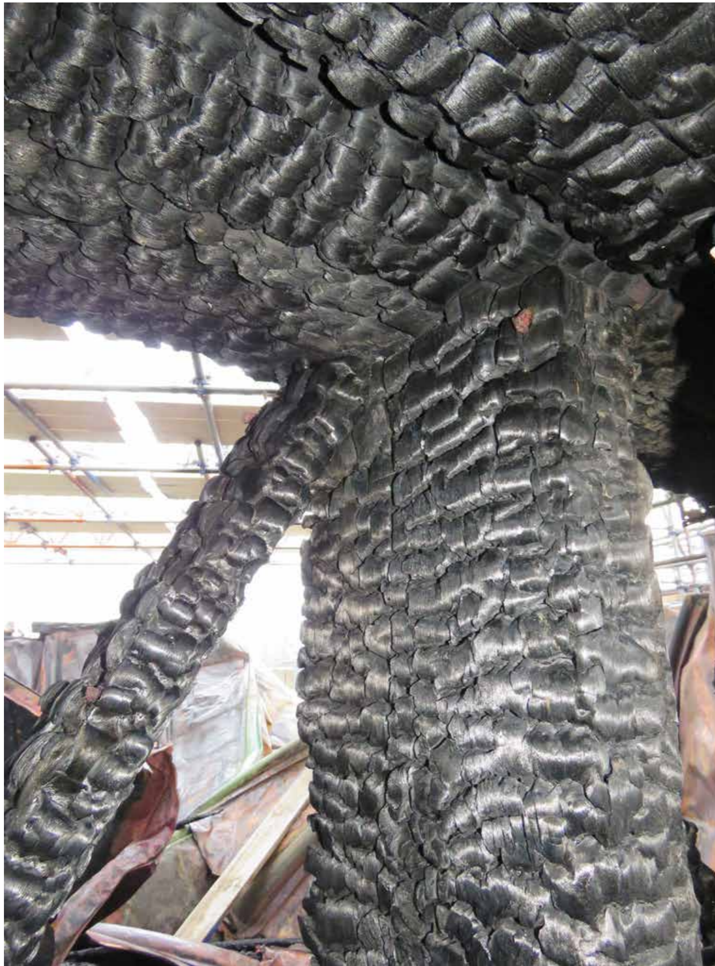
Figure 100: Inner upper rafter plates (E1) with main support post (A) and braces (G) in situ (2020) © SLHA
