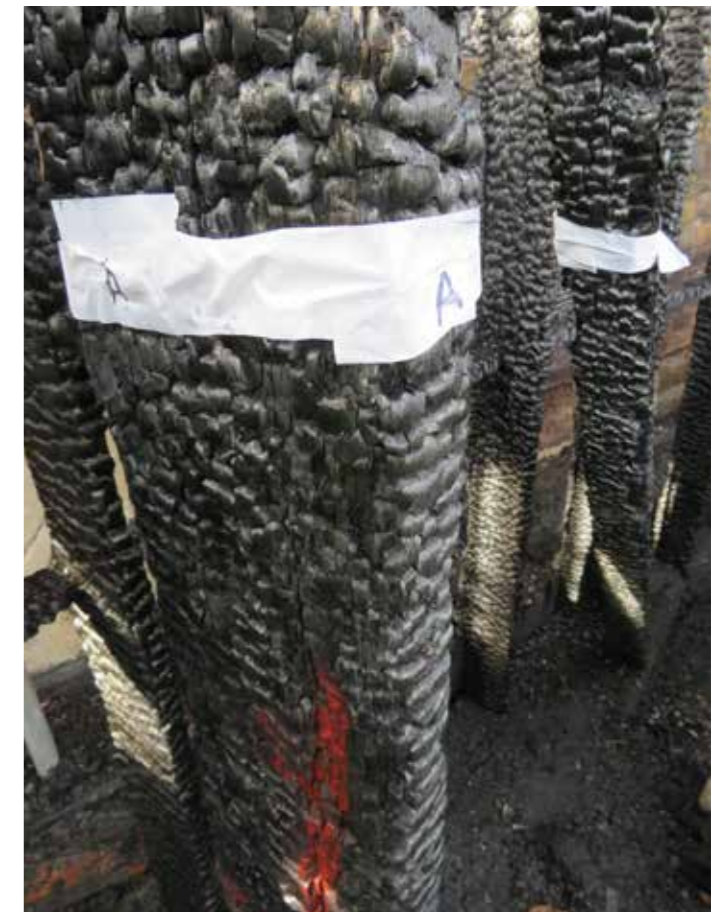
Figure 54: Main support posts (A) in situ (2020) © SLHA
