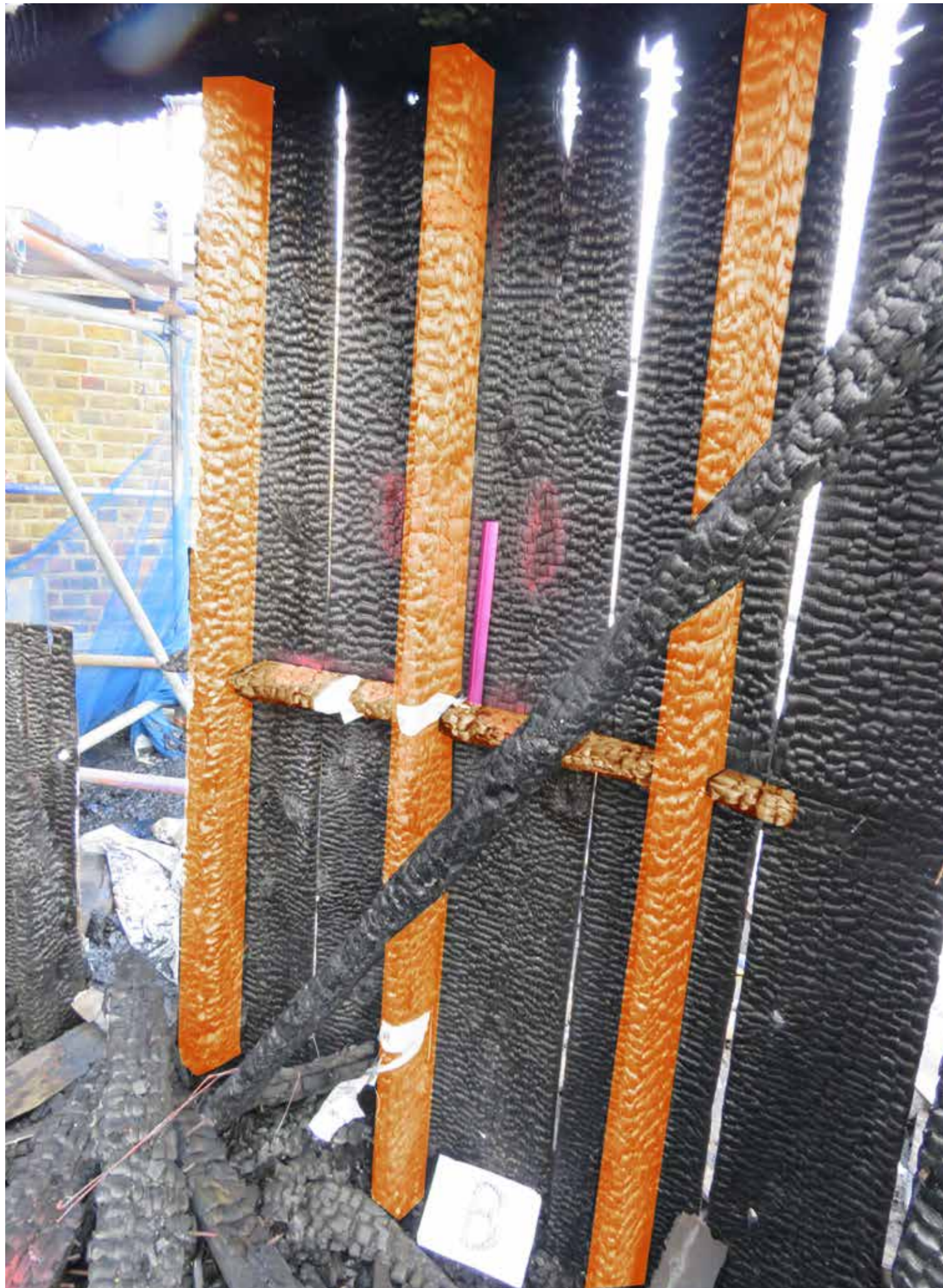
Figure 58: Wall studs and ties (B) in situ (2020) © SLHA
