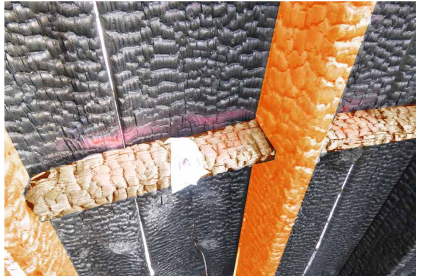
Figure 59: Wall studs and ties (B) in situ (2020) © SLHA
