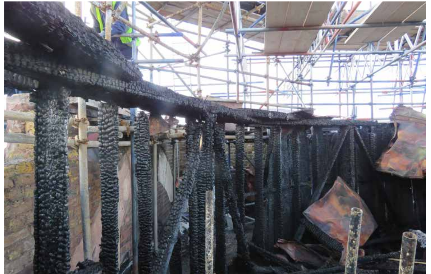
Figure 102: Upper rafter plates (E) in situ with dome wall construction (2020) © SLHA
