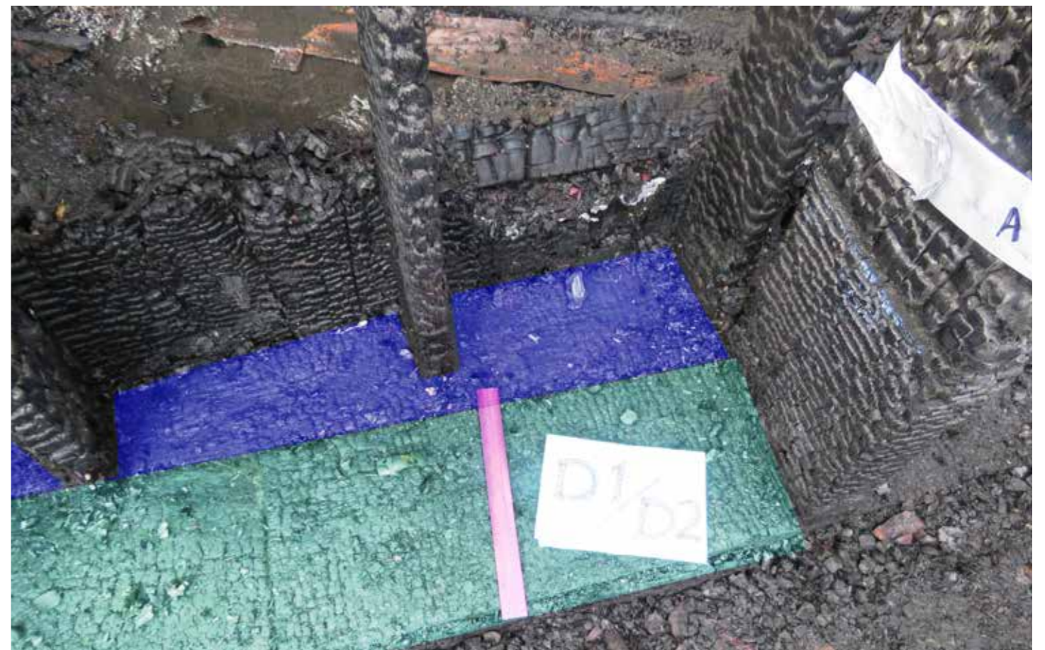
Figure 81: D- Lower stud wall plate in situ (2020) © SLHA
