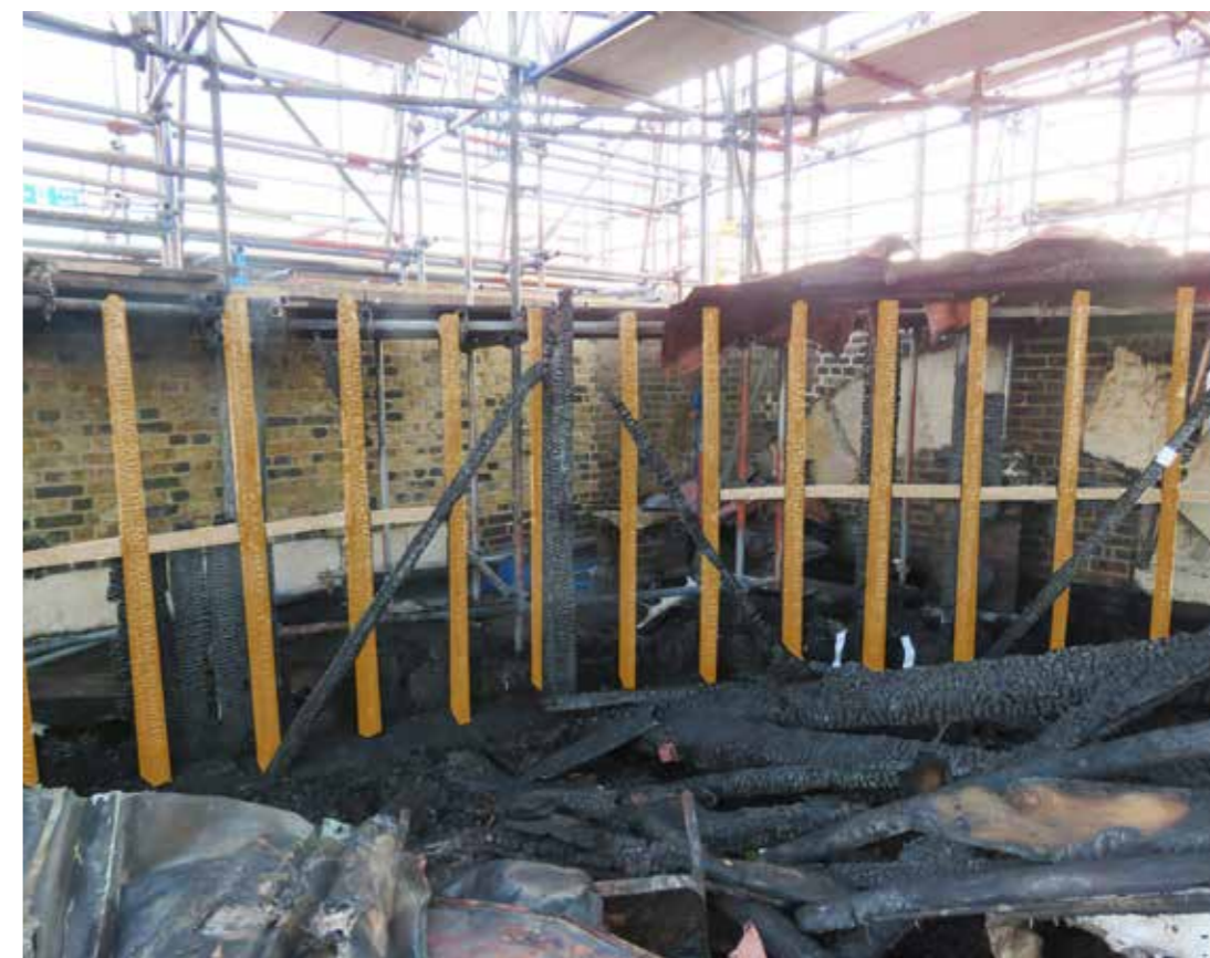
Figure 56: Wall studs and ties (B) in situ (2020) © SLHA
