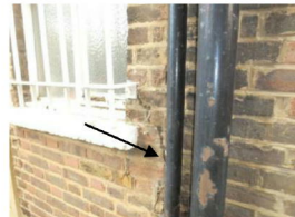
Stepped crack below ground floor bathroom rear window
