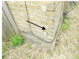
Stepped crack to brickwork – front left corner
