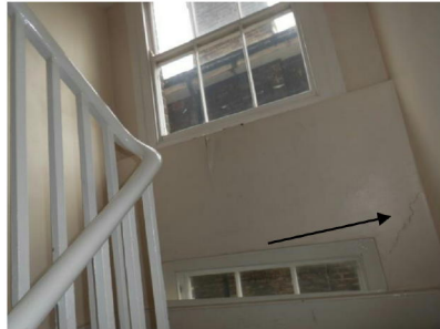
Mid landing rear window – cracks around window
