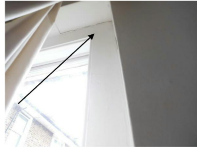
Separation crack around flat 4 rear bedroom window
