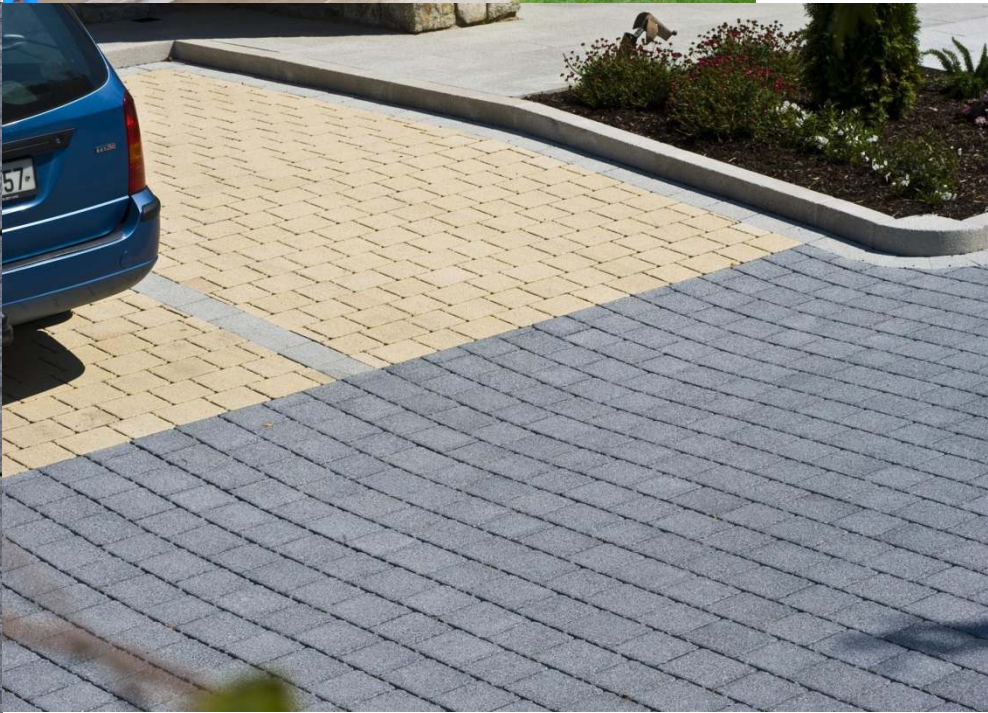
Driveway: Tobermore Hydropave Tegula Charcoal permeable block paving
