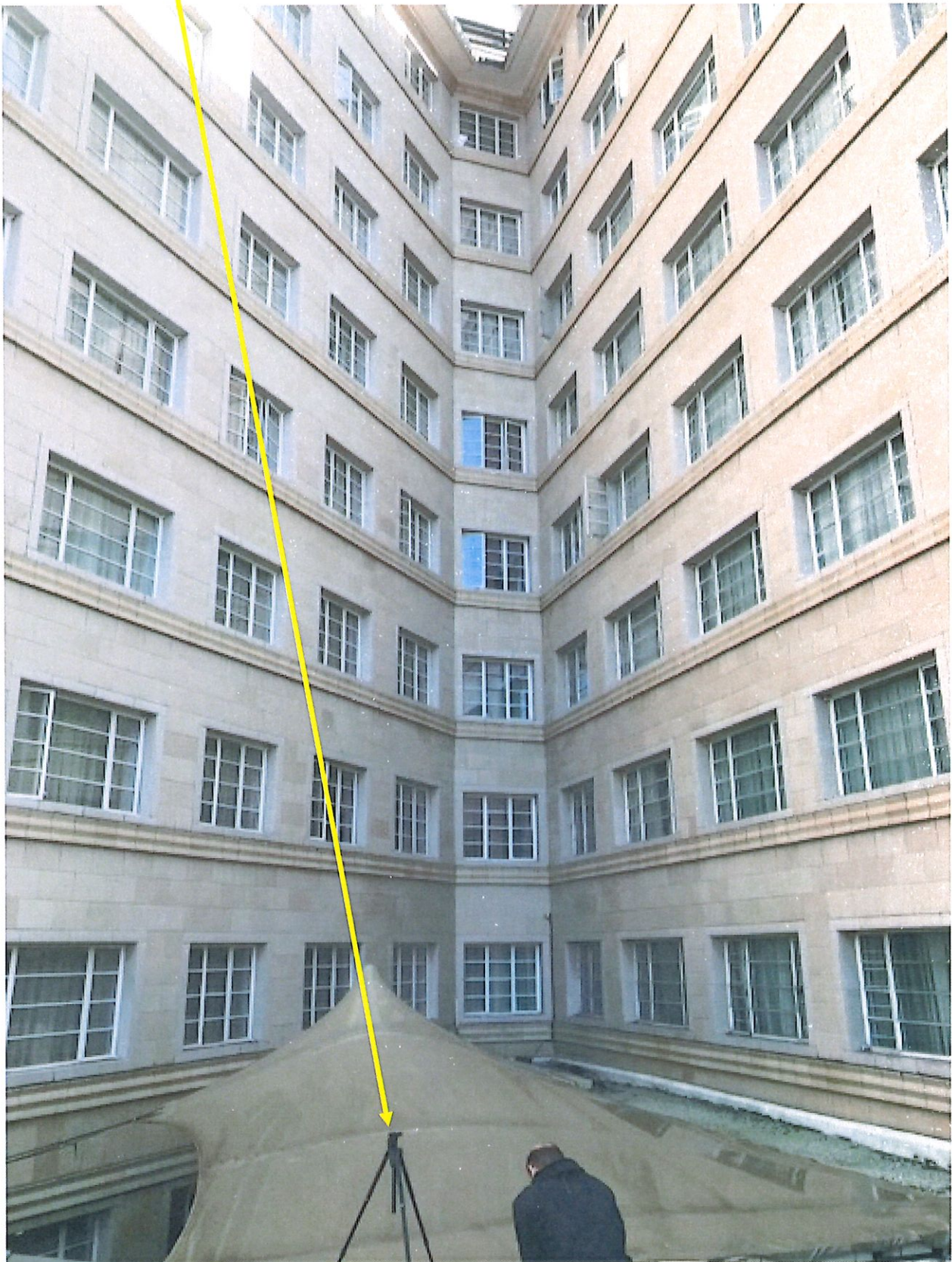
Photo B – View of hotel facades which surround and face the plant room roof
