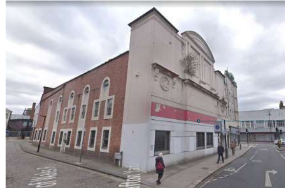
Former cinema on north side of Prince of Wales Road near junction with Kentish town Road
