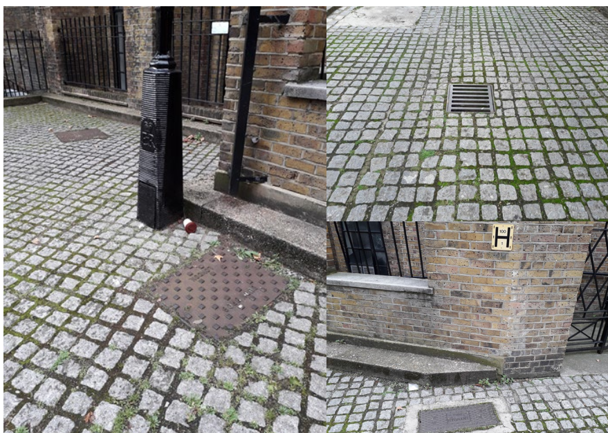
Photograph Plate B – Several manhole covers were recorded around the perimeter of the site, indicating the presence of underground services.
