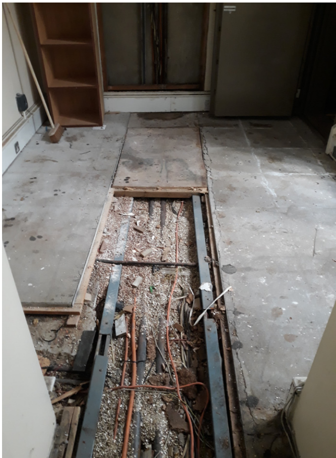
Photograph of the existing service trench in the basement slab
