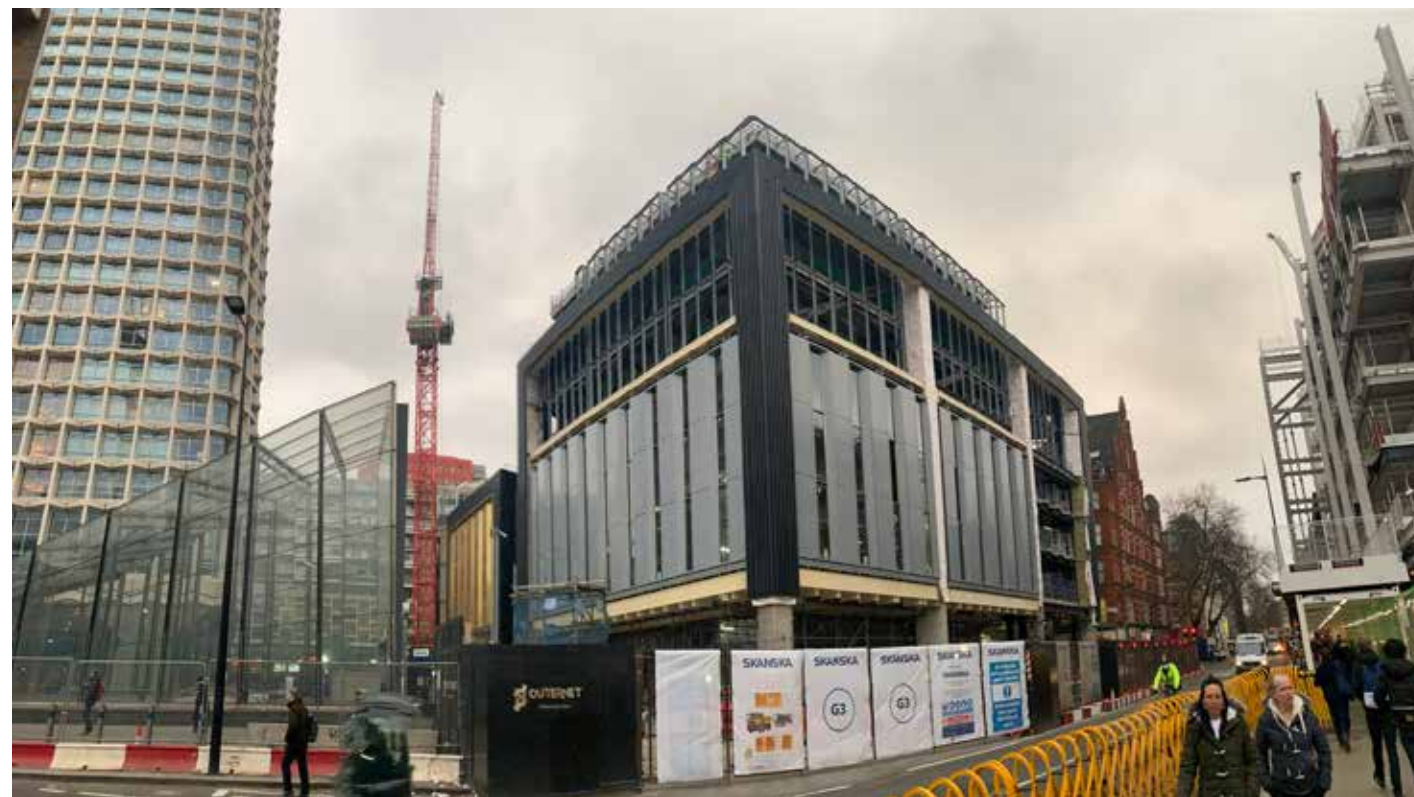
Figure 3.5 Primary frontage of the site with fins installed where the proposed retractable external skin is intended for installation
