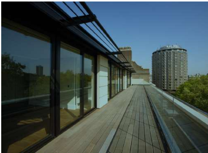
Photo 2: New penthouses above Lowndes Square
