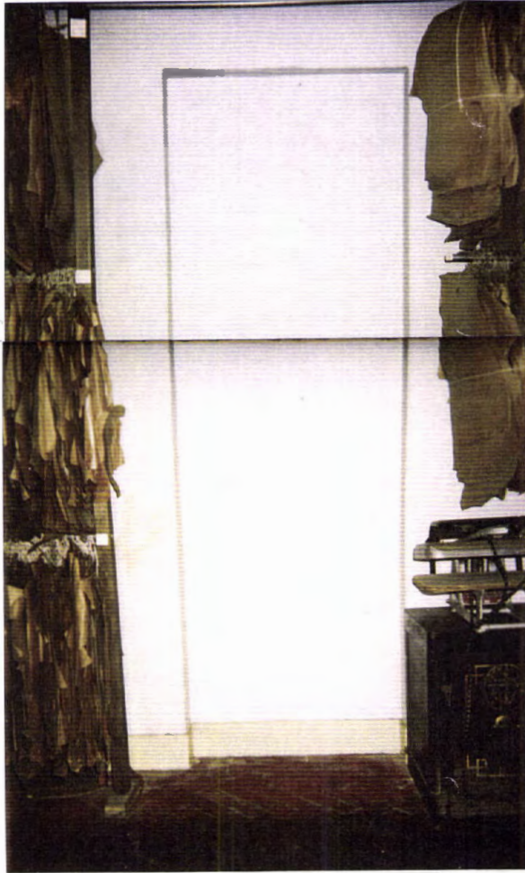
PHOTOGRAPH OF SECTION OF WALL WHERE FIRE ESCAPE IS PROPOSED
