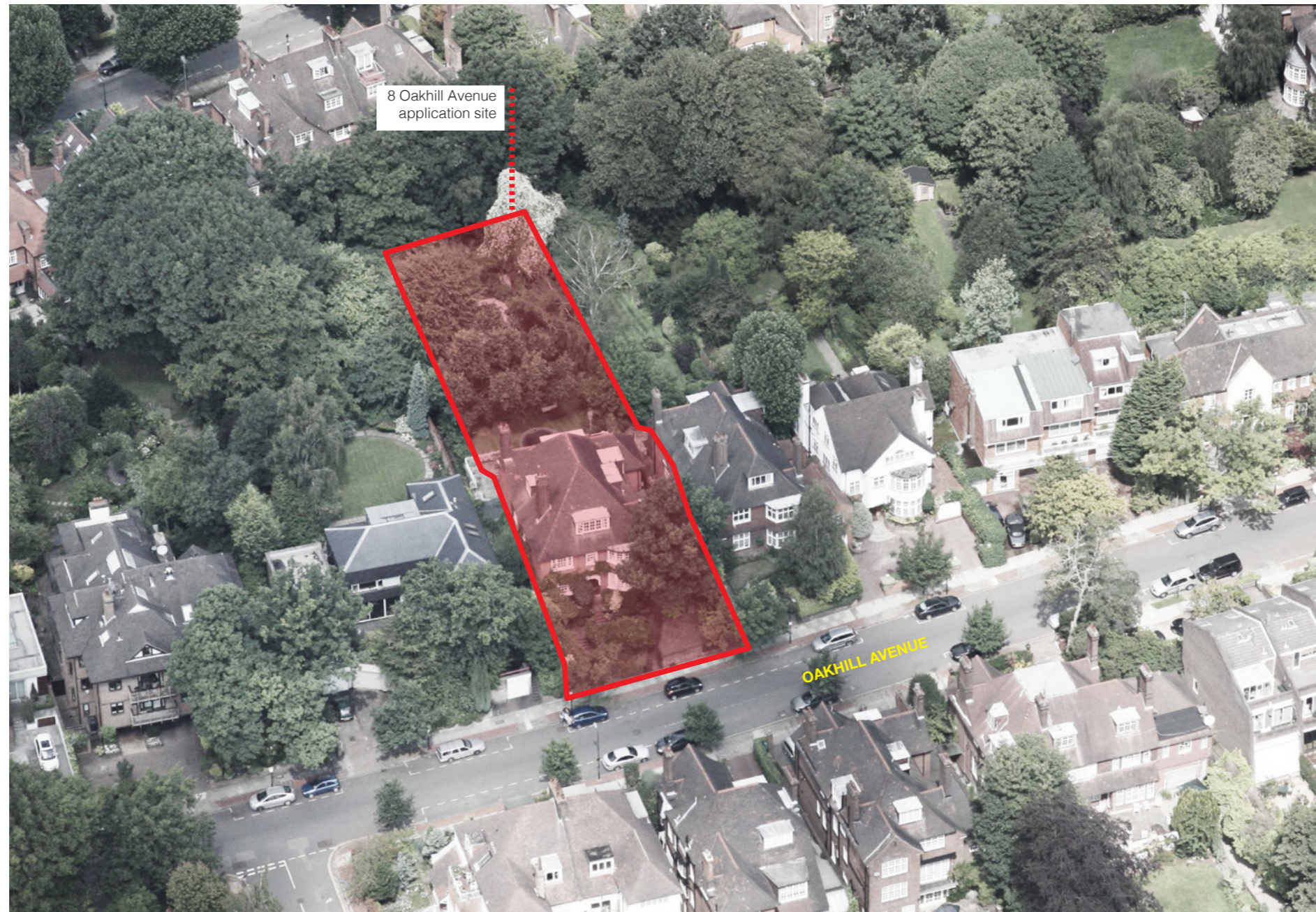
Fig 2: Aerial view of site and surrounding context
