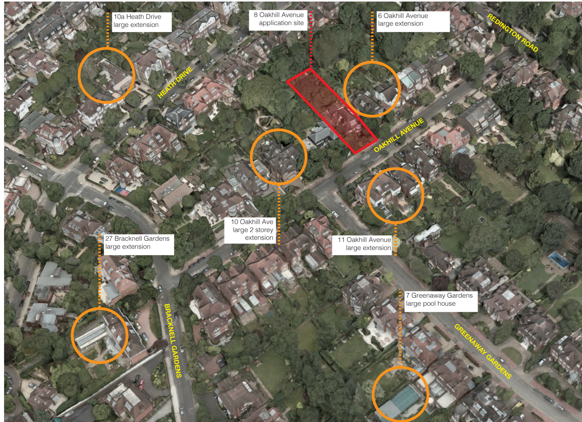
Fig 30: Aerial view of site and wider context. Circles denote large + deep extensions within the conservation area
