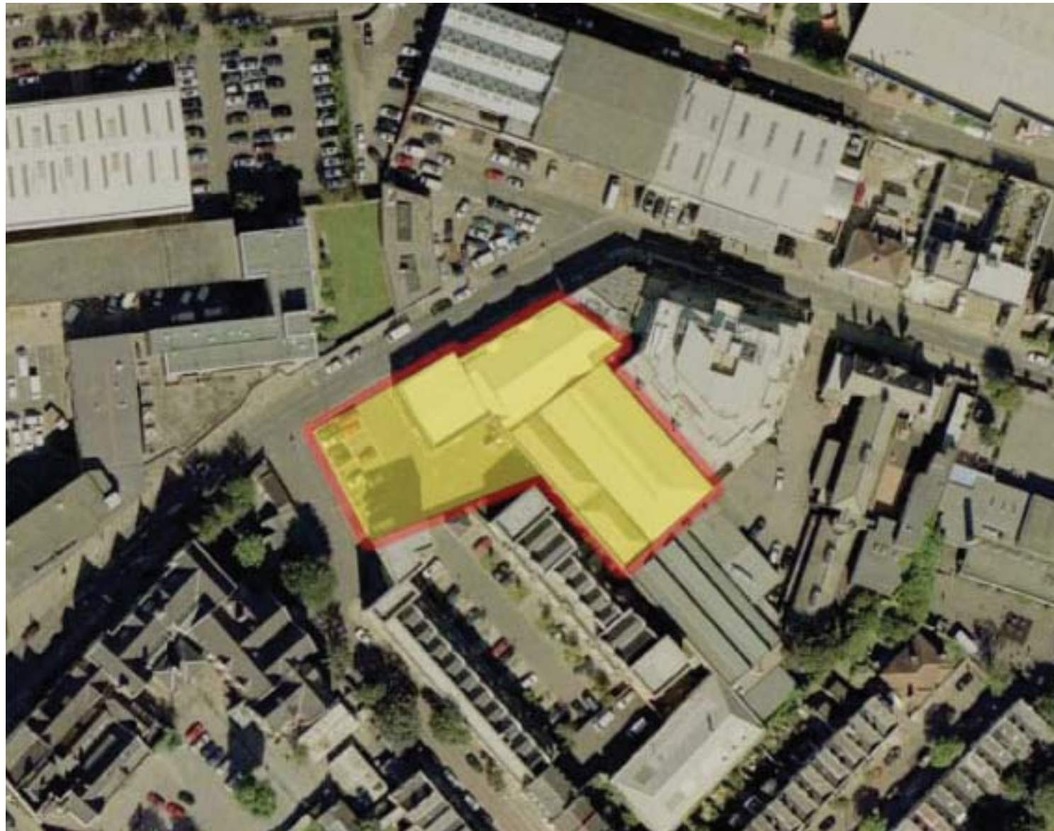
Aerial Photograph Showing Site Location
