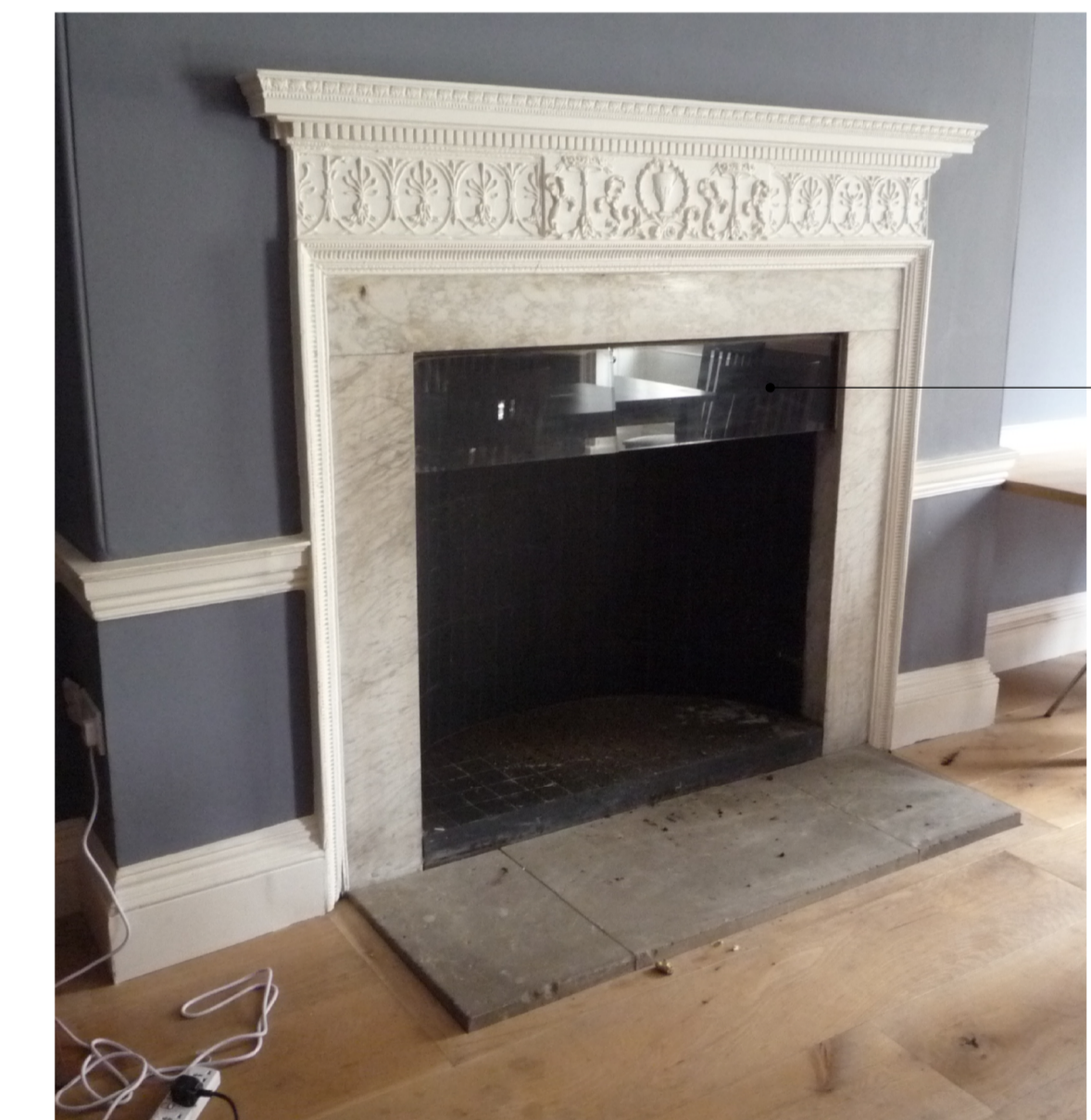
CHIMNEY PIECE IN ONSITE STORAGE TO BE REINSTATED
