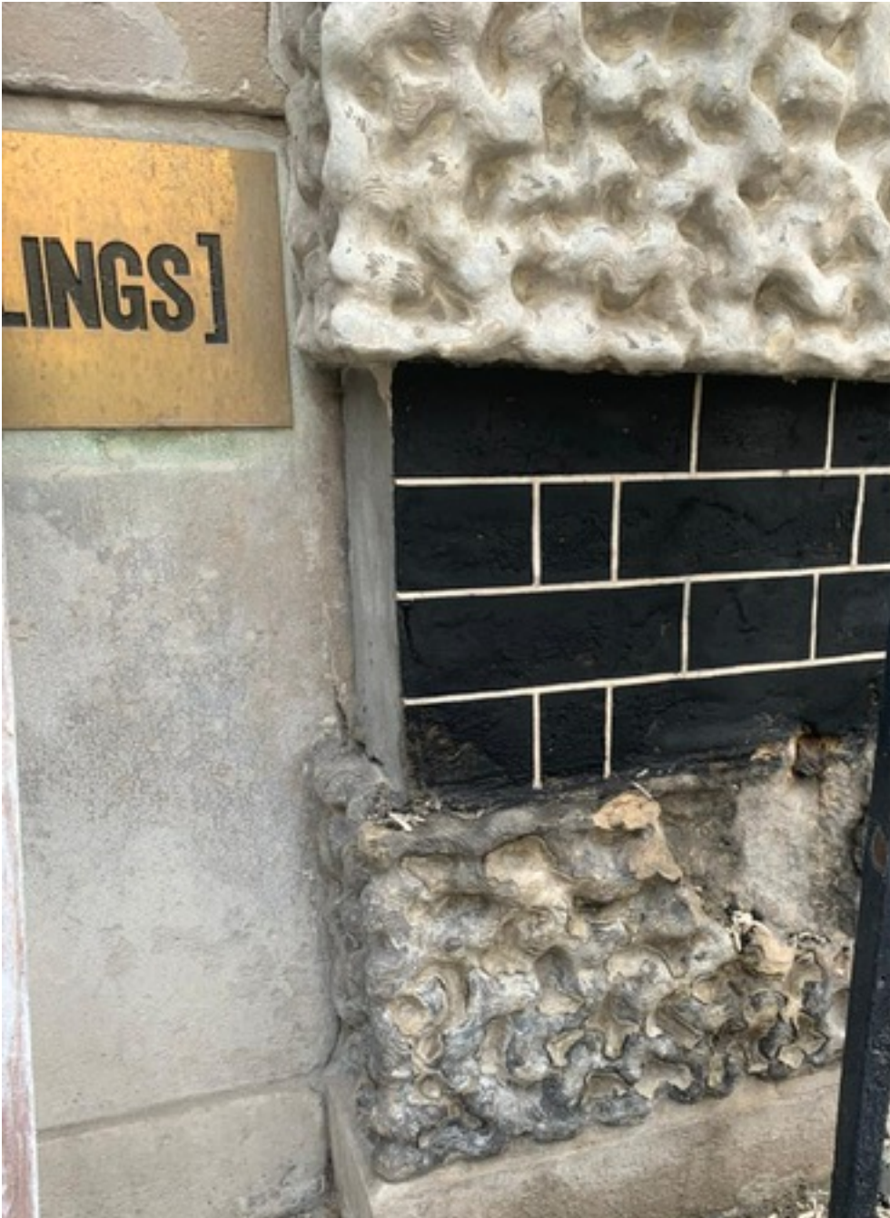
1 Proposed Brick Sample - Front Elevation 41 Bedford Square PL_055 NTS • DOFF cleaned • Applied stopping mortar • 4mm tuck pointing
