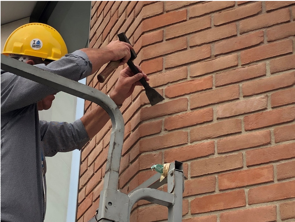
Figure 6 Mechanically removing arris lips
