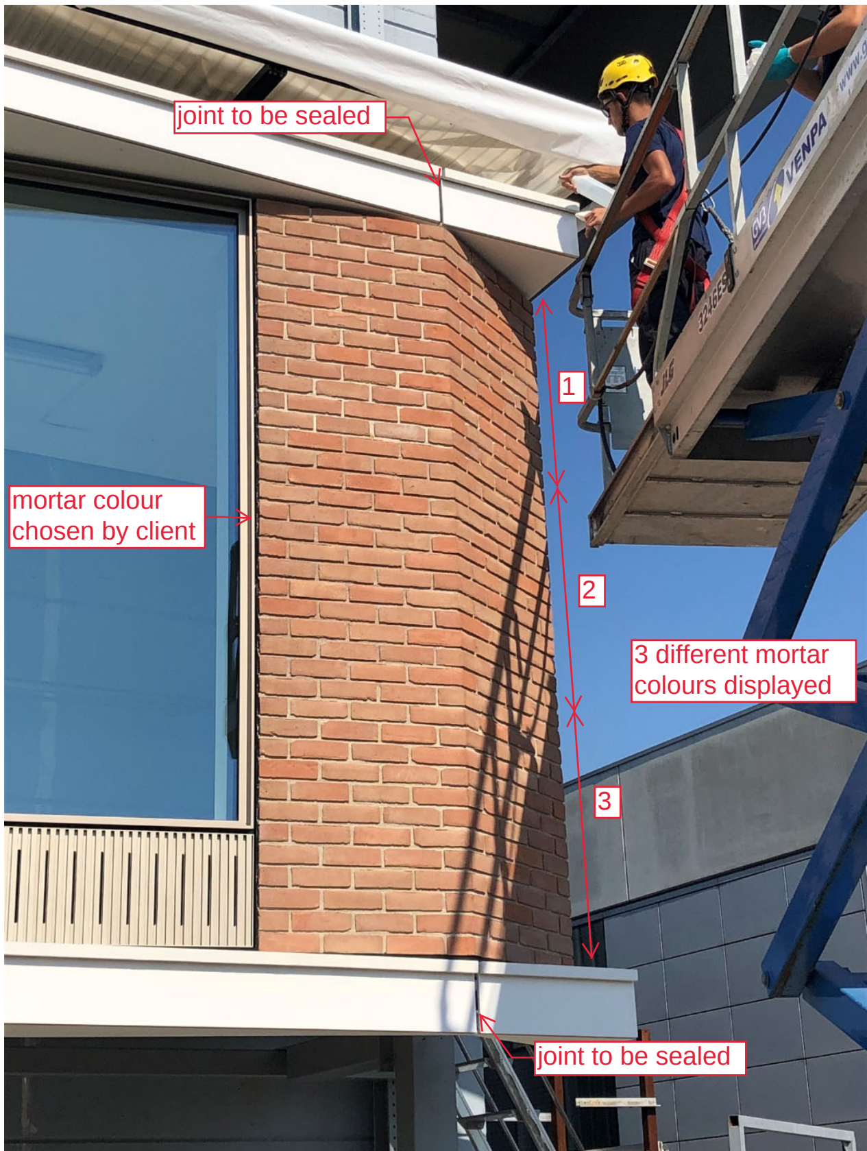
Figure 4 Close up of VMU. Note three different mortar colours in equal sized bands (light: top 13 courses; dark: middle 12 courses; medium: lower 13 courses)
