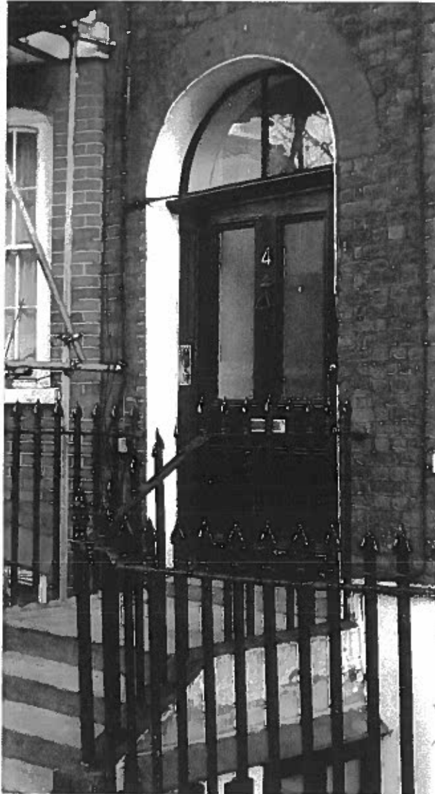
5. Oblique view of 4 Handel Street front door (frame, door and fanlight to be replaced)
