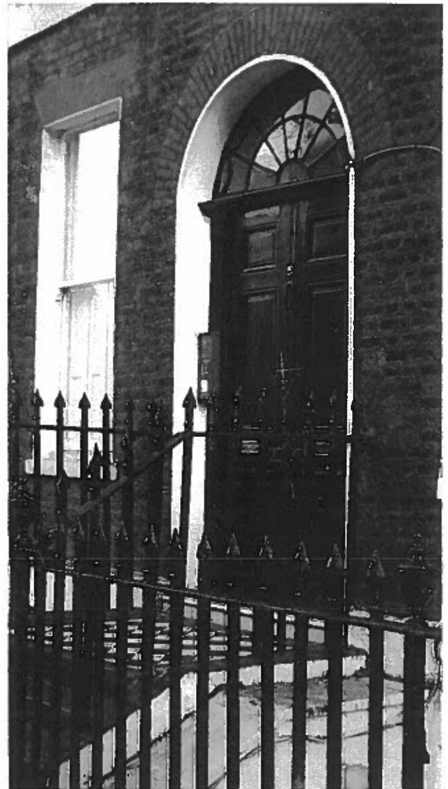
6. Oblique view of 5 Handel Street front door (frame, door and fanlight to be copied)
