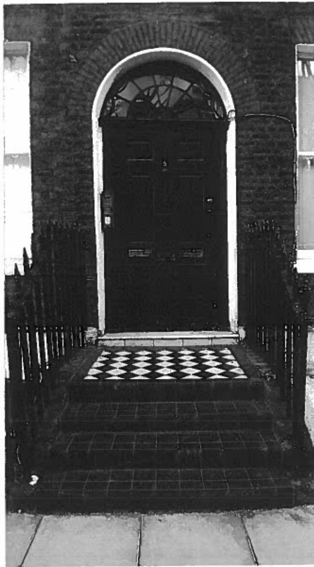
4. Close up view of 5 Handel Street front door (frame, door and fanlight to be copied)
