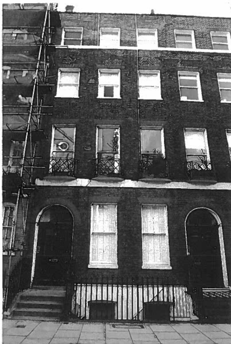
1. View of 4 Handel Street showing front door (frame, door and fanlight to be replaced) and adjoining 5 Handel Street (front door, frame and fanlight to be copied)
