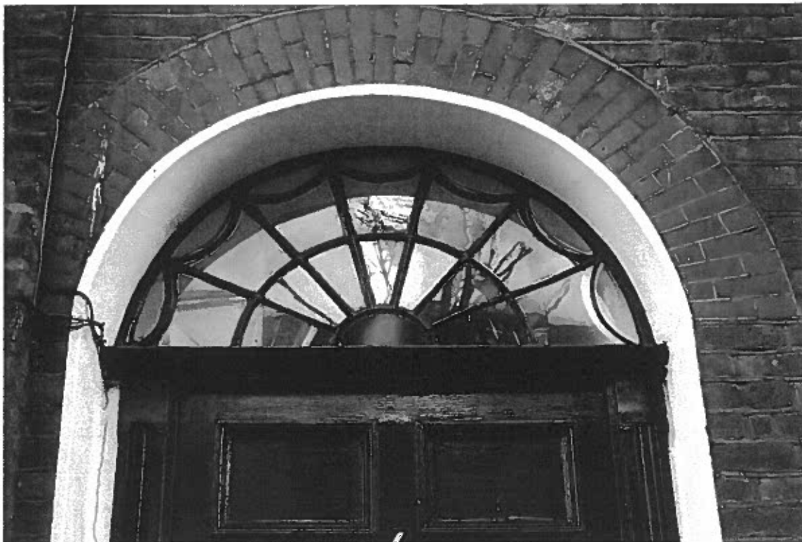
7. Close up view of 6 Handel Street fanlight which is identical to 5 Handel Street (to be copied)
