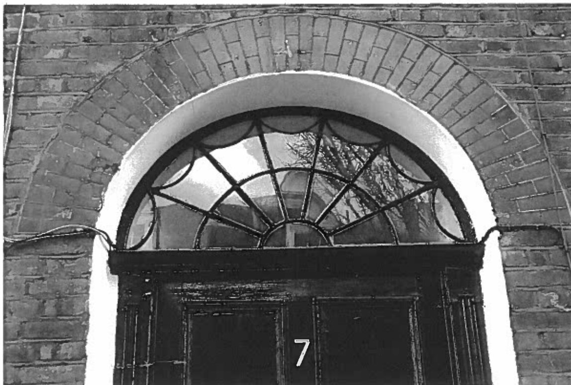
8. Close up view of 7 Handel Street fanlight which is identical to 5 and 6 Handel Street (to be copied)
