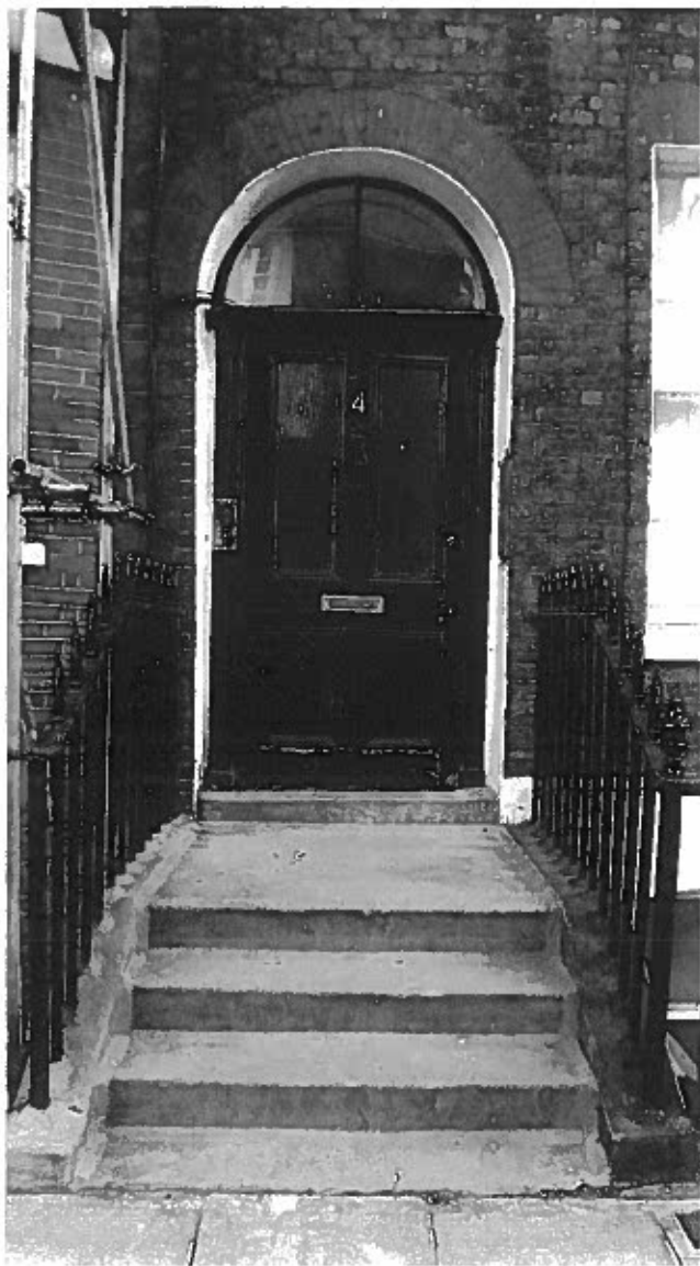
3. Close up view of 4 Handel Street front door (frame, door and fanlight to be replaced)
