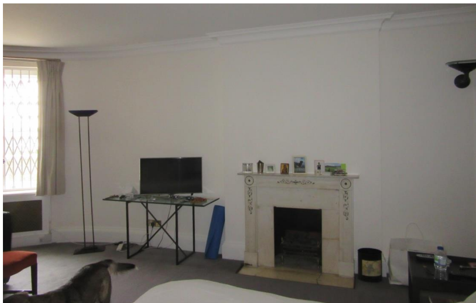
Figure 26: One of the principal first-floor bedrooms showing original cornicing, joinery and fire surround.
