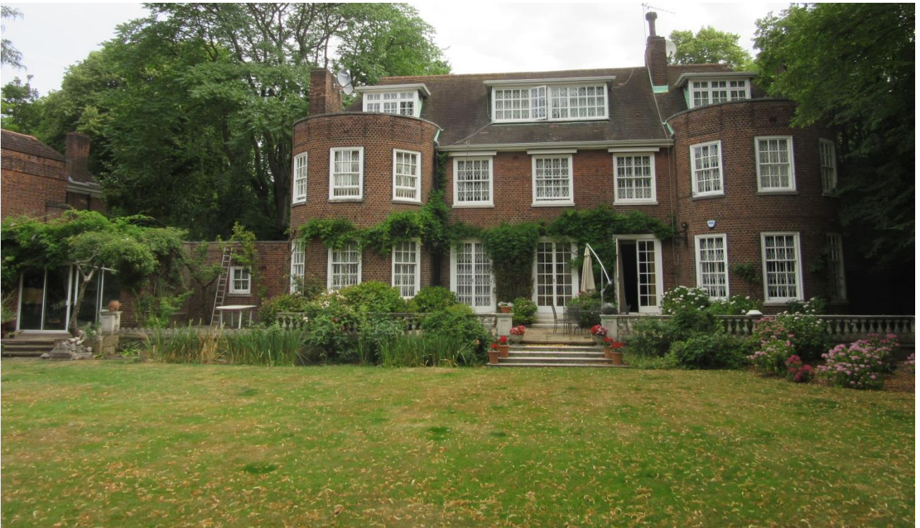
Figure 18: The rear garden elevation of No. 69.
