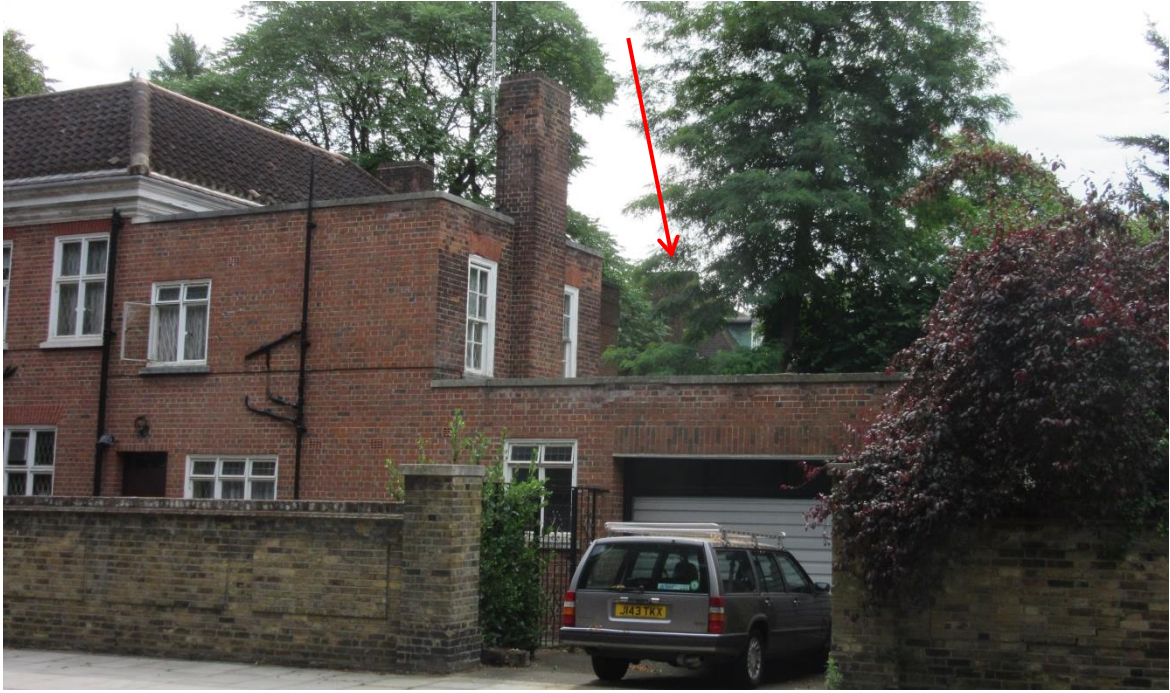
Figure 6: The rear elevation of the subject site (indicated) is only glimpsed from Queen's Grove outside the St John's Wood Conservation Area.
