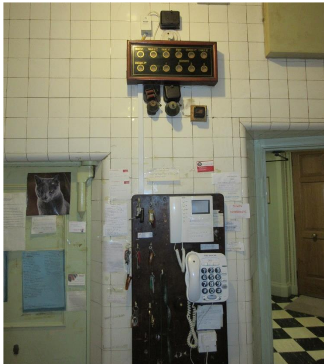
Figure 20: Original tiling and servants’ bell-box within the pantry.
