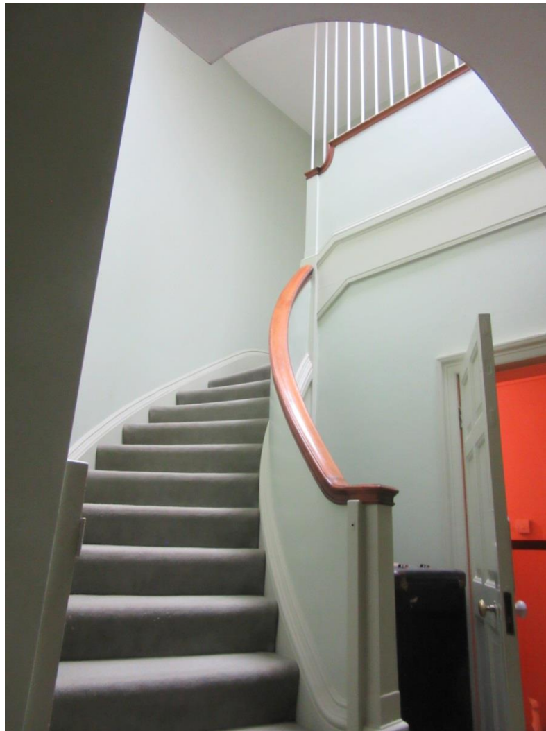
Figure 28: The stairs to the second floor lit by a rooflight – the balusters may be concealed within later boarding.
