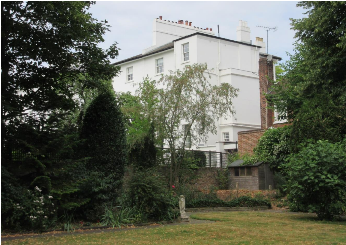
Figure 5: The rear garden and rear elevation of the subject site contributes to the suburban settings of the Grade II listed Nos. 34-37 Queen's Grove.
