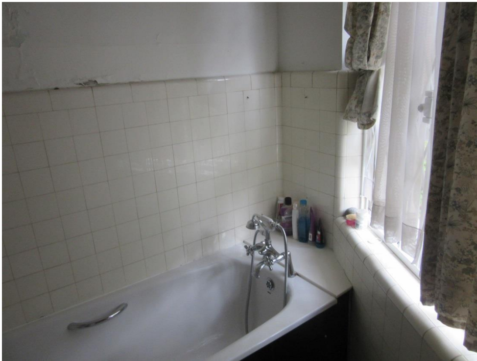
Figure 27: The One of the first-floor bathrooms showing original tiling.
