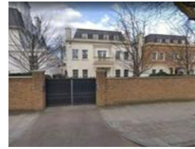
40 Avenue Road ● Full demolition with double basement
