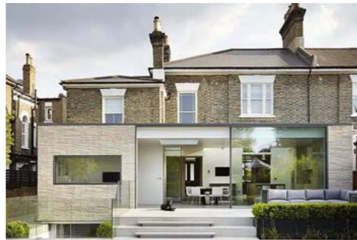
White Lodge Putney - extension subservient to host, light coloured brick relates to existing, minimal glazing
