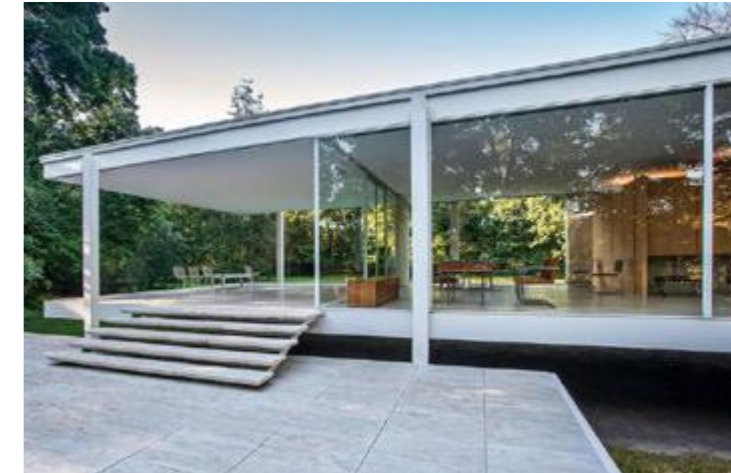
Farnsworth House - light and minimal, simple glazing, fine columns and projecting horizontals
