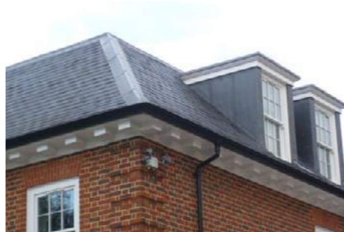
15 Acacia Road - prominent slate roof, dormer windows, ornate cornice
