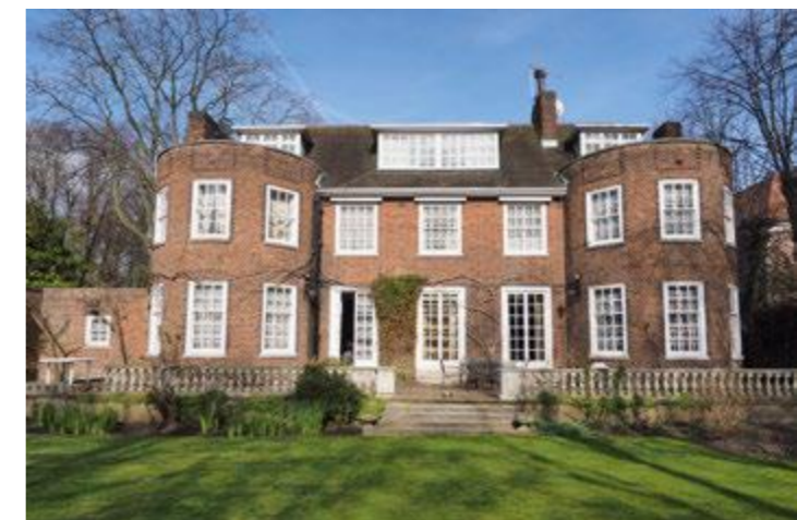
69 Avenue Road - Brick Recesses, symmetrical facade, hierarchy of windows, balanced proportions.
