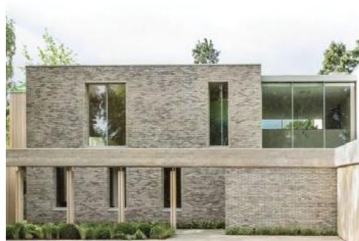
Berkshire II - contemporary use of brick, minimal window openings, horizontal layering
