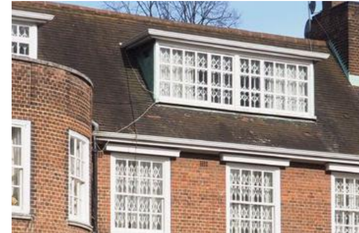
69 Avenue Road - prominent slate roof, dormer window recesses, paned windows
