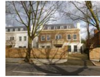
38 Avenue Road ● Full demolition with double basement
