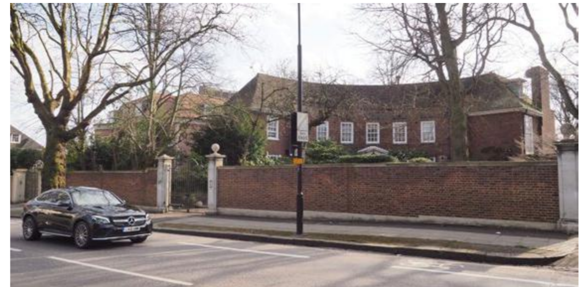
View 1 - Avenue Road Frontage
