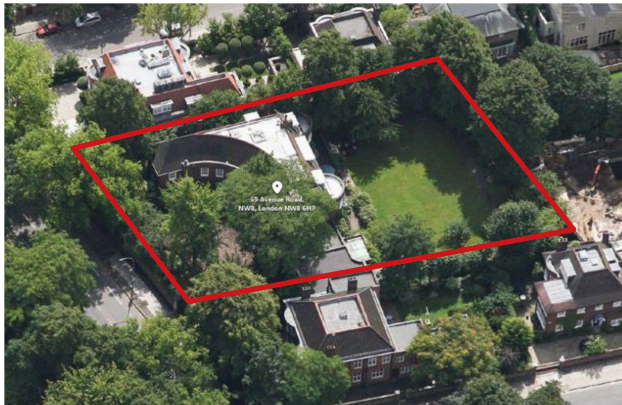
2.2.3 View North West
