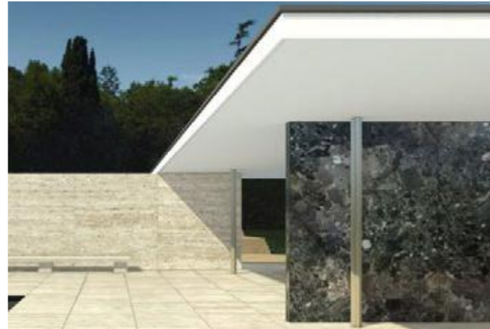
Barcelona Pavilion - lightweight structure, fine columns, floating roof, thin roof edge flat, overhangs
