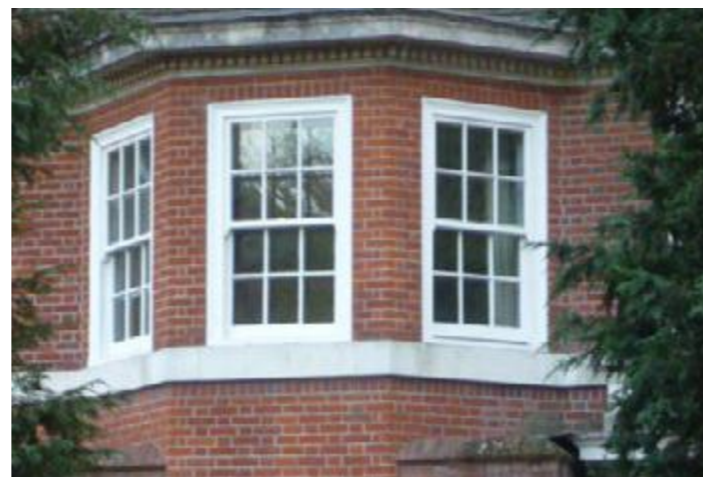
43 Avenue Road - stone banding, brick lintels, symmetrical hexagonal bays, red brick
