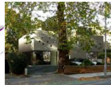
77 Avenue Road ● Full demolition with basement
