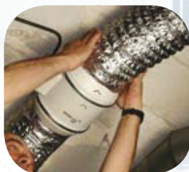
Connect the ducts
