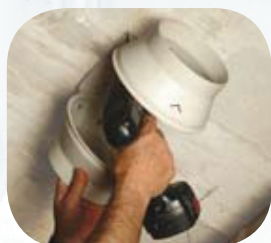
Fix the support bracket
