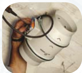
Carry out the wiring connections
