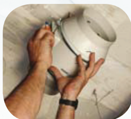
Place the impeller and motor assembly
