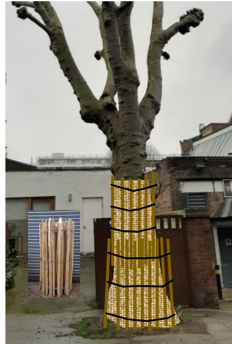
Fig 2. Above showing installation of chestnut fencing over hessian wrap.
