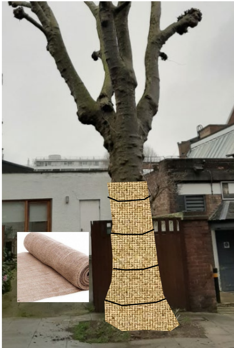
Fig 1. above showing installation of hessian wrap.
