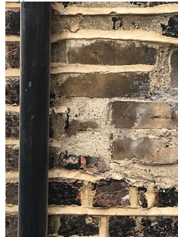
Figure 19 : Poor quality infill work
