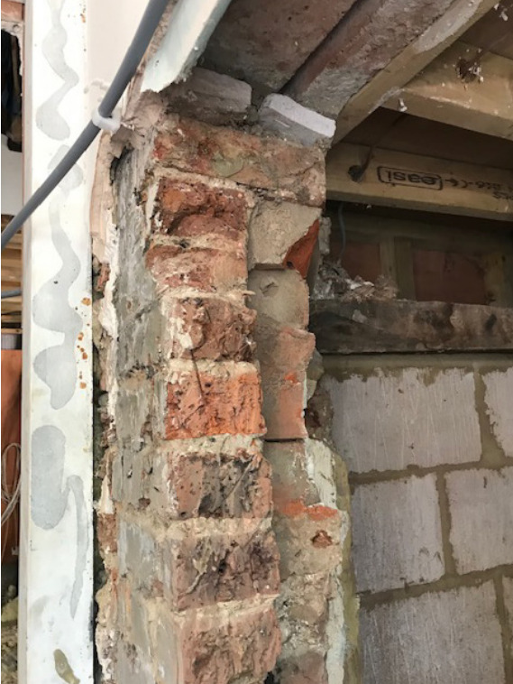
Figure 26 : Steel, original masonry and blockwork
