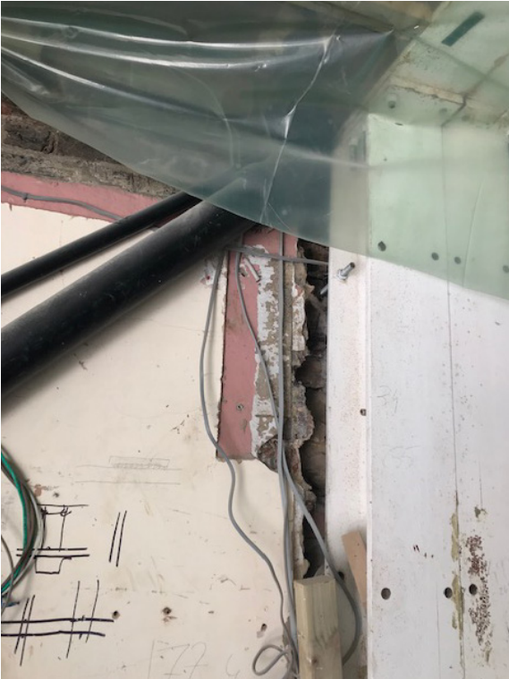
Figure 24 : Steel columns inserted into closet wing wall
