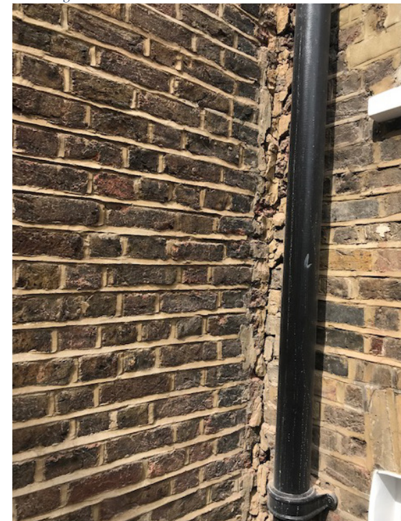
Figure 20 : Exposed open joint between the closet wing and the main house.
