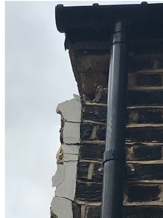
Figure 17 : Detailed photograph of the poor corner brickwork + plastic downpipe.
