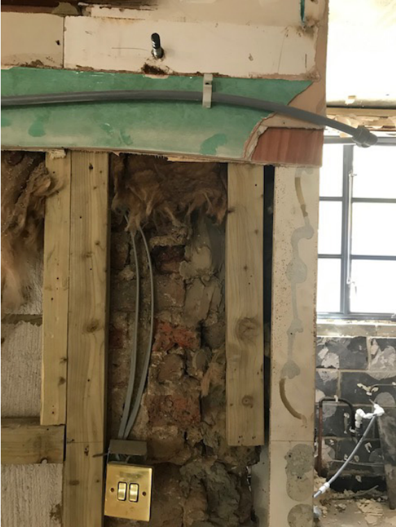
Figure 23 : Old masonry patched and altered
