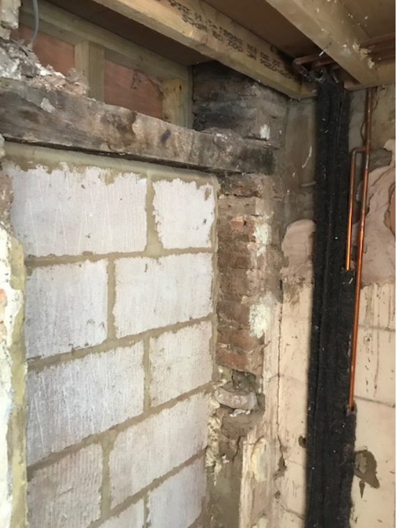
Figure 27: Blockwork wall infill
