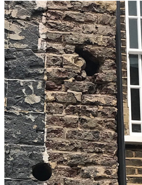
Figure 13 : Detailed photographs of the holes in the existing brickwork
