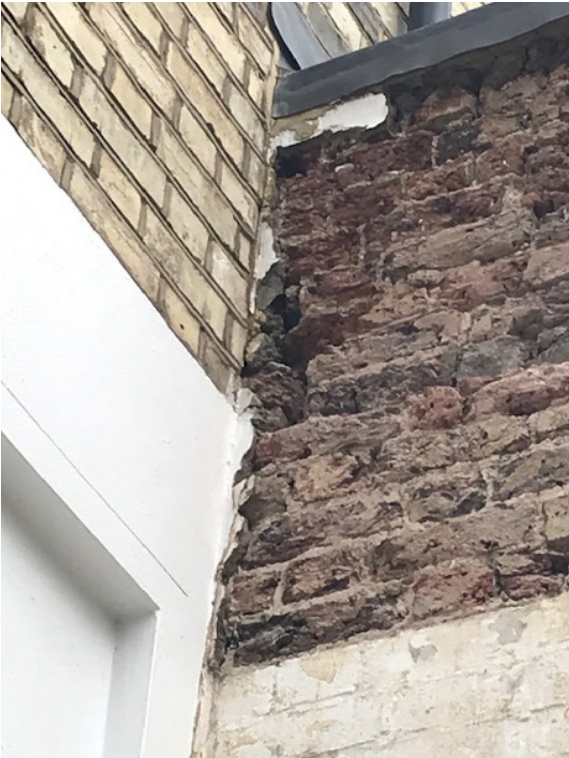
Figure 9 : View of the eroded brickwork on the corner of the closet wing
