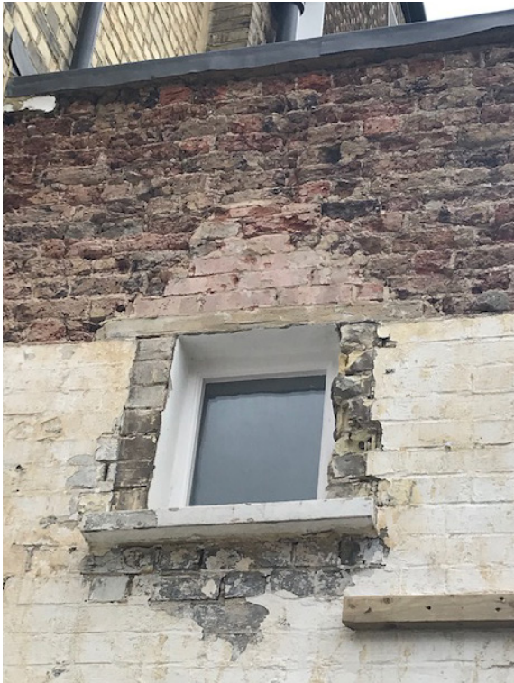
Figure 10 : View of the upper window and patched brickwork
