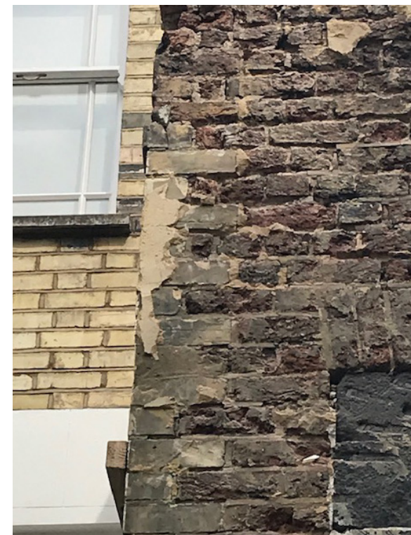
Figure 15 : Detailed photograph of the the poor corner brickwork
