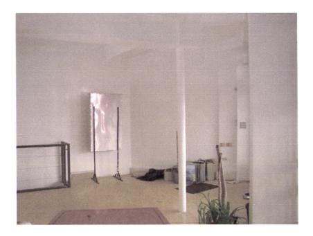
Photograph No.14 — Showing the two party walls to the adjacent Units that are proposed to be demolished to allow access through. Where both walls abutt a supporting pillar will remain.
