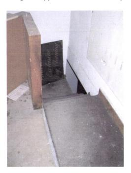
Photograph No. 4 – Shows the top of the stairs leading down to the basement of Unit 6. The stairs are proposed to be removed and the floor boarded over.
