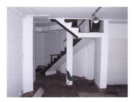
Photograph No.7 – Showing the stairs construction within Unit 6 basement.
