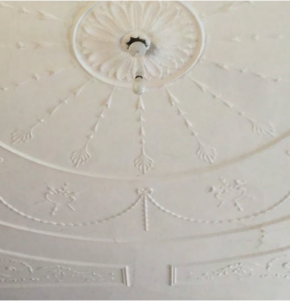
Existing decorative ceiling plasterwork of swag and drop detail with central leaf plaster rose
