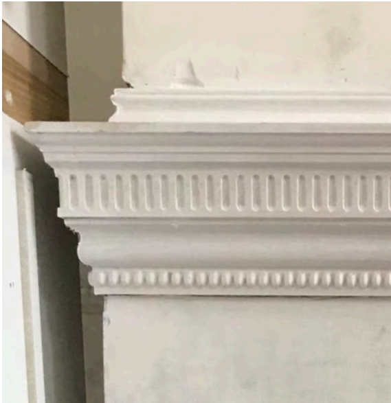
Existing dado rail with fluted & beaded panel moulds
