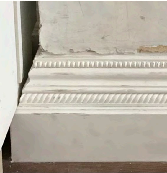
Existing skirting with double rope panel moulds
