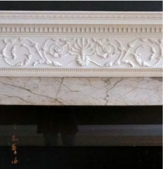
Existing decorative plasterwork of swag and drop detail to centre of Fireplace surround
