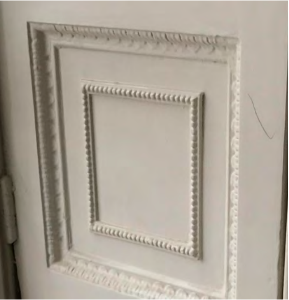
Existing window shutter with leaf & bead panel mouldings
