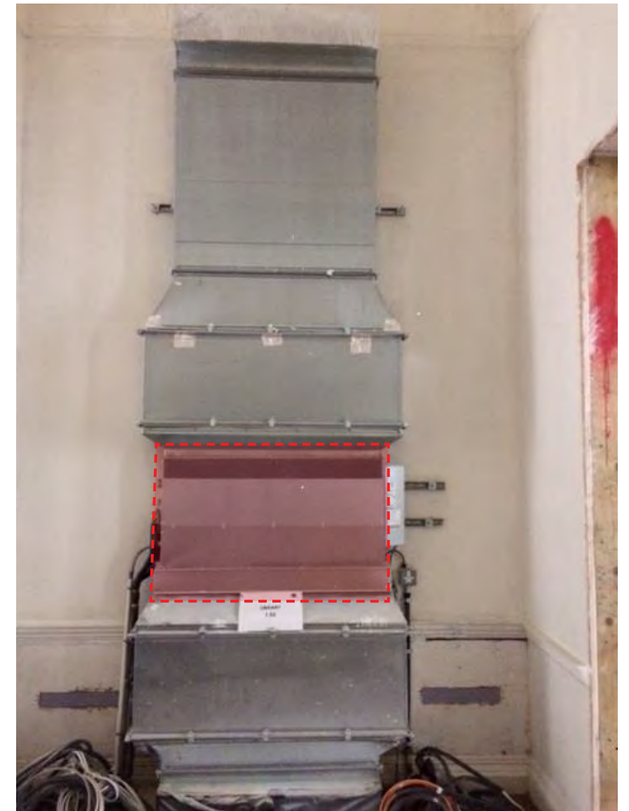
Comfort cooling unit with attenuation in first floor library. Red hatch represents actual unit.
