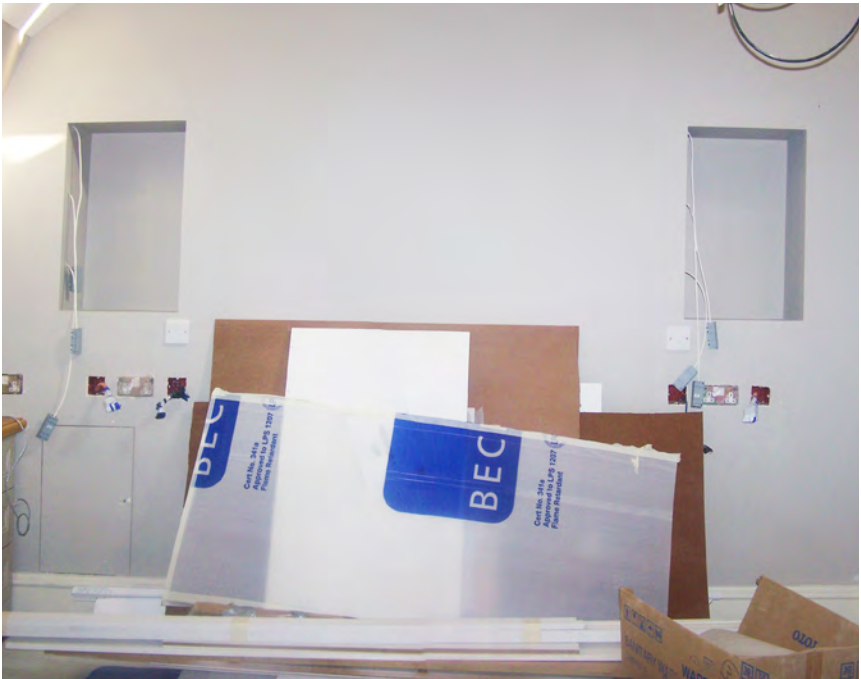
3.07. Wall lining with niches in front of chimney breast to be removed.
