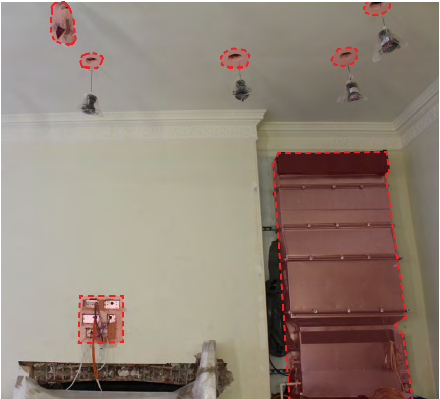
Image of Dining Room Fireplace elevation illustrating fan coil unit to be reduced, ceiling penetrations to be repaired and socket outlets above fireplace to be removed.
