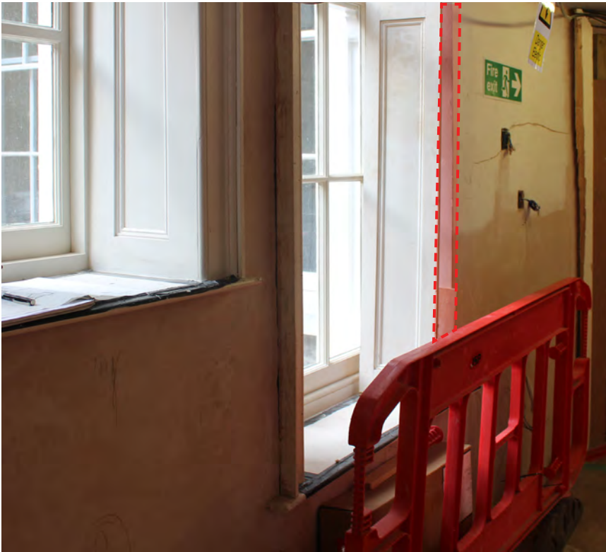
0.01. Missing window architrave to be reinstated
