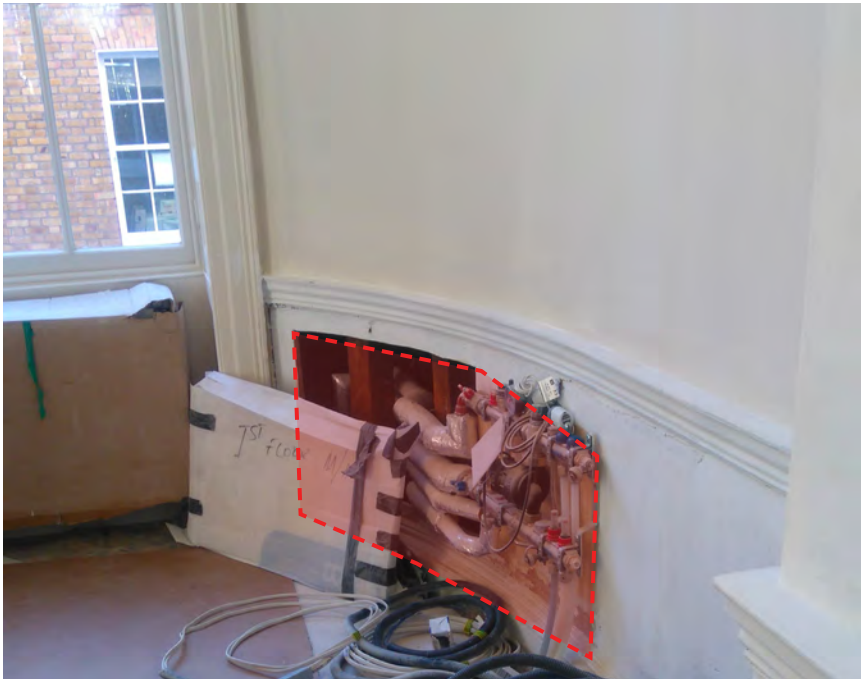
1.03. Underfloor heating manifold to be relocated to concealed location in rear bay lift hall. Timber panel to be reinstated.
