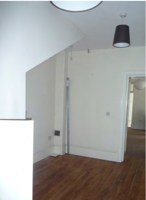
Image taken within the lower ground stair hall prior to the 2014 application. Note the modern finishes throughout, low plasterboard ceilings and the uncharacteristic open space beneath the boarded up cantilevered stone stair intended to connect the lower ground and ground floor levels.
