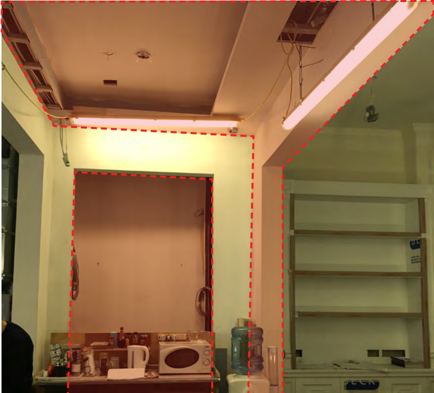
0.06 Image of central area of Living Room illustrating enlarged openings, modern nib partitions and modern suspended ceiling area all to be carefully removed and reinstated.
