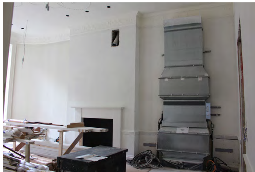
Section of masonry wall removed and excessive scale of fan coil unit.
