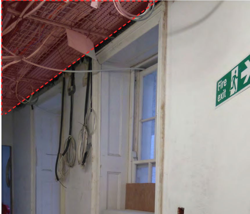
B.01. Ceiling to be reinstated above window architrave.
