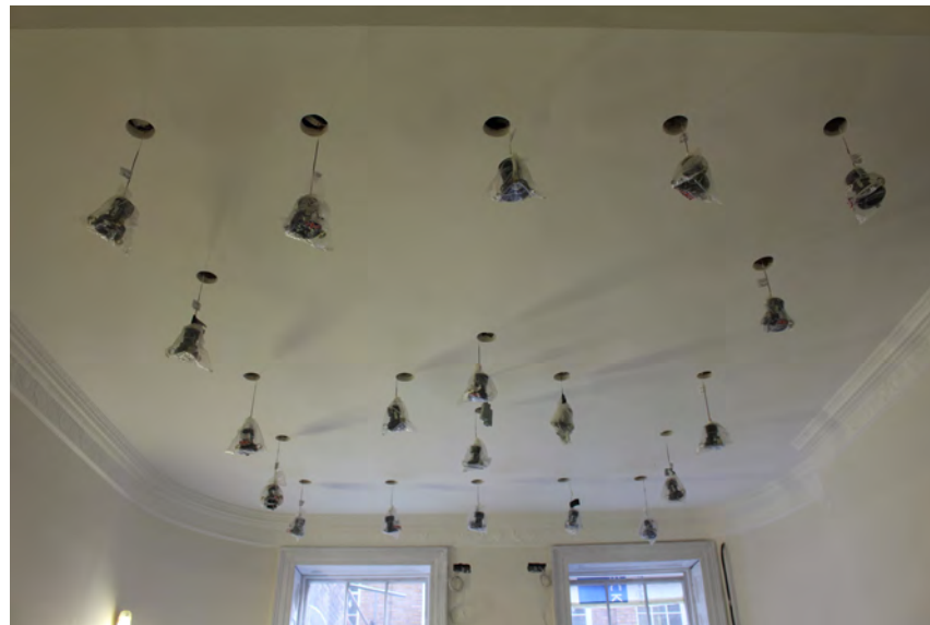
Holes created in lath and plaster ceiling at ground floor level
