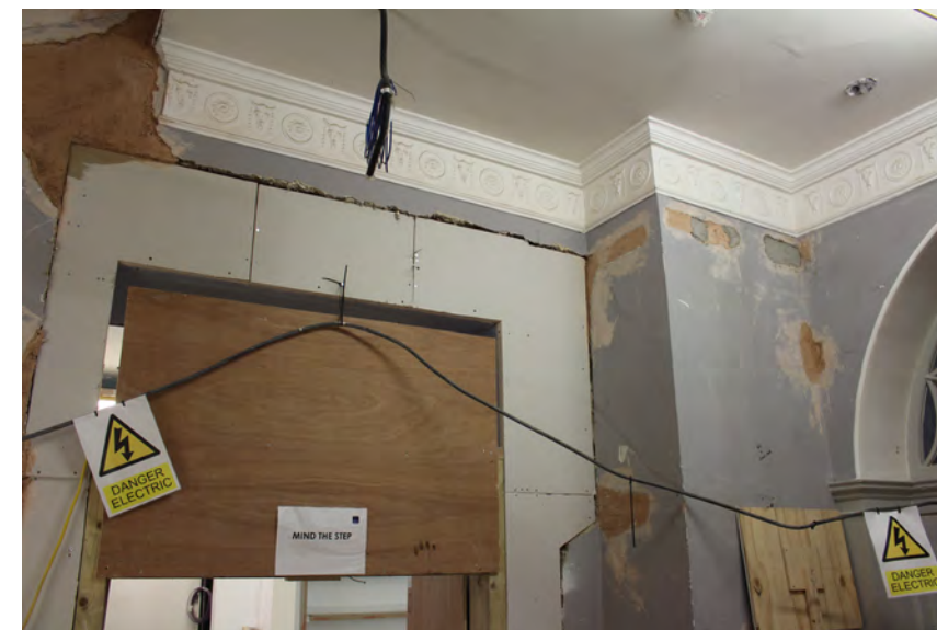
Existing door opening enlarged. Making good of opening in modern materials..
