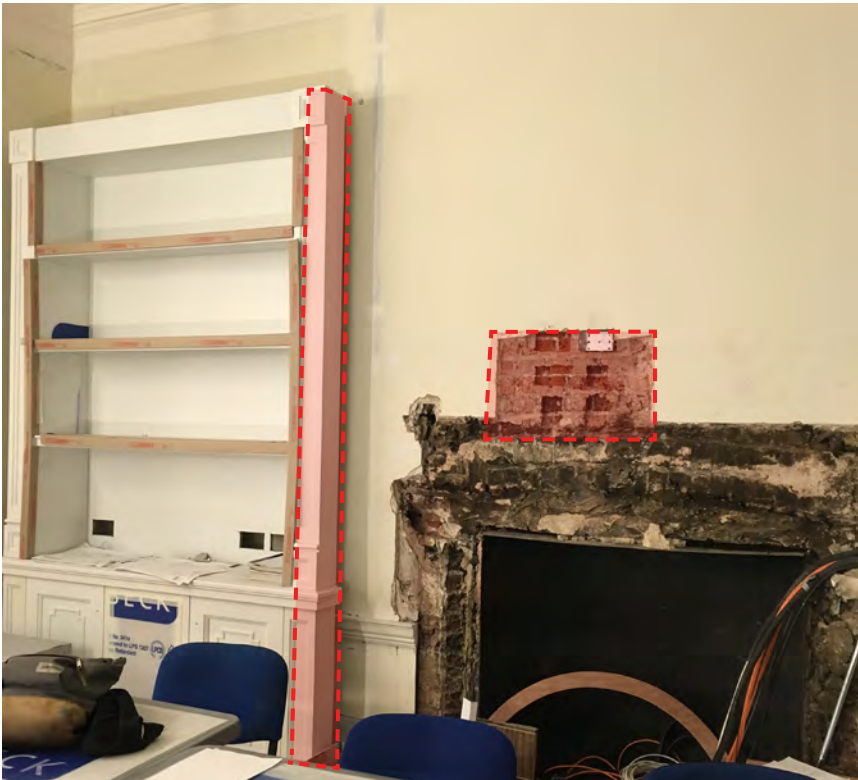
0.06 Image of Living Room Fireplace elevation illustrating socket outlets above fireplace to be removed and example of current furniture design overlapping chimney breast feature.
