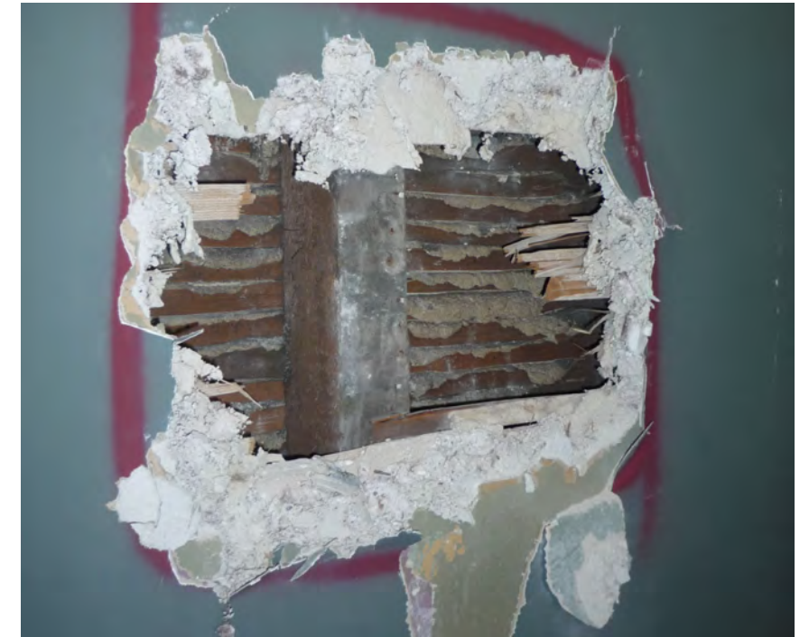
Image of an intrusive investigation in the rear room at the ground floor taken prior to the 2015 application revealing lath and plaster construction on timber stud partition.
