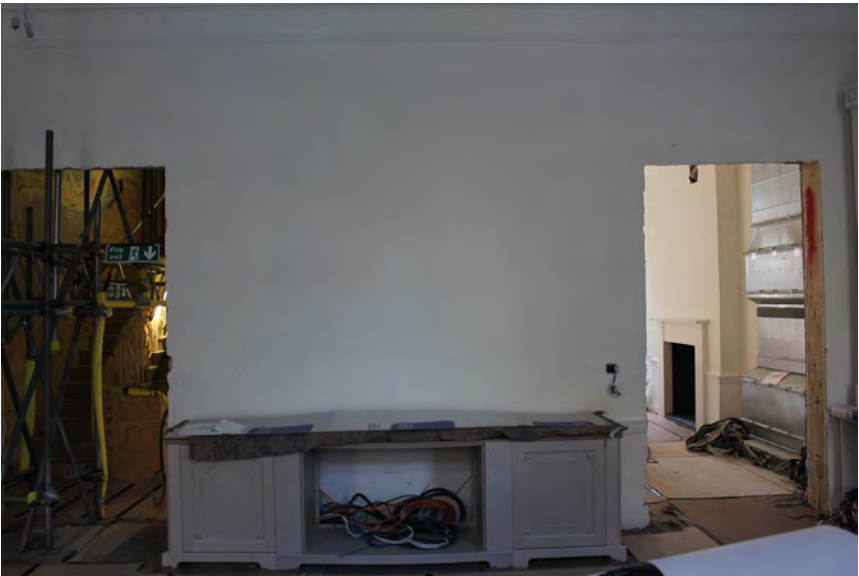
Enlargement and relocation of existing door openings at first floor level
