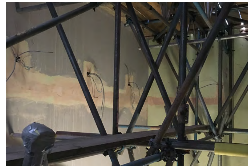
Modern plaster repairs throughout stair well to be replaced with lime plaster to match existing.
