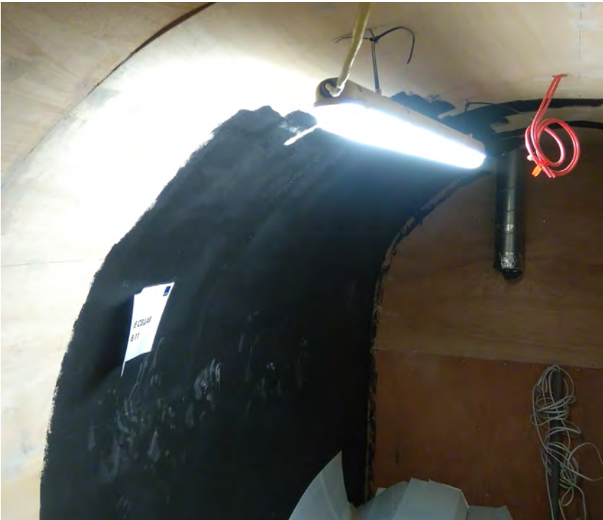
B.11. Ply lining over poor quality brickwork to be painted black and new timber battens installed.
