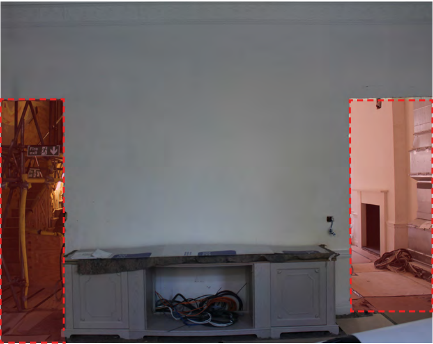
1.04. Relocated and enlarged openings to be reinstated to match original locations and scale
