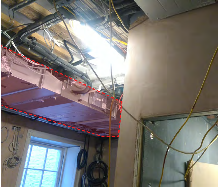
B.08. High level fan coil unit to be reduced and relocated. Ceiling to be reinstated above window architrave.
