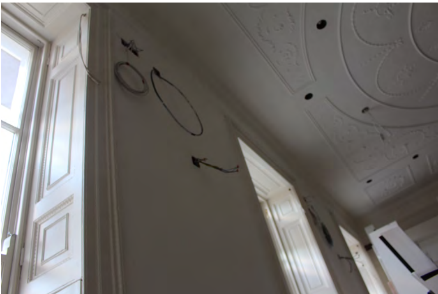
High level socket outlet locations adjacent to windows at first floor. Holes in decorative ceiling
