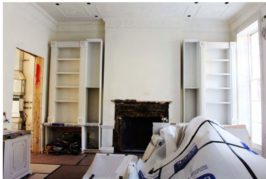
Existing fireplace removed from wall at first floor reception room. Fireplace in safe storage.
