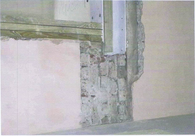
PHOTO OF RIGHT SIDE (FROM STAIRS)
