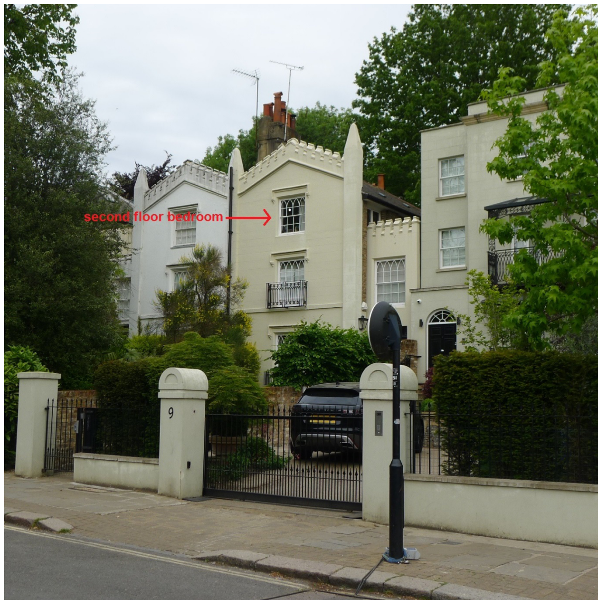
Front elevation from Downshire Hill
