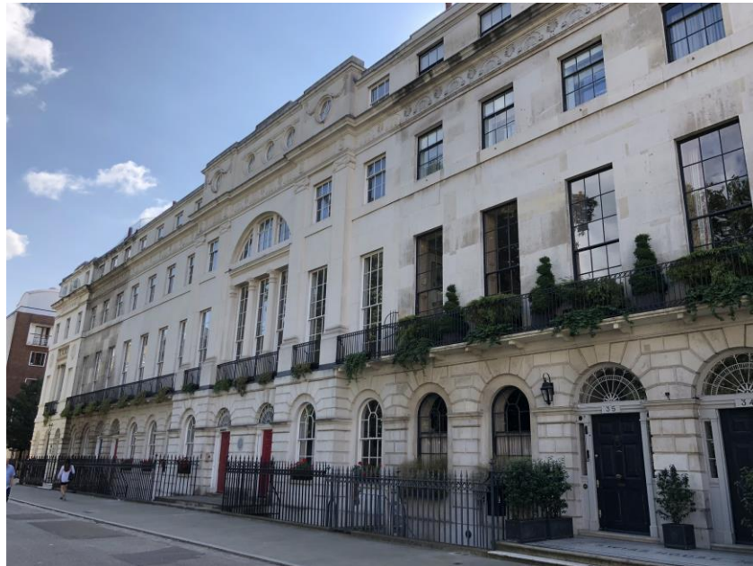
Boston House from Fitzroy Square (view northwest to southeast)
